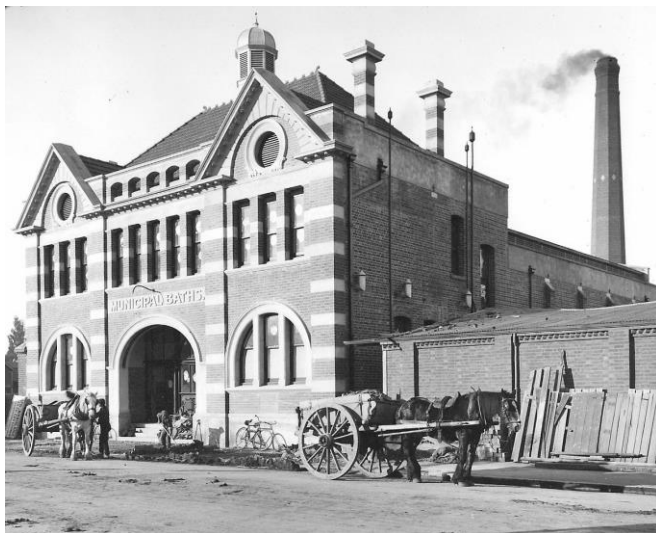
The Tepid Baths building on Manchester Street. Behind is the chimney of the rubbish destructore which heated the water for the pool.
