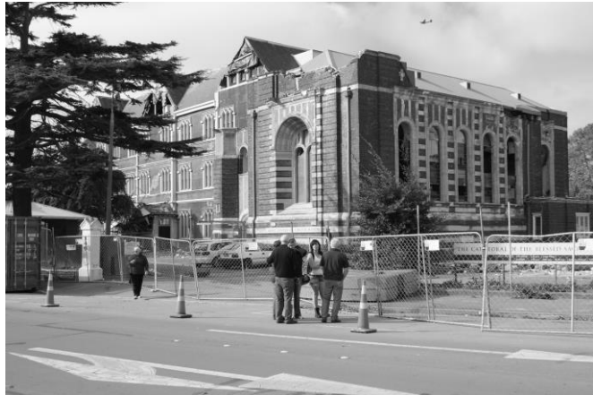
A Former convent and its chapel beside the Catholic Cathedral had become a thriving Music Centre, with the chapel used for performances, before earthquake damage, evident in this photo, resulted in both buildings being demolished.
