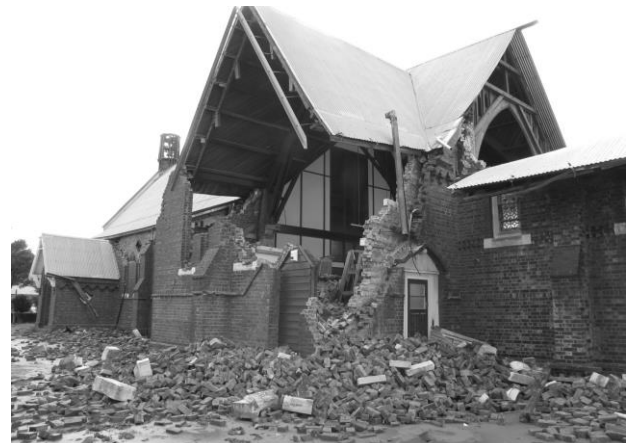
The Church of the Good Shepherd, Phillipstown, was also badly damaged in the 22 February 2011 earthquake and subsequently demolished.
