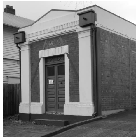
Typical of the many small substations throughout the city is this one on Worcester Boulevard, in the central city.
