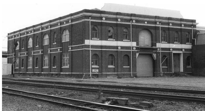
Wool and grain stores as well as factories were located in the 'railway corridor'. This early woolstore designed by W.B. Armson survived until the earthquakes.
