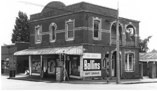
The most imposing architectural of Christchurch's 'corner shop' buildings was well-known as the Piko wholefoods store. It was demolished after the earthquakes.
