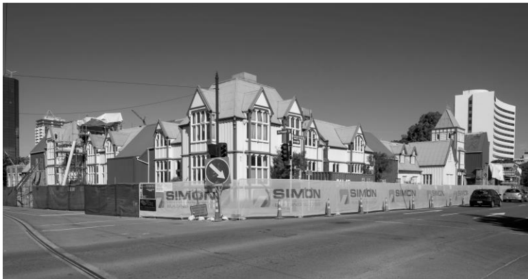
Although the Stone Chamber collapsed in the 22 February 2011 earthquake, the wooden portions of the Provincial Government Buildings survived the earthquakes with relatively little damage, caused mostly by the collapse of masonry walls and chimneys.
