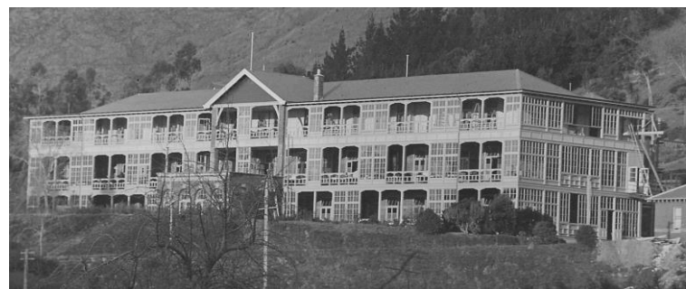
The buildings of the Sanatorium were landmarks on their spur of the Cashmere Hills. They have all been demolished.
