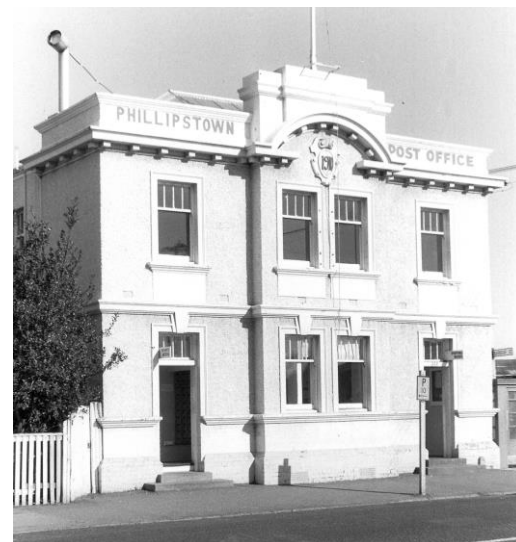
The Phillipstown post office on Ferry Road was demolished many years before the earthquakes.
