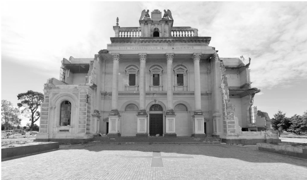
The city's two cathedrals, Anglican (top) and Roman Catholic (lower), were among the most conspicuous casualties of the Christchurch earthquakes. The futures of both buildings are unclear in the middle of 2013.
