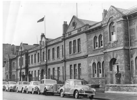
The old police station on the site which the Police occupied from 1874 until the earthquakes. The building was made up of two early stone wings linked by a later brick block.
