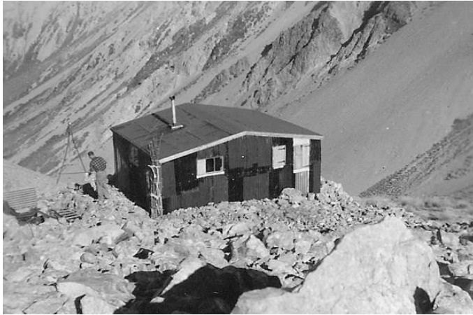
The tow hut built by volunteer labour in the early 1950s at one of the club ski fields in the Craieburn Range.
