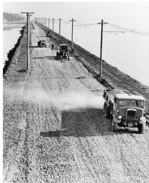
As use of private cars increased, the city's roads were improved to cater to the increased traffic. In the 1930s a road was built alongside the older tram track to form the McCormack's Bay causeway on the way to Sumner.
