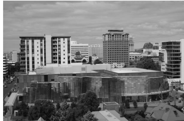
The Clarendon Towers, centre right, and the apartment building, centre left, have been demolished since the earthquakes.
