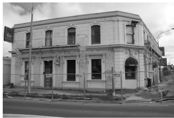
Damaged in the earthquakes, the Lancaster Park hotel was subsequently demolished. It was the last of the hotels designed by J.C. Maddison
