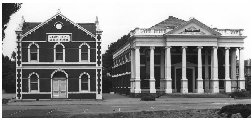
The Oxford Terrace Baptist Church hall, left, was demolished many years before the church itself became a casualty of the earthquakes.
