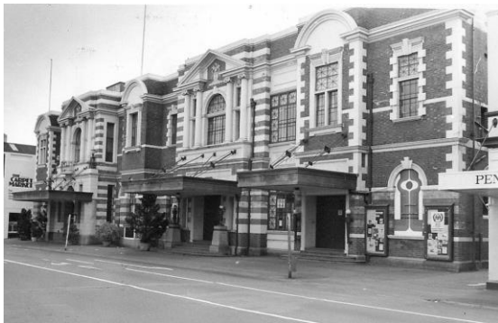
The Council's home from the 1920s until 1980 on Manchester Street has been demolished.
