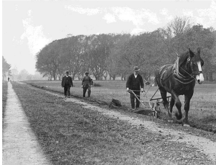
By around 1915, when work was still proceeding on developing Hagley Park, the earlier plantings of trees, background, were already mature.
