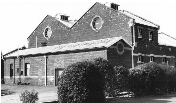
When the city's high-pressure water system was built in the early 20th century, a large brick pumphouse was constructed in Beckenham. The building was demolished in the 1980s.
