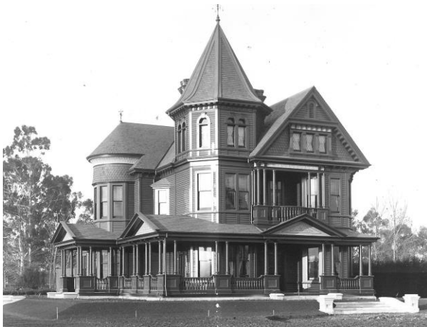
Fitzroy, the grand Merivale home of a city industrialist, became the headquarters of the Nurse Maude Association.
