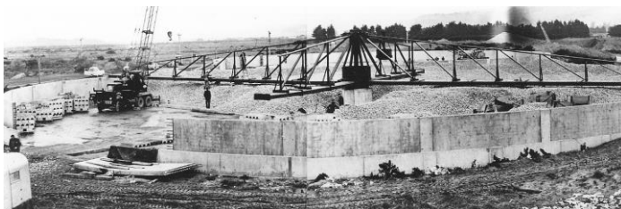
Top: When Christchurch's first sewerage system was built in the 1880s, a sewage farm was built at Bromley. Bottom: When a treatment station was built on the site of the farm in the 1950s, trickling filters were among the improvements.
