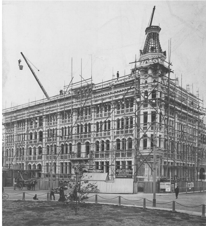
The Press building on Cathedral Square was one of the city's notable commercial buildings, until it was demolished after the earthquakes. It is seen here under construction.
