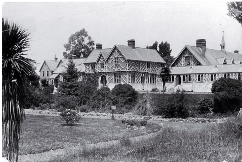
The early buildings of the Christchurch Hospital seen from what are now the Botanic Gardens.
