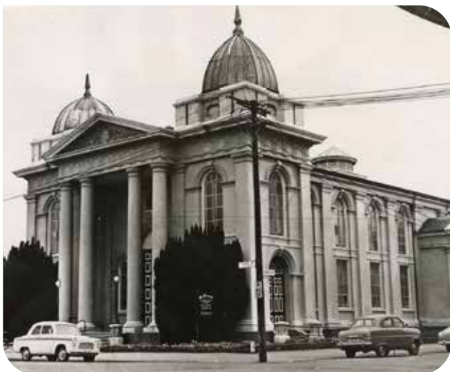
St Paul's Presbyterian Church on the corner of Cashel and Madras streets.
