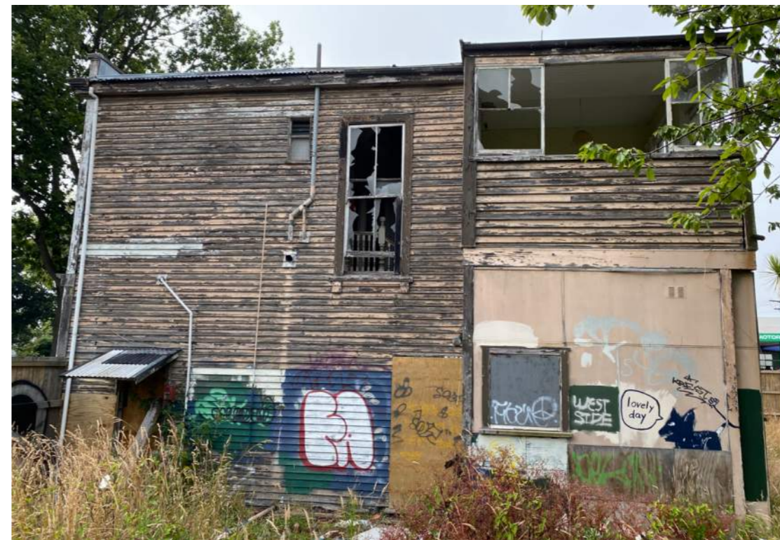
4 Photo 4: North Elevation
