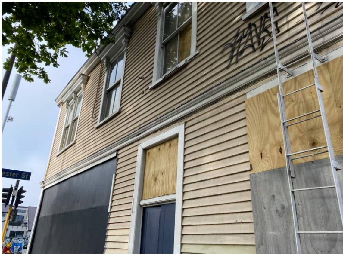
1 Photo 1: East Elevation
