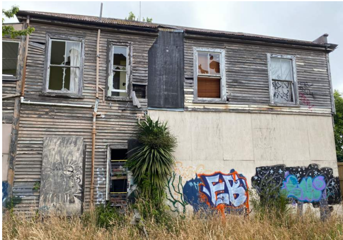
3 Photo 3: West Elevation
