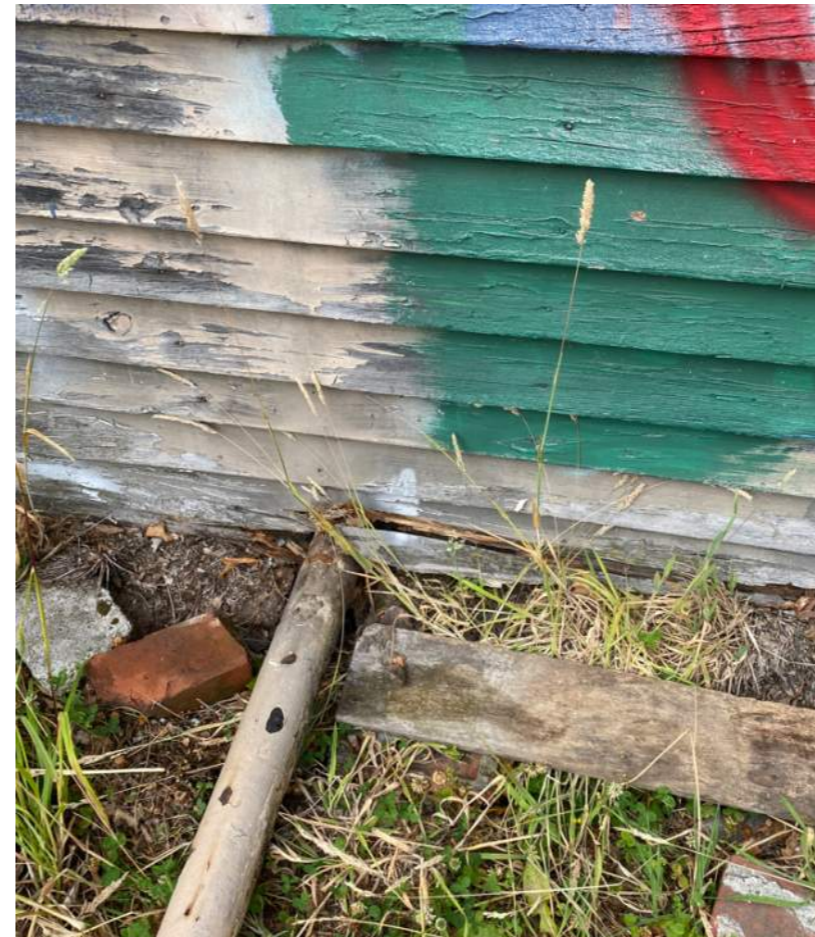
12 Photo 12: External weatherboard, foundations and drainage
