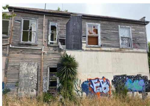
Image 7: Existing cladding on elevation
