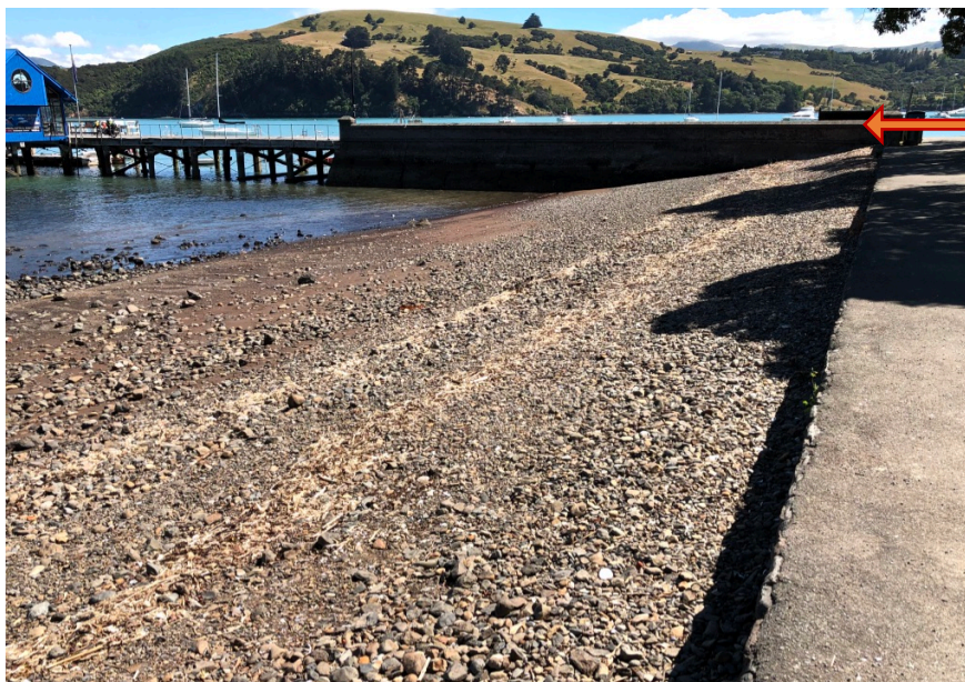
South side of the Akaroa Wharf next to the Britomart Reserve, 2022
