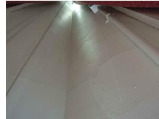
2.32 | CRAZED CRACKS UP WHOLE HEIGHT OF COLUMN AT GRID 21 A-520
