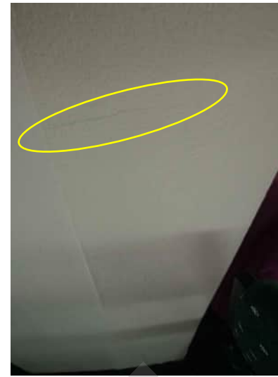
2.27 | MULTIPLE HAIRLINE HORIZONTAL CRACKS DOWN SIDE OF COLUMN ON GRID 16 (GRID 17 SIMILAR) A-520
