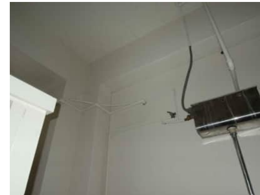
0.55 | VIEW OF BEAM COLUMN JOINT AT GRID 13 A-500
