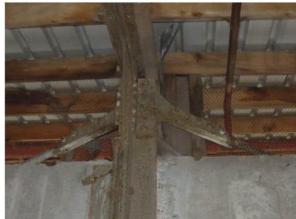
Bracing connection to level 4 shear wall
