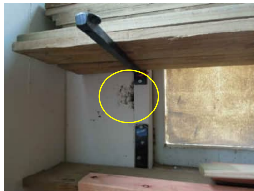
0.10 A-500 | POORLY COMPACTED CONCRETE AROUND WINDOW FRAME AT MID-HEIGHT OF GRID D COLUMN
