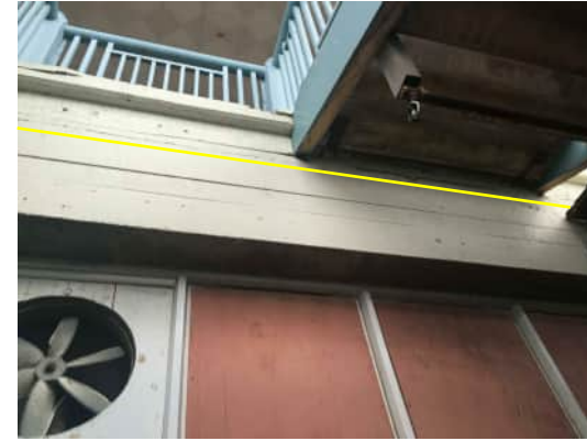
EN8 A-552 SIGNIFICANT HORIZONTAL CRACK ALONG TOP OF WALL AROUND 10MM WIDE, AT LOCATION WHERE STAIRS TO STANDS HAVE BEEN CAST INTO THE WALL
