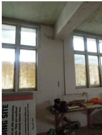
0.44 TYPICAL BEAM COLUMN JOINT ON GRID D A-500
