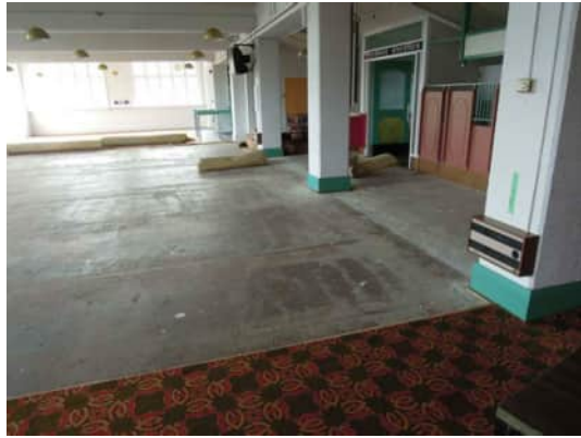
1.1 | VIEW OF EXPOSED SLAB A-510
