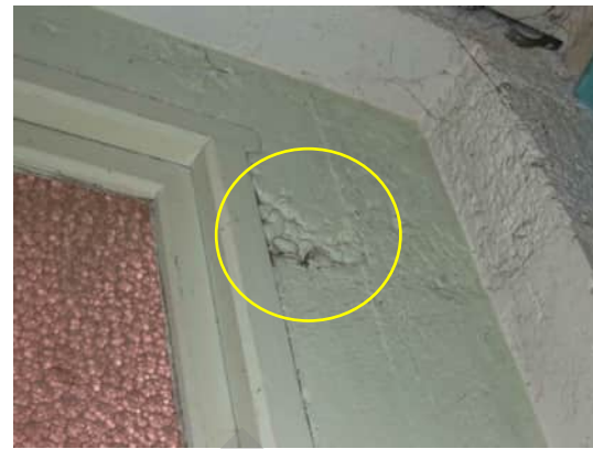
0.26 A-500 | TYPICAL POORLY COMPACTED CONCRETE WITH EXPOSED AGGREGATE NEAR TOP OF COLUMNS
