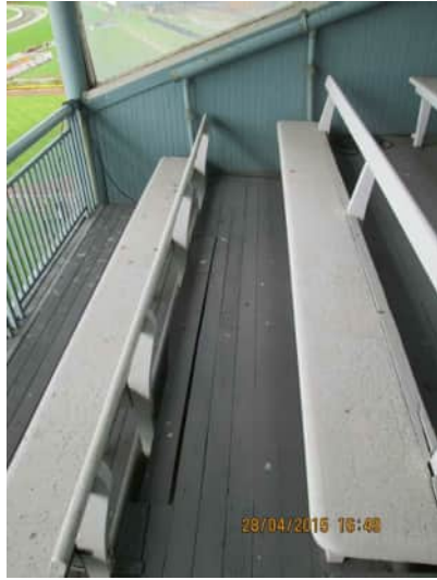
4.13 A-540 | CONDITION OF TIMBER DECKING ON THE UPPER STAND
