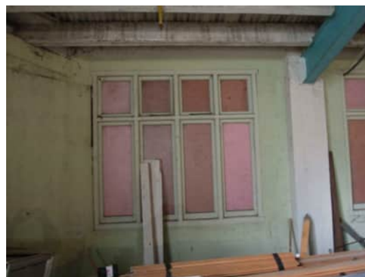
0.21 VIEW OF TYPICAL GRID A BAY A-500
