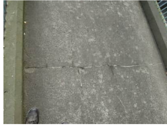
R2 A-810 TYPICAL CONSTRUCTION JOINT ON TOP SIDE OF RAMP
