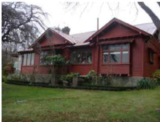
Red House viewed from the west. The area of wall between the two gables was formerly an entry. The steps are still in place
