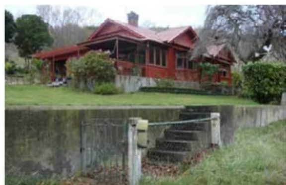
Steps and retaining wall below the house
