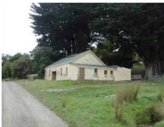
The barracks in context. Note macrocarpa trees behind building
