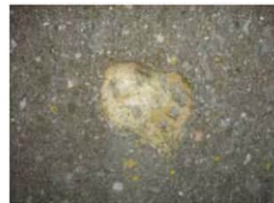
Mortar patch to monument stone
