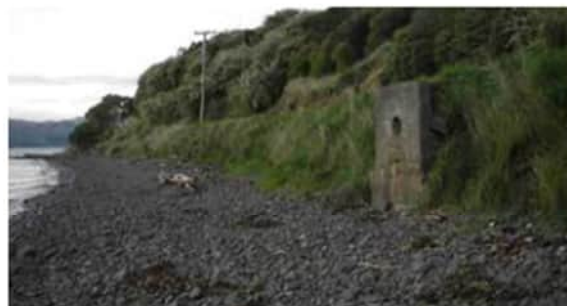
Concrete foundation for culvert (Mosley, May 2010)
