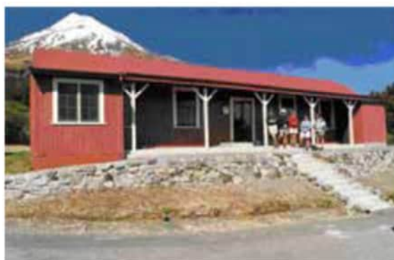
Surviving section of the old New Plymouth army barracks on Mt Taranaki, following restoration ( http://www.doc.govt.nz )
