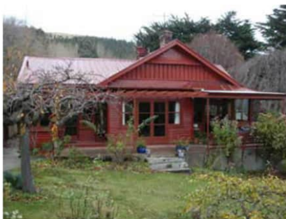
The house as viewed from the north. Various additions and alterations have been carried out.
