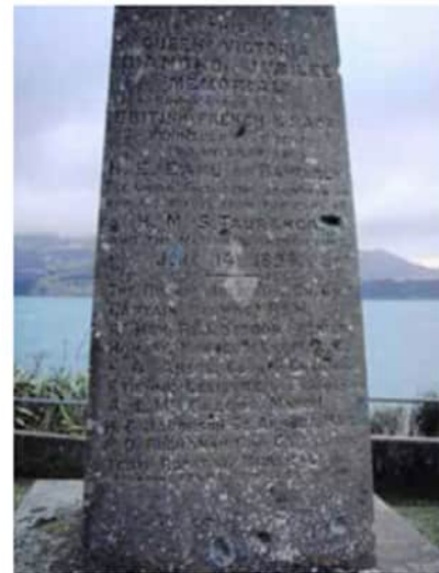
Pitting of stone. A substantive crack is also visible towards the right of the stone
