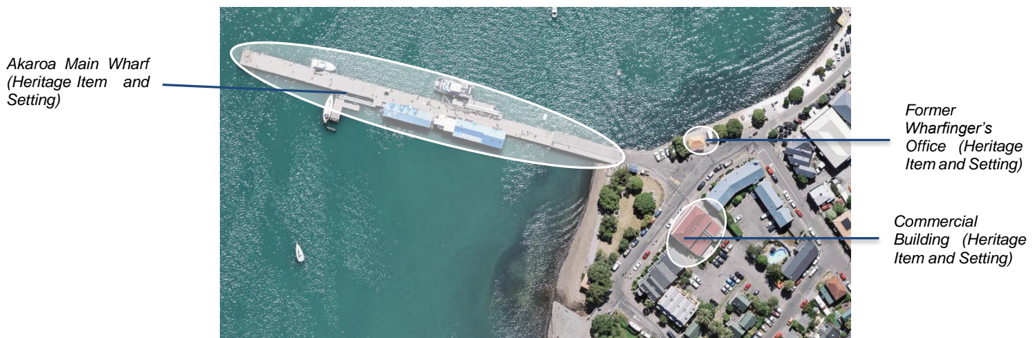
Figure 3: Aerial photo of the surrounding area to the Main Wharf in Akaroa.
