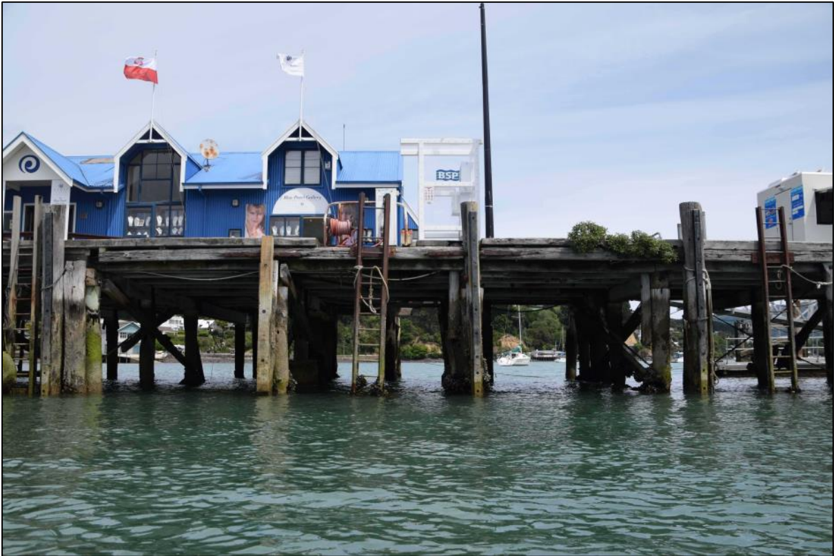
Photo 10 The end of the shed and the BSP fuel station. On the far right is a tethered caravan selling fresh fish. The outer piles here have had modern fenders added.
