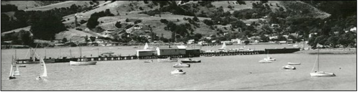
Figure 40. Detail of a 1971 photograph showing the south side of Akaroa Main Wharf (Archives New Zealand).
