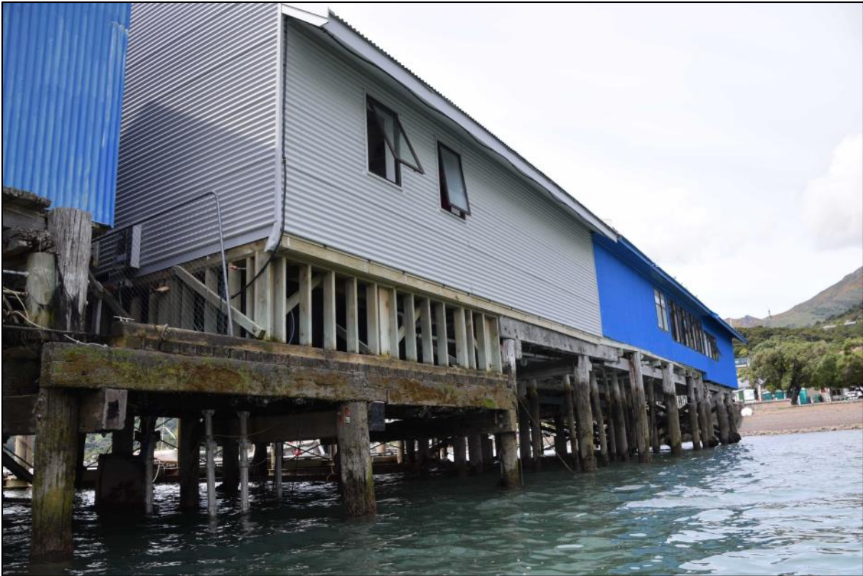
Photo 22 showing the lowered deck area (Photo 21) accessed by timber steps between the two sheds. Note the steel props under the lowered deck.
