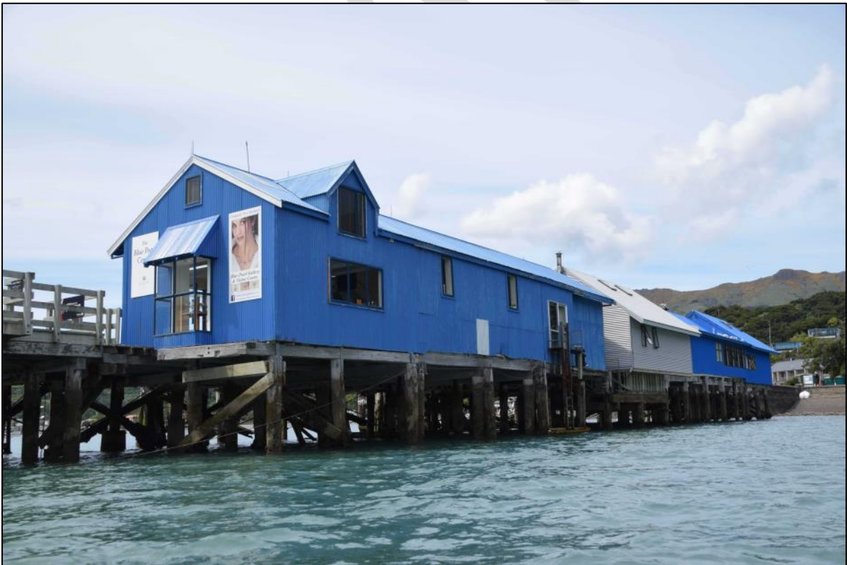
Photo 15 The line of modern sheds on the south side of the wharf running from the 6th bent from the abutment to the 21st and enveloping and extending the original sheds' footprint which ran from the 15th to 20th.
