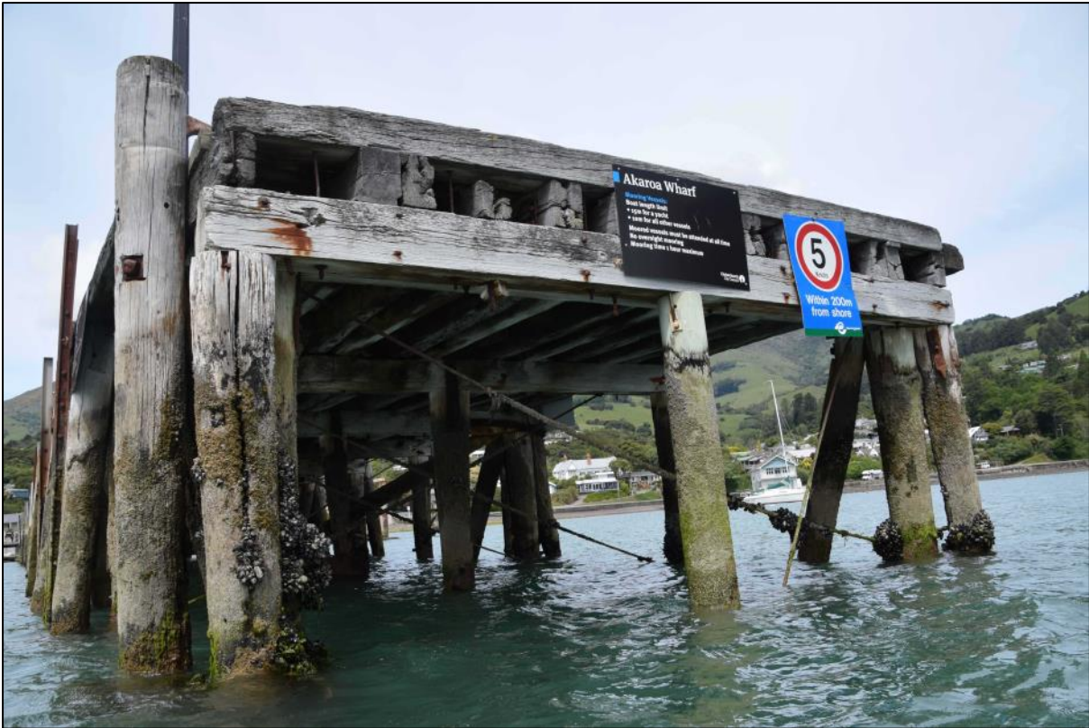
Photo 12 The outer/west end of the wharf clearly showing the original construction, although with some replacement tanalised piles. Along the top of the piles is the timber pile cap (beam). On top of that are the stringers and running parallel to the cap is the timber kerb with the timber decking behind it. On the far left and far right are fender piles and each corner has an inner bracing pile.
