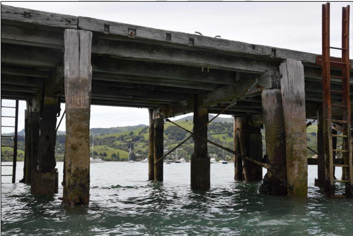
Photo 13 Here the original timber cross-braces to the bents have been replaced with modern steel bracing rods and a number of the piles have had repair 'jackets' encased around their lower sections.
