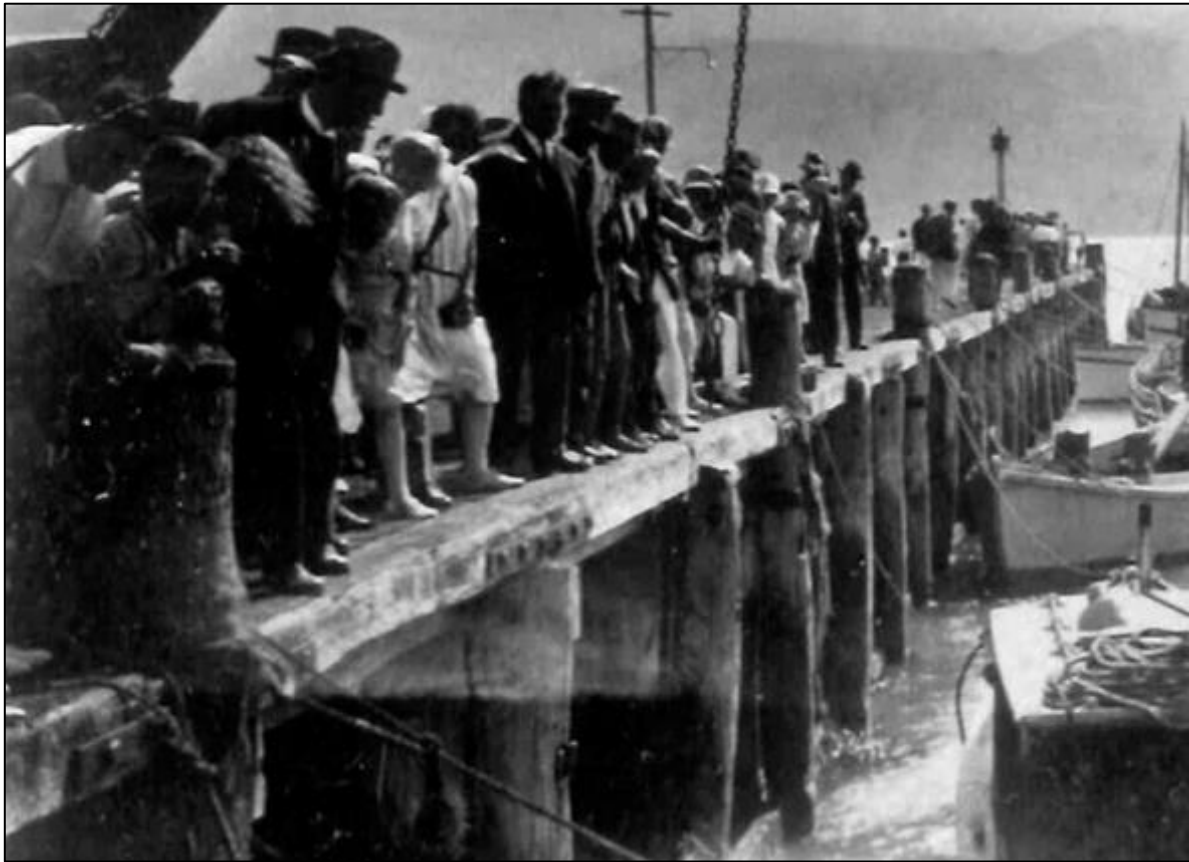
Figure 29. Detail of an undated early 20 th century image showing the iron slice straps on the side of the wharf (Canterbury University Archives).
