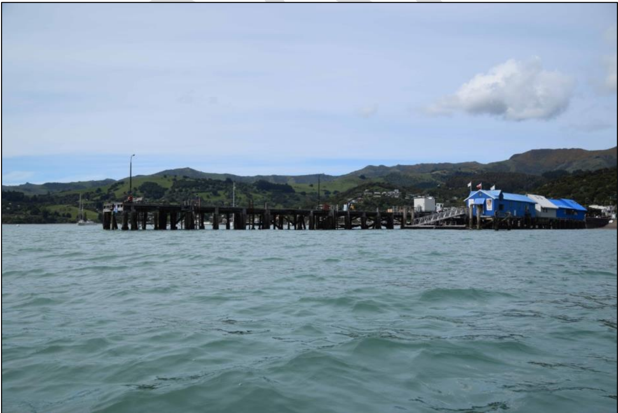
Figure 2. The south side of Akaroa Main Wharf (2018).
