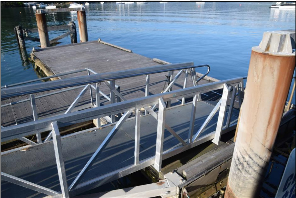
Photo 51 South floating pontoon.
