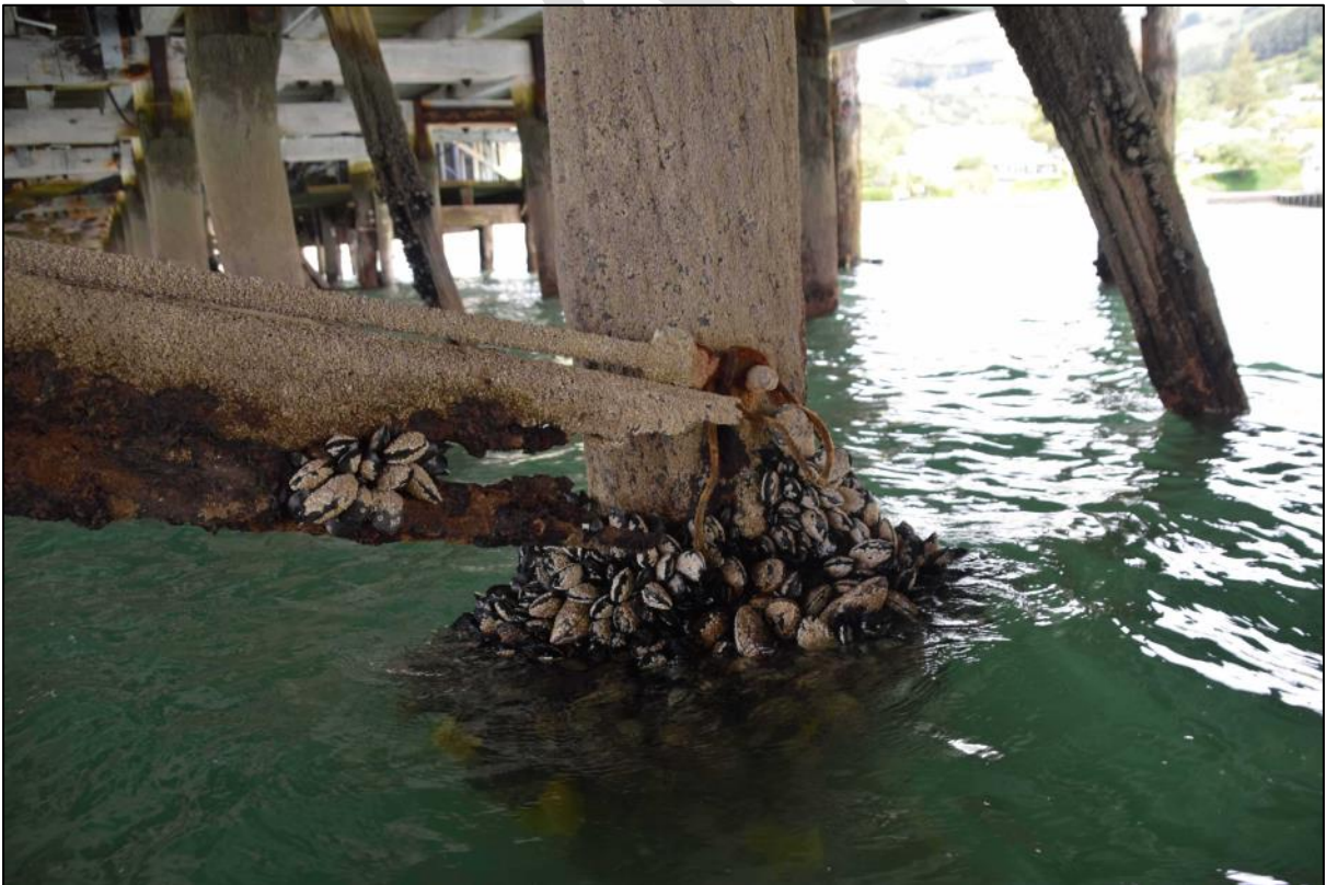
Photo 35 Broken/corroded steel brace.
