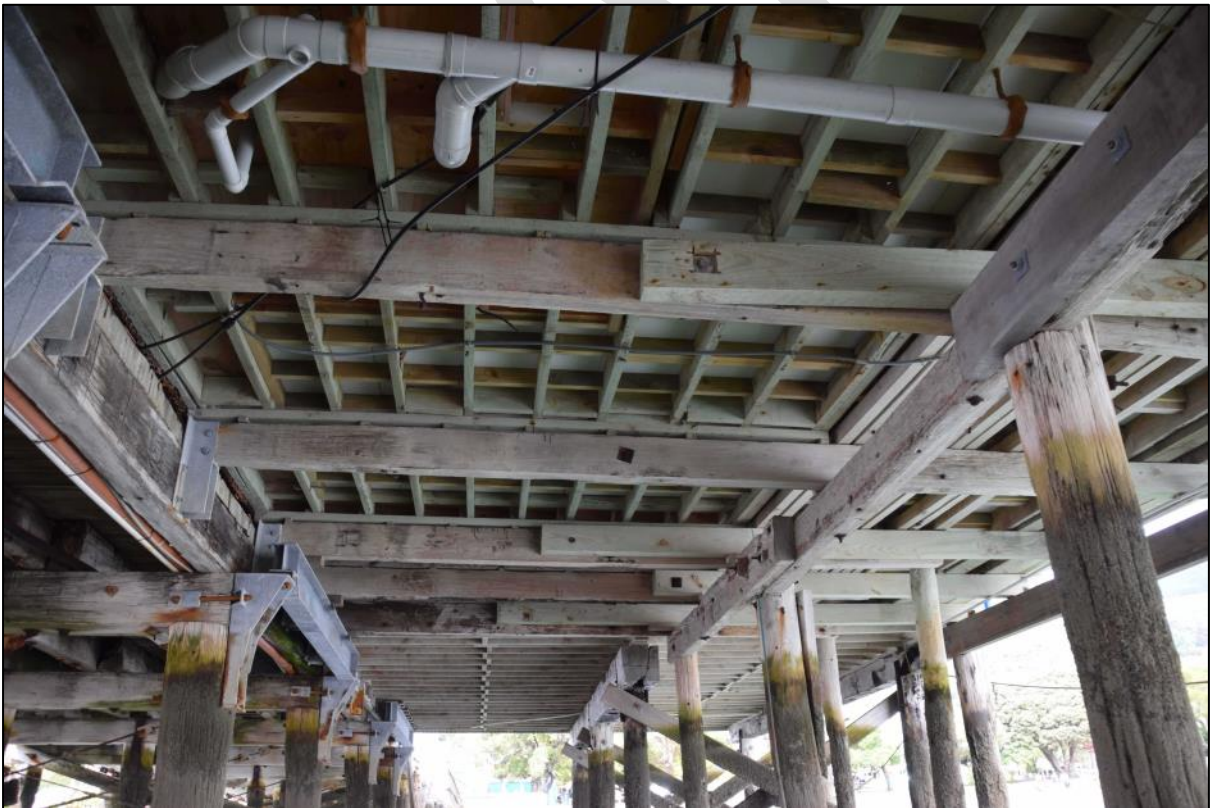
Photo 43 As Photo 42 (looking east), but showing in more detail two different periods of modern floor framing (foreground and distance).
