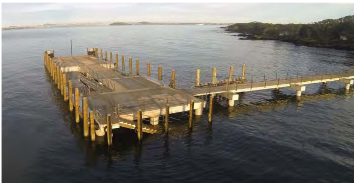
Figure 22: Rangitoto Island Wharf, Auckland. Example of reinforced concrete wharf
