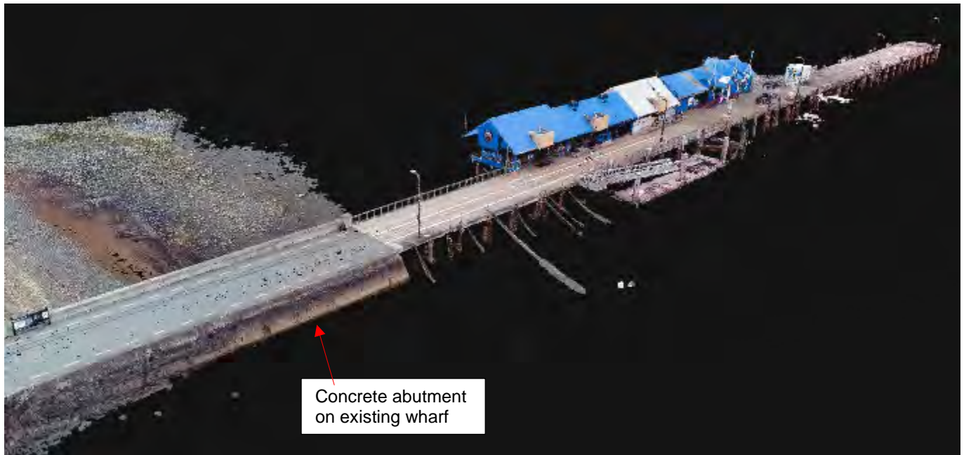
Figure 19: 3D scanner image of existing wharf, showing concrete abutment and hardwood wharf beyond
