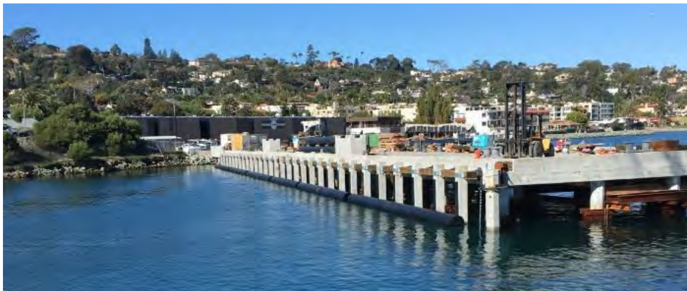
Figure 21: UCSD Nimitz Wharf. Example of reinforced concrete wharf
