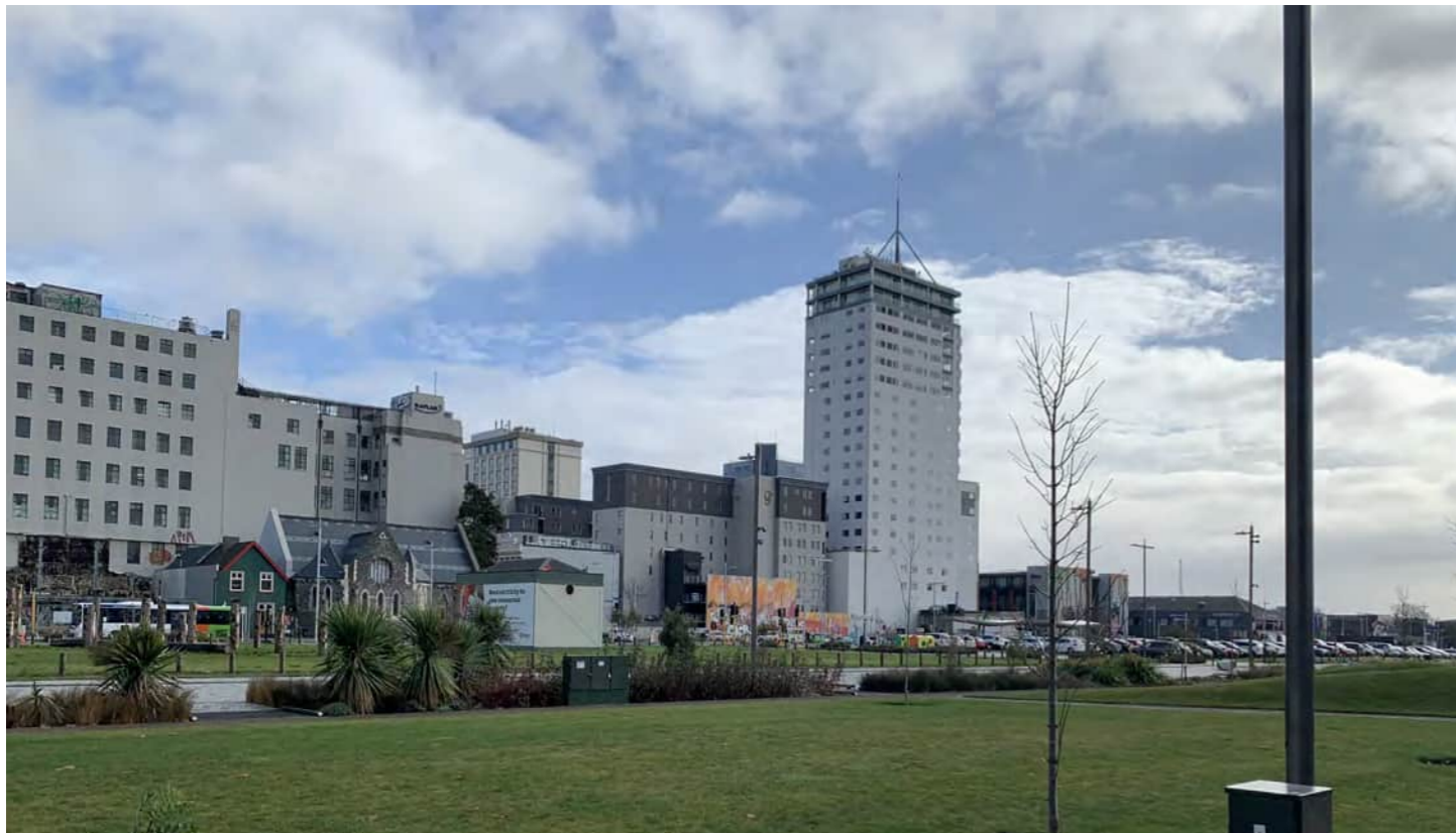
C View from adjacent greenspace of multi-storey buildings (Rendevous Hotel, earthquake damaged Kaplan Centre and Trinity Congregation Church, and Cathedral Junction Appartments), all have a view above the proposed site to the greenspace.
