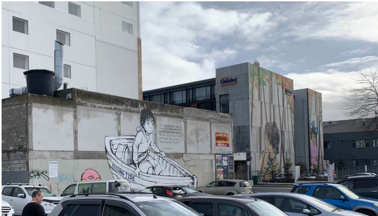
E View of the buildings which are located to the west of the proposed site. The vacant buildings along Manchester Street display murals/street art, post earthquake, and now play a role in the urban character of Christchurch CBD.
