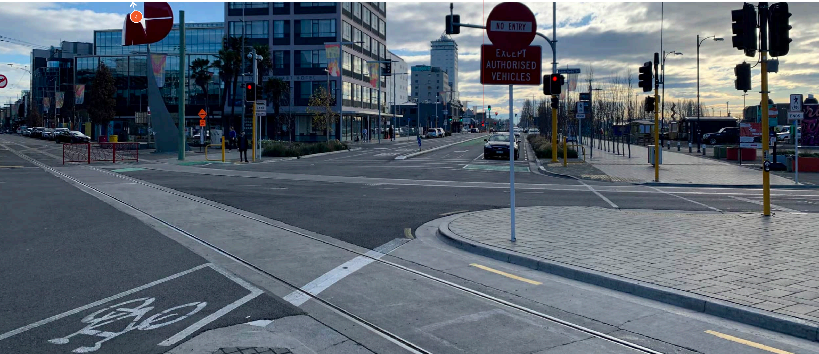
A. EXISTING VIEW
