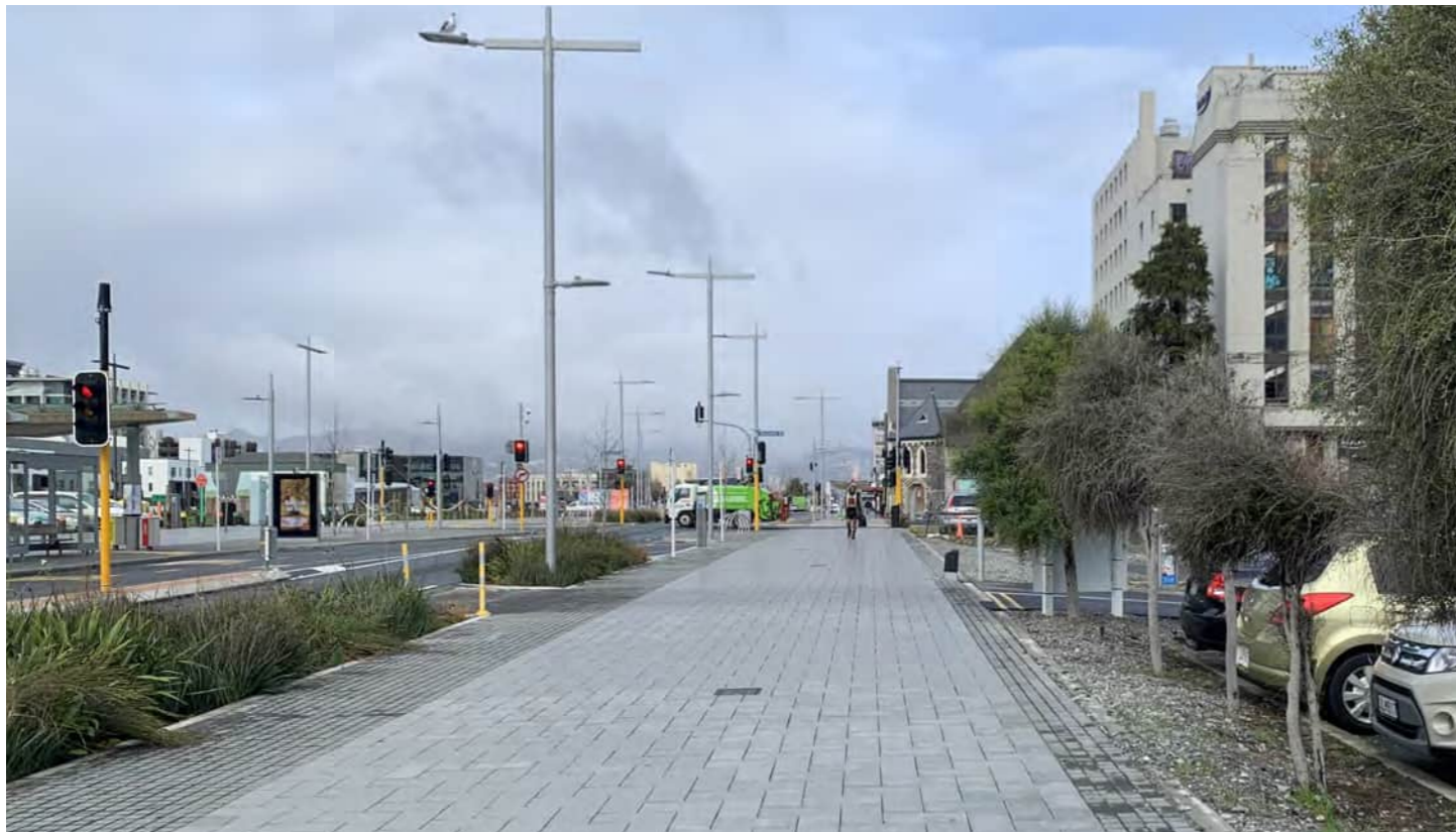
A View from the the proposed site looking down Manchester Street towards the historic Trinity Congregational Church, a site now owned by the Chrsitchurch Heritage Trust due to earthquake damage.
