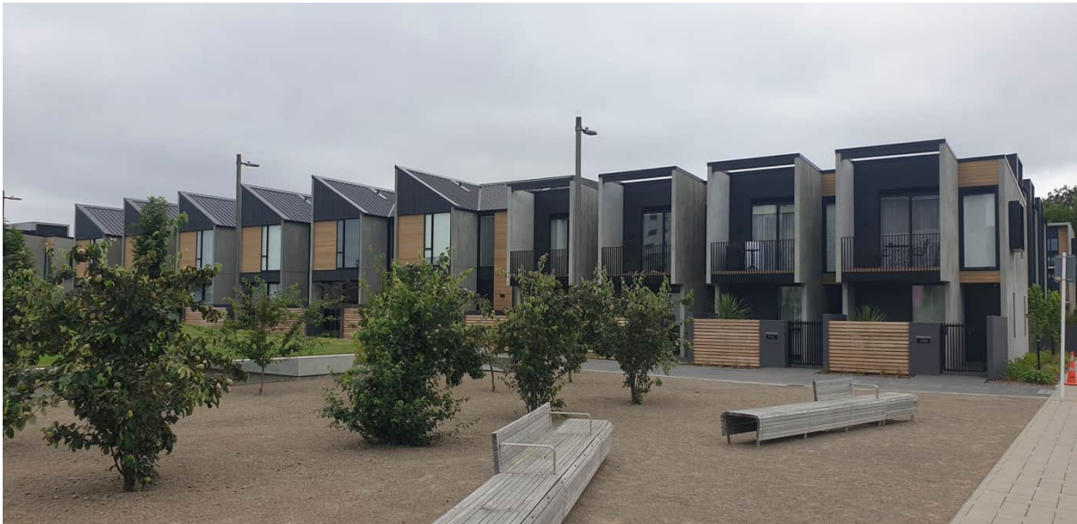
Photo1: Residential units under construction at 198 Gloucester Street
