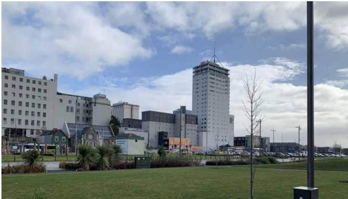
C View from adjacent greenspace of multi-storey buildings (Rendevous Hotel, earthquake damaged Kaplan Centre and Trinity Congregation Church, and Cathedral Junction Appartments), all have a view above the proposed site to the greenspace.
