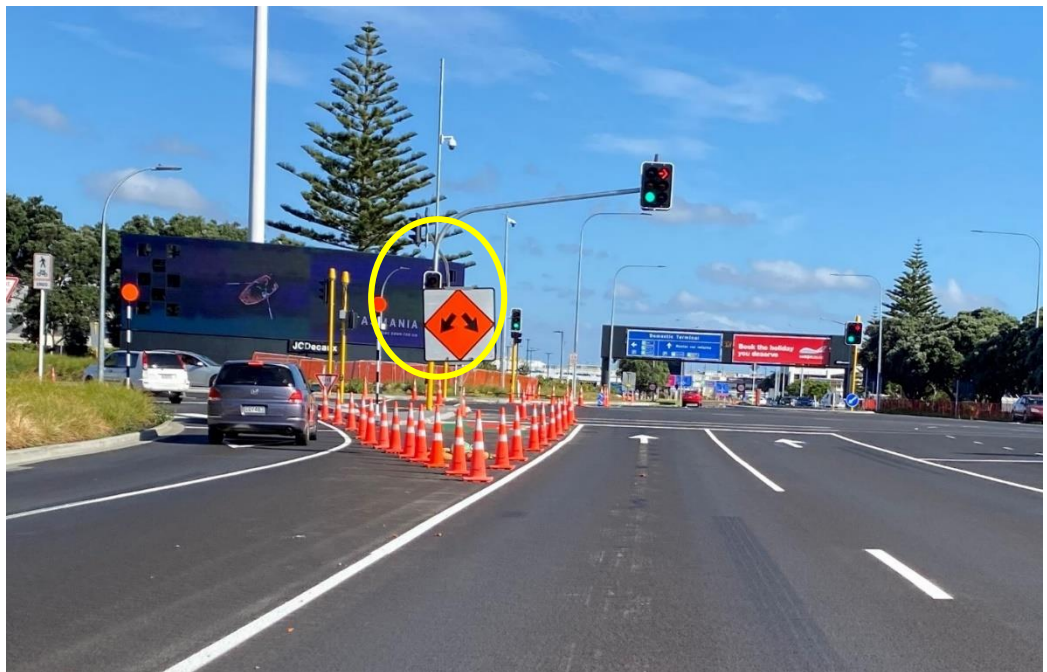
Photograph 4: Straight-Head Lane (Overlap with Primary Signal Highlighted, Behind Temporary Signage)
