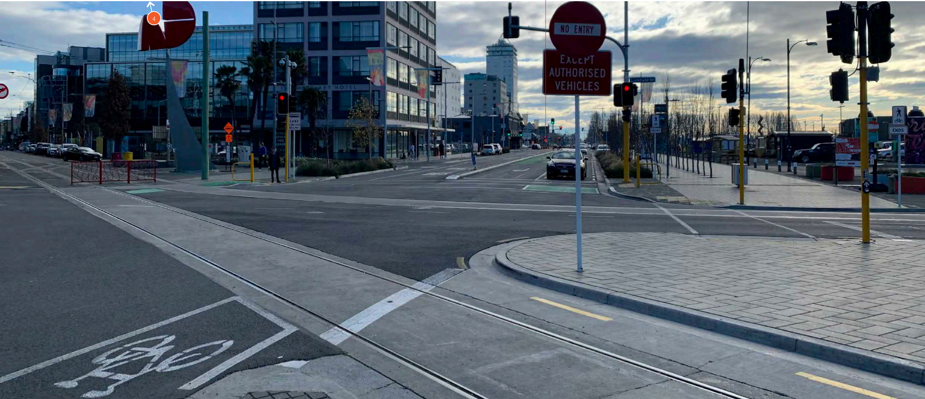
A. EXISTING VIEW
