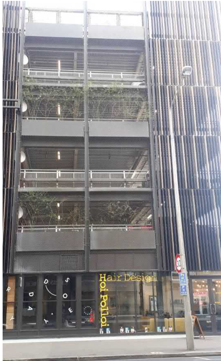
Photo 3: Climbers growing up the northern façade of the Westend carparking building in July
