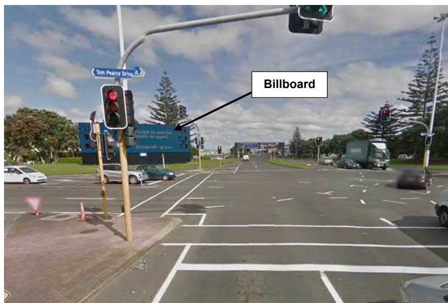
Figure 11: Digital Billboard at the George Bolt Memorial Drive / Tom Pearce Drive Intersection
