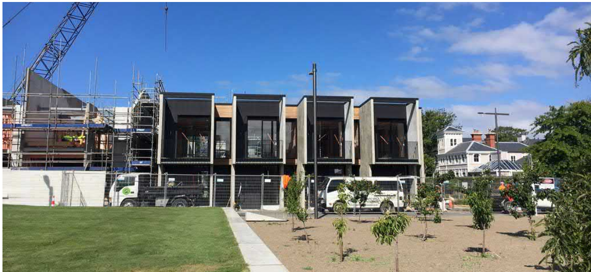
Photo1: Residential units under construction at 198 Gloucester Street
