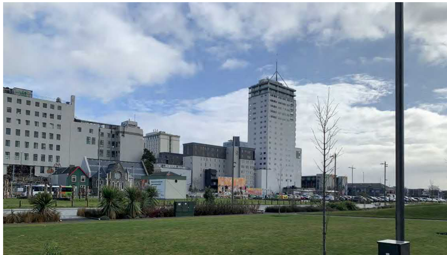
C View from adjacent greenspace of multi-storey buildings (Rendevous Hotel, earthquake damaged Kaplan Centre and Trinity Congregation Church, and Cathedral Junction Apartments), all have a view above the proposed site to the greenspace.
