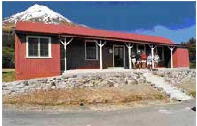
Surviving section of the old New Plymouth army barracks on Mt Taranaki, following restoration ( http://www.doc.govt.nz )
