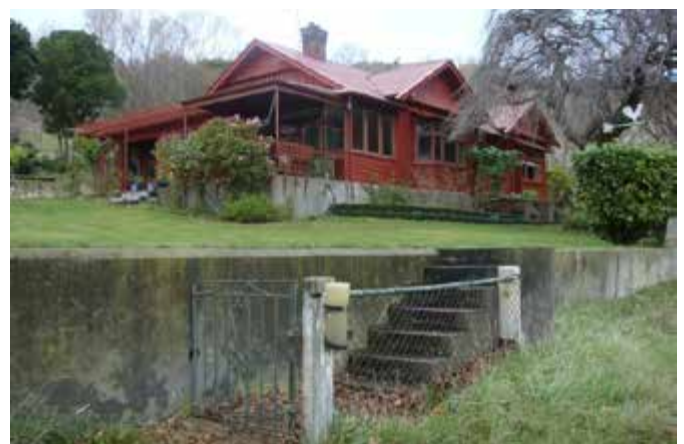
Steps and retaining wall below the house
