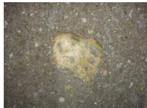
Mortar patch to monument stone
