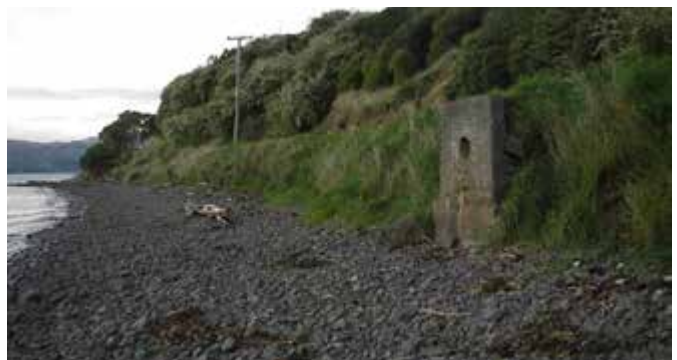
Concrete foundation for culvert (Mosley, May 2010)
