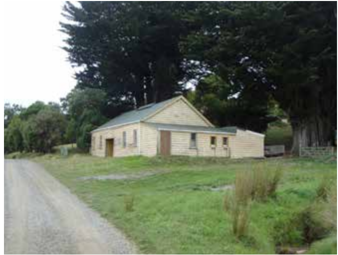
The barracks in context. Note macrocarpa trees behind building
