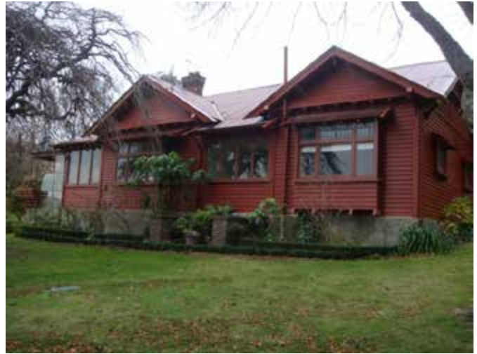
Red House viewed from the west. The area of wall between the two gables was formerly an entry. The steps are still in place
