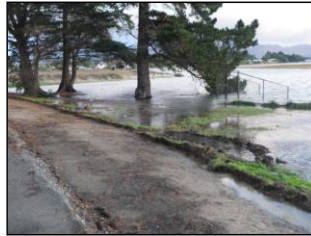
King tide flooding
