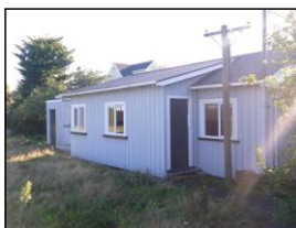
Former croquet club building in Blighs Garden
