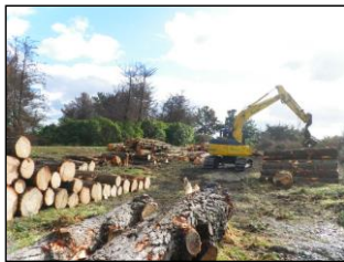
Tree removal in Bridge Reserve 2012
