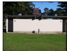
Old Toilet block
