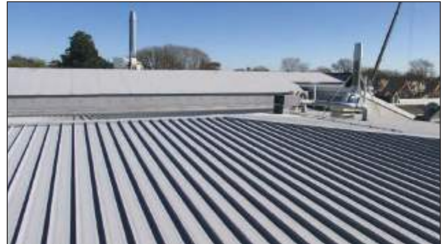
10.1 1995 General Roof Looking north
