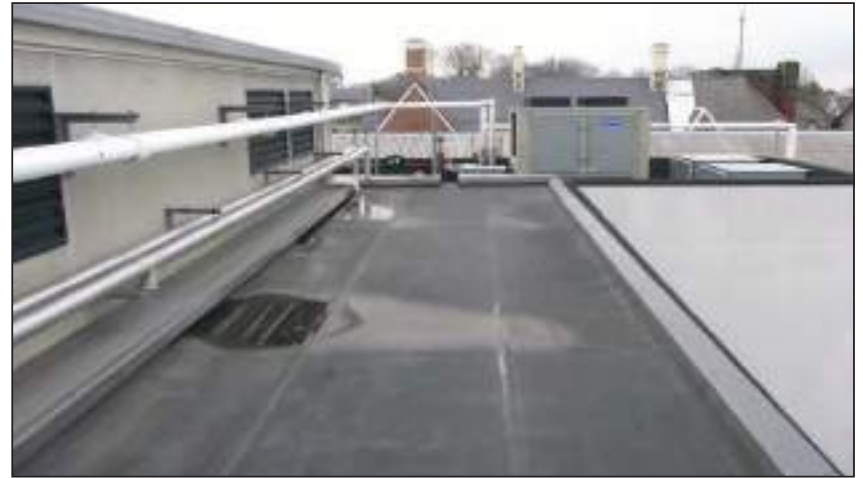
11.5 1995 General Walls Eastern wall and roof looking north
