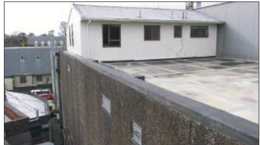
8.1 1995 Staffroom South elevation of staffroom
