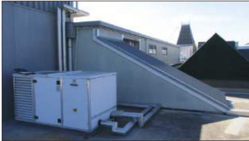
11.1 1995 General Walls Looking east from 1977 roof
