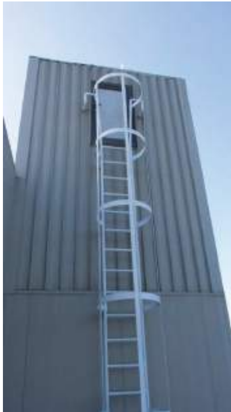
9.4 1995 Freezer panel store The lift overrun building
