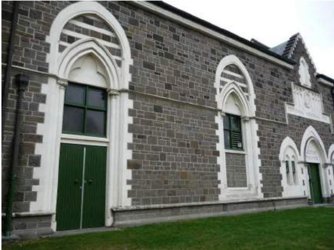
Fig.3. Centennial Wing Eastern Façade – View From Rolleston Ave.
