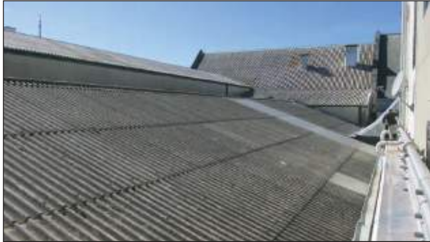
1.8 1958 Roof Looking east
