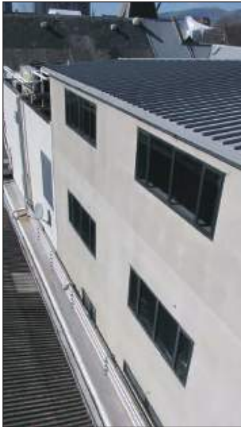
11.4 1995 General Walls North elevation of fibre cement board wall
