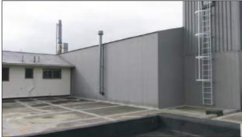
9.1 1995 Freezer panel store West side of the freezer panel building
