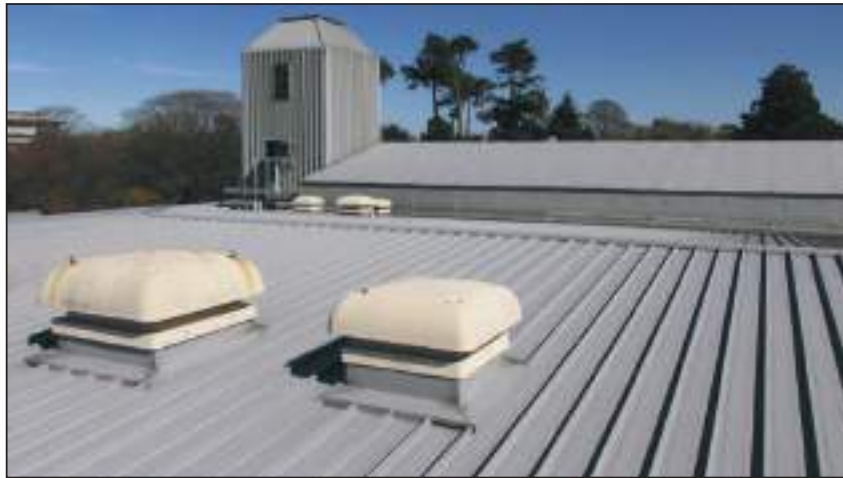
10.3 1995 General Roof Looking southwest
