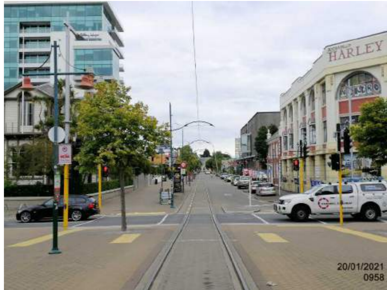
Worcester Boulevard Bridge View: Existing
