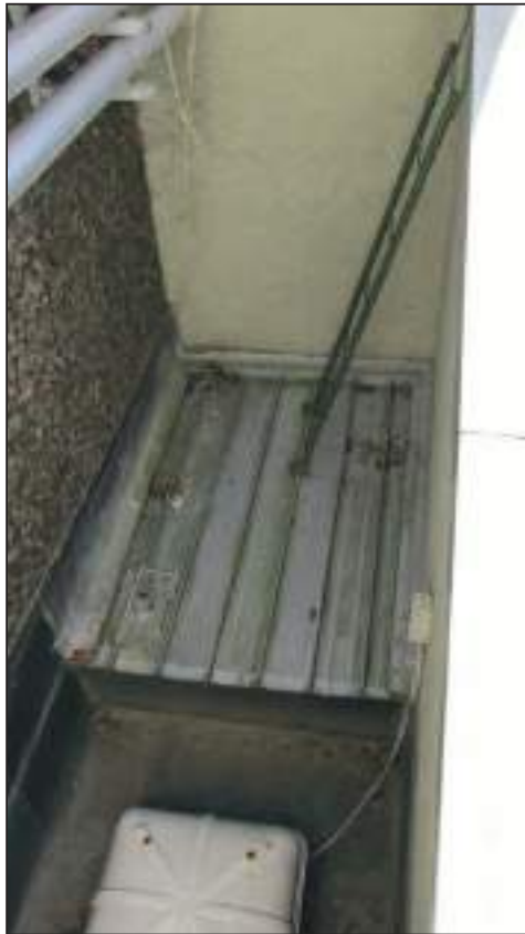
1.15 1958 Roof Looking down into the sump
