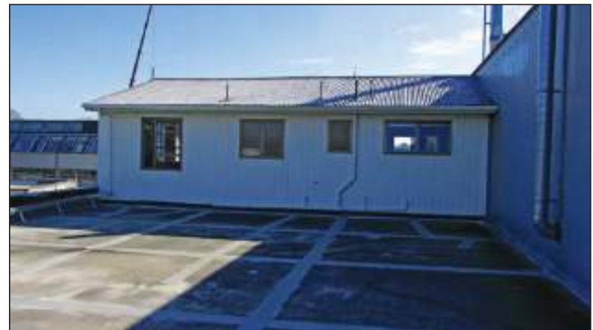
8.2 1995 Staffroom South elevation of staffroom
