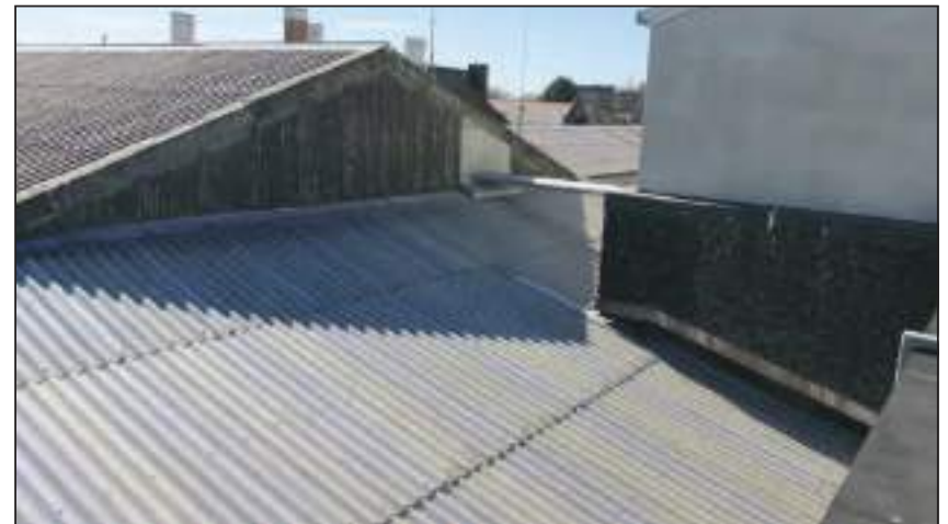
1.17 1958 Roof The asbestos roof adjacent to the staffroom outdoor patio
