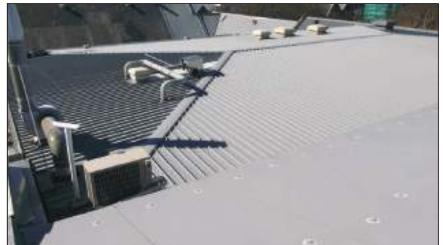
10.2 1995 General Roof Looking southeast
