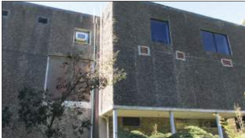
5.4 1977 Walls West elevation
