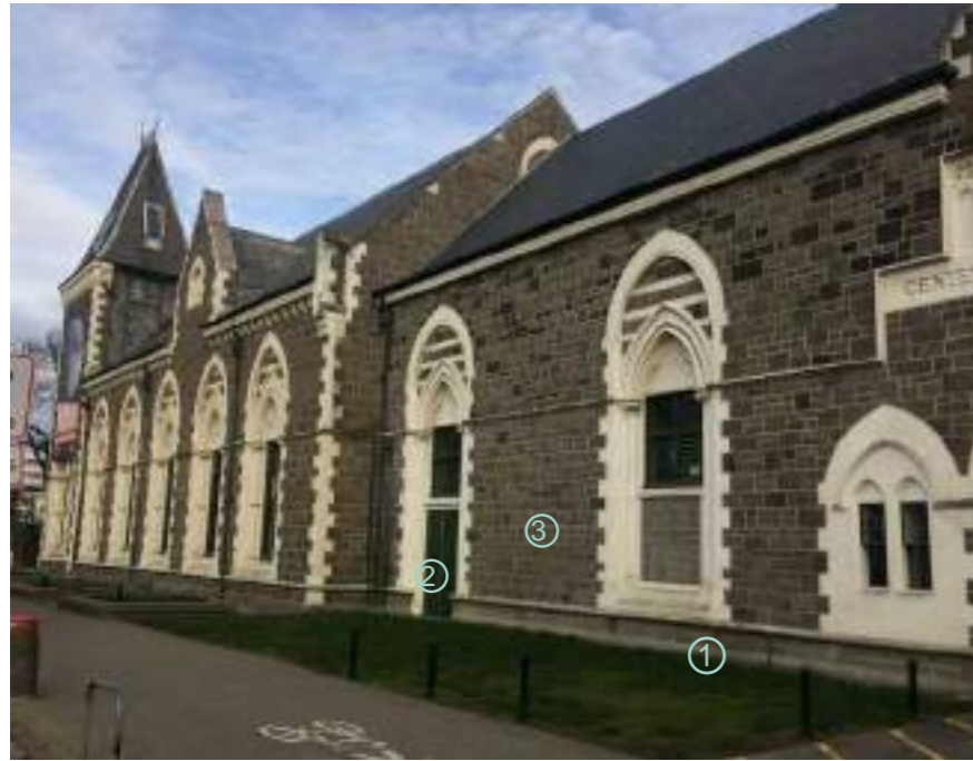
Centennial Wing windows - current conditions
