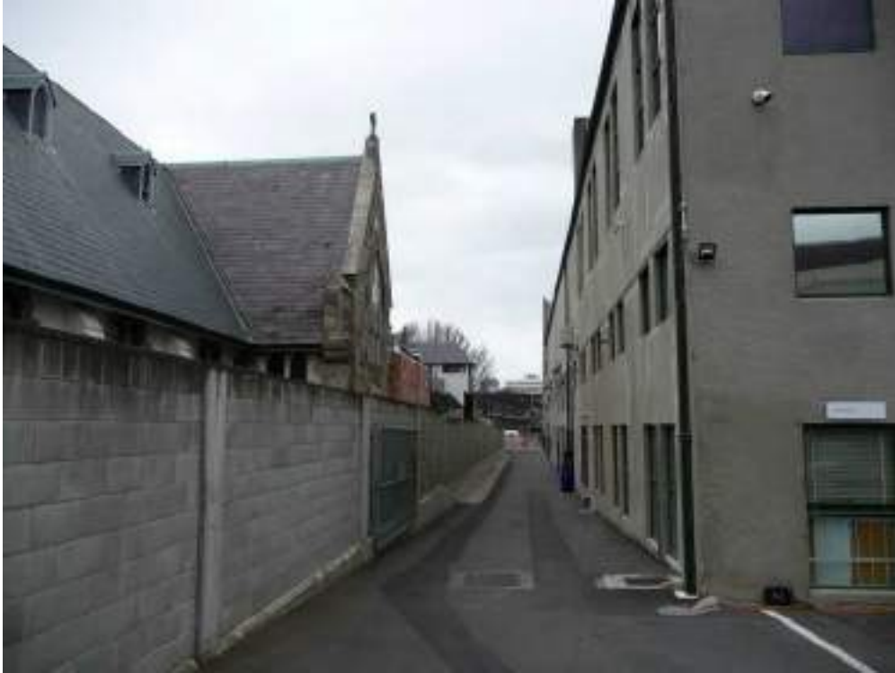
Fig.26. View along northern boundary - looking east down service lane toward Rolleston Ave.
