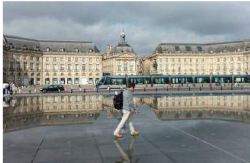
Miroir d'eau (Water Mirror), Bordeaux, France The reflecting pool is made of granite slabs, intermittently covered by 2cm of water, then drained away and a system allows it to create mist every 15 minutes.
