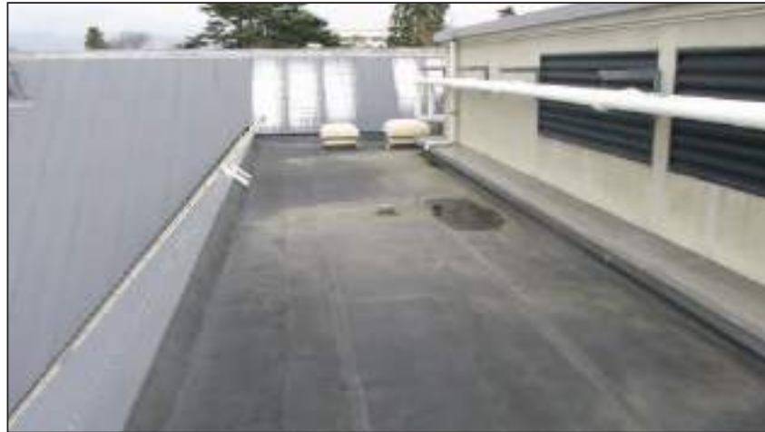
10.18 1995 General Roof East side looking south
