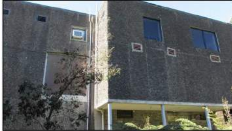
5.4 1977 Walls West elevation
