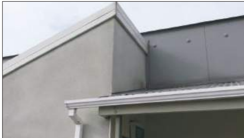
11.7 1995 General Walls Complex detailing adjacent to staffroom
