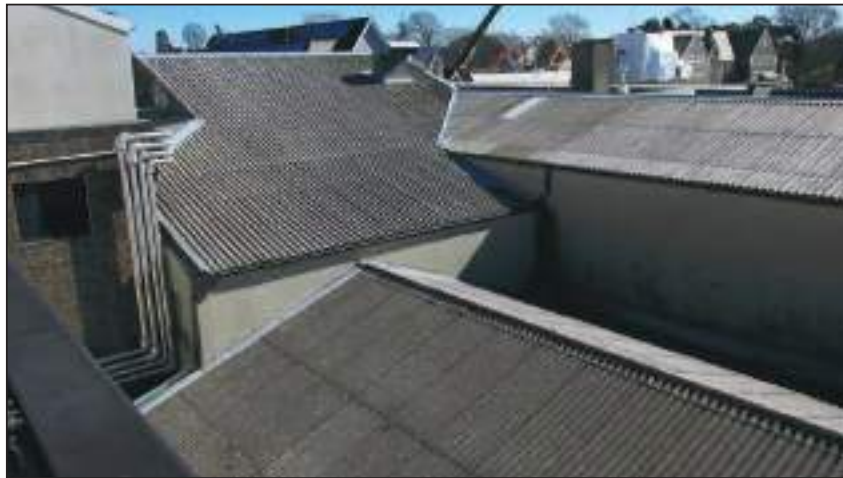
1.3 1958 Roof Asbestos roof looking northwest
