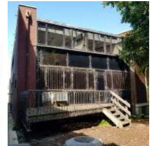
Canaday Wing - Current condition
