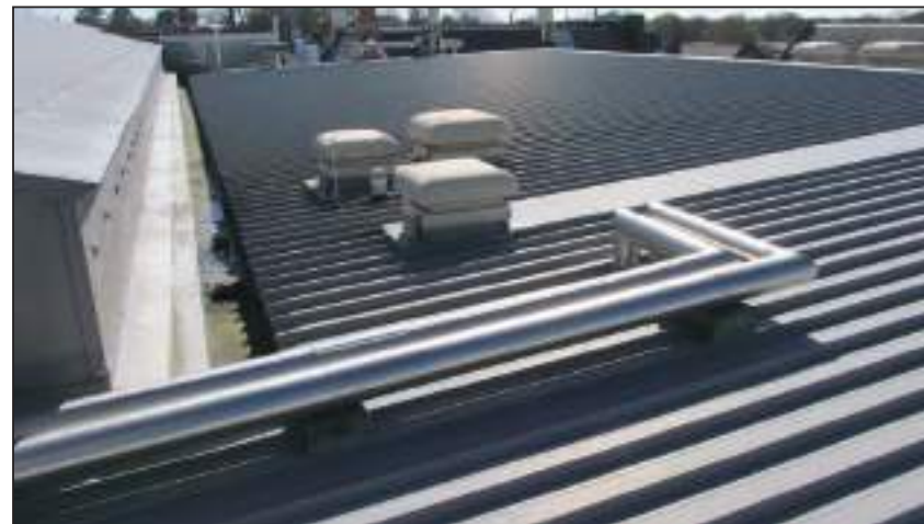
10.4 1995 General Roof Looking north
