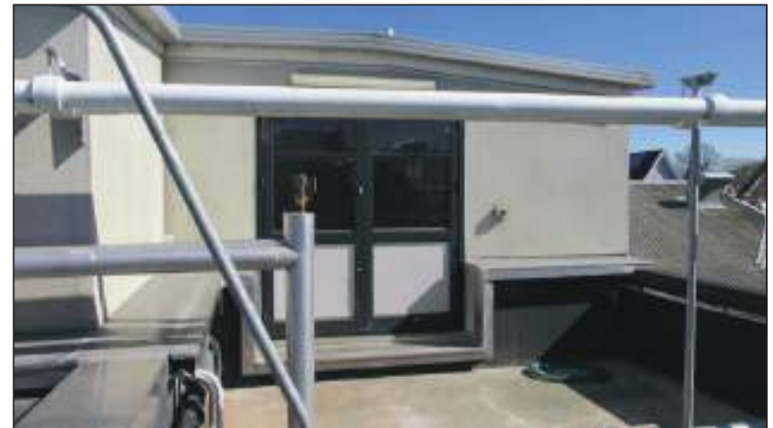
11.9 1995 General Walls Connection to the plant room area
