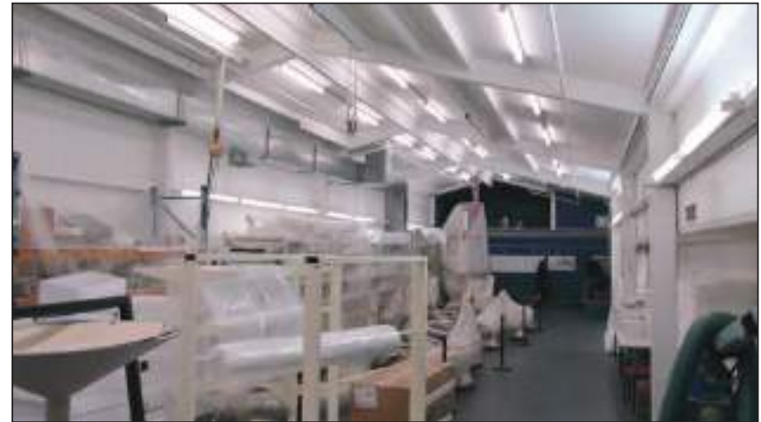
9.5 1995 Freezer panel store Interior of the freezer panel building showing the exposed structure to which the freezer panels are attached
