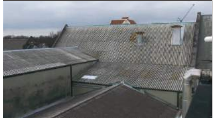
1.1 1958 Roof Asbestos roof looking to the east
