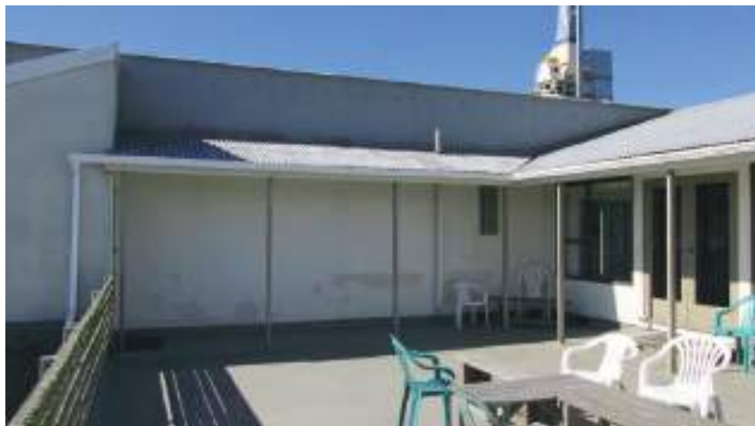
8.4 1995 Staffroom Connection of staffroom to freezer panel building
