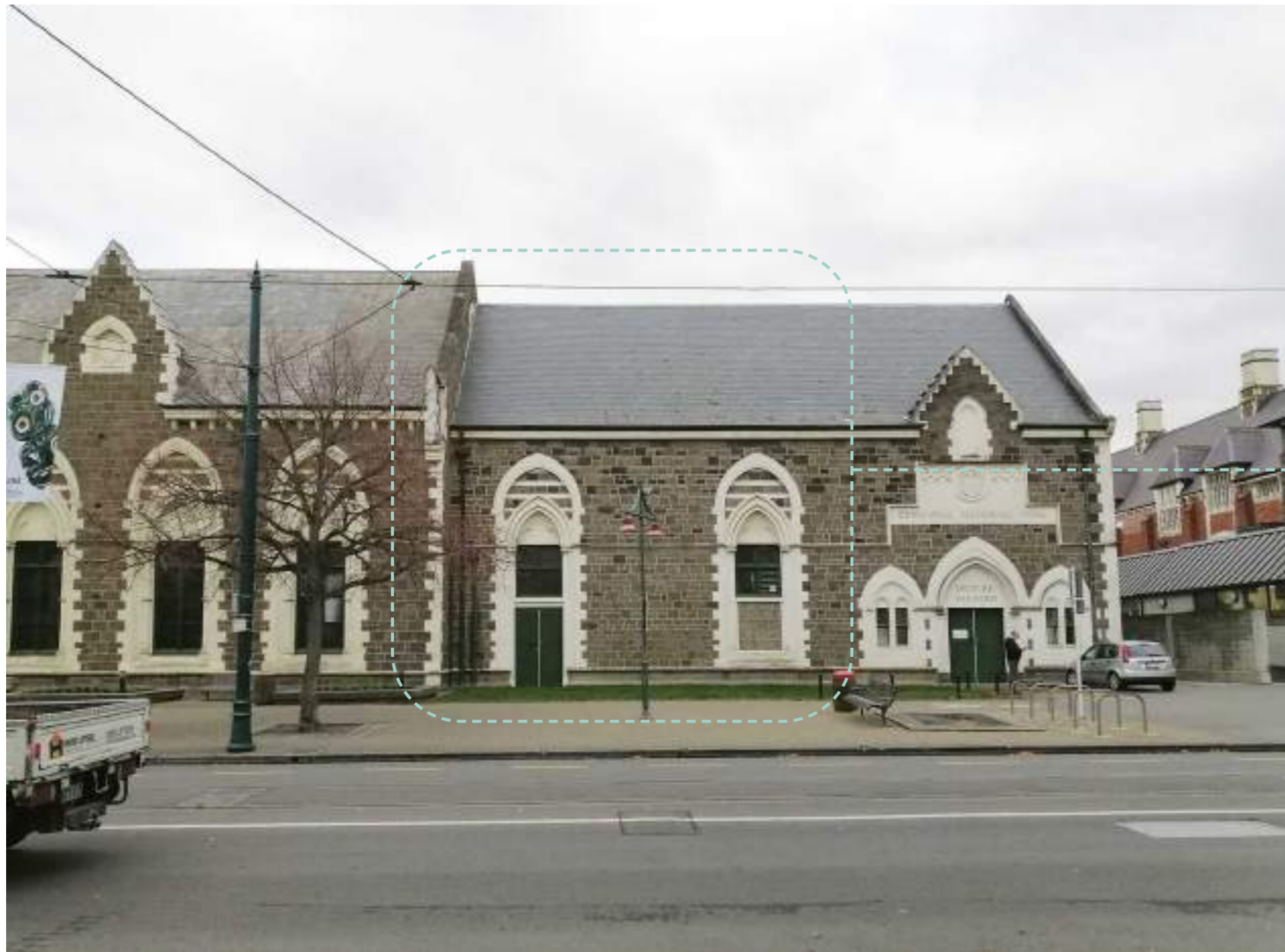
Existing Centennial Wing East Facade
