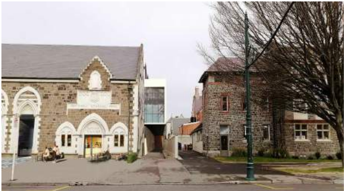
VP3 – From Rolleston Avenue - looking along northern boundary with Christ's College - proposed.
