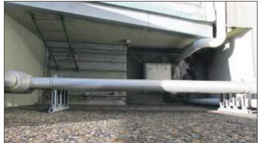
1.14 1958 Roof Looking down into the sump
