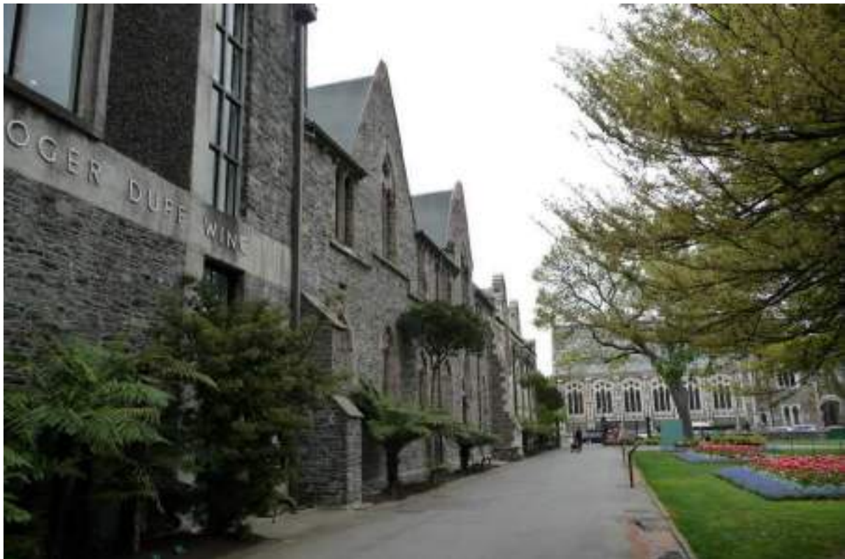
Fig.2. Canterbury Museum south façade – Roger Duff Wing, Mountfort 1872 and 1877 buildings. View from Botanic Gardens towards Arts Centre on Rolleston Ave.
