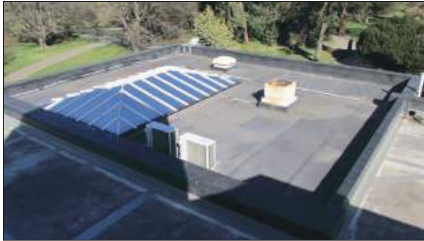
4.3 1977 Roof Looking southwest
