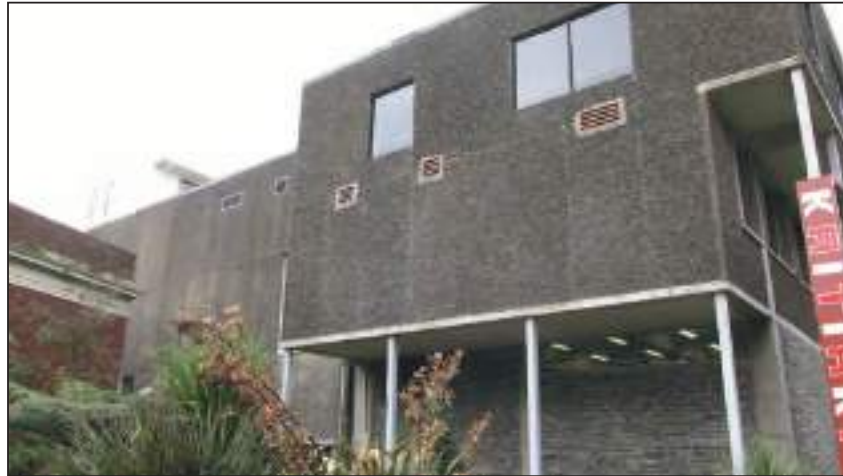
5.3 1977 Walls West elevation
