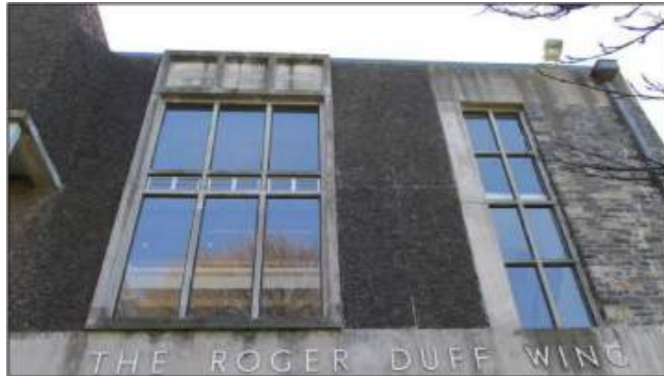
5.5 1977 Walls Part south elevation
