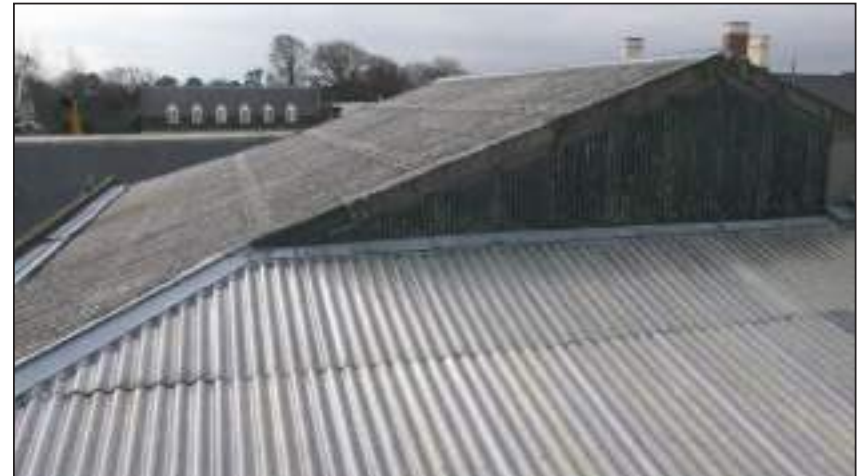
1.6 1958 Roof The western end of the asbestos roof
