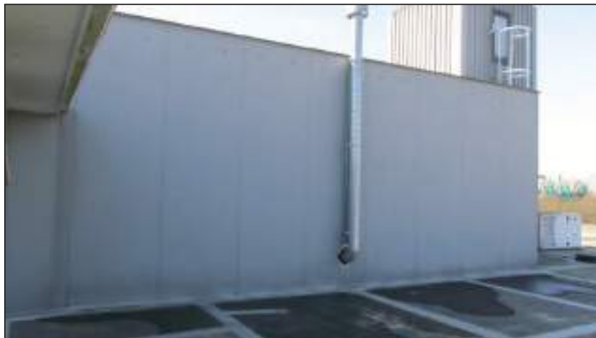
9.2 1995 Freezer panel store West side of the freezer panel building
