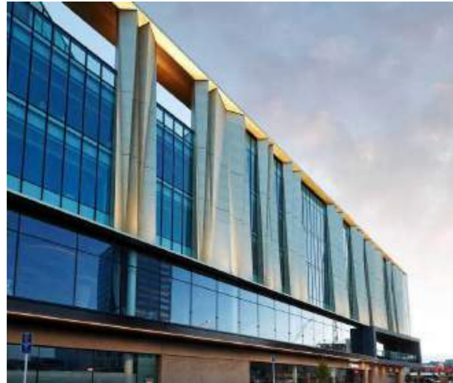
Example of APL Structural Glaze - Tūranga Christchurch Central Library
