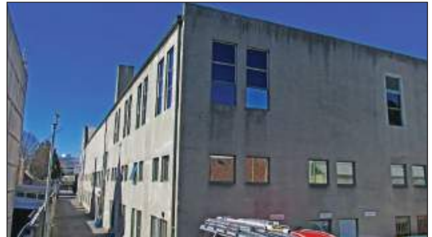
2.2 1958 Walls North and west elevations
