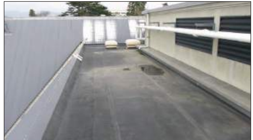
11.6 1995 General Walls Eastern wall and roof looking south
