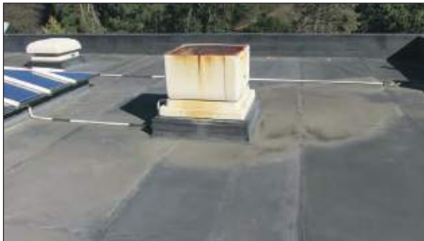
4.4 1977 Roof Original roof without a topping slab added
