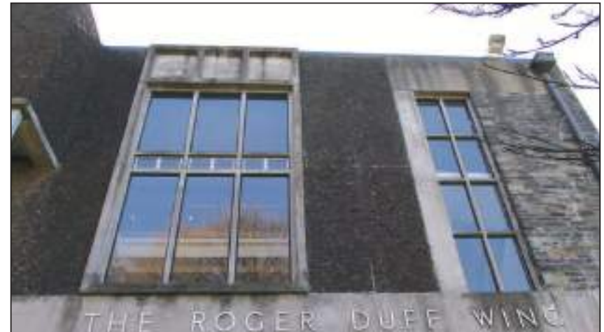
5.5 1977 Walls Part south elevation
