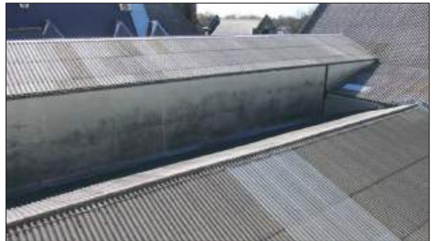
1.2 1958 Roof Asbestos roof looking north
