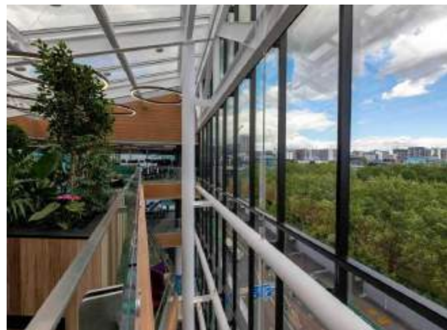
Example of APL Structural Glaze - 155 Fanshaw Street, Auckland, 5 Greenstar Rating
