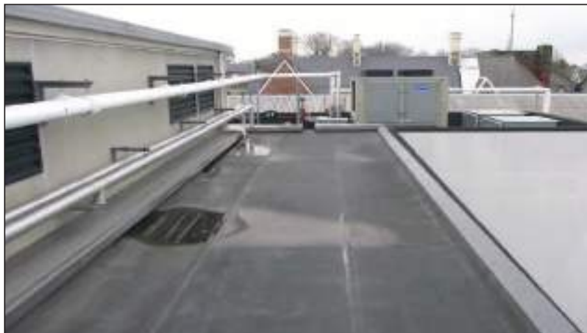
10.19 1995 General Roof East side looking north
