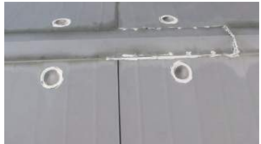
9.9 1995 Freezer panel store Surface applied sealant to fixing bolts
