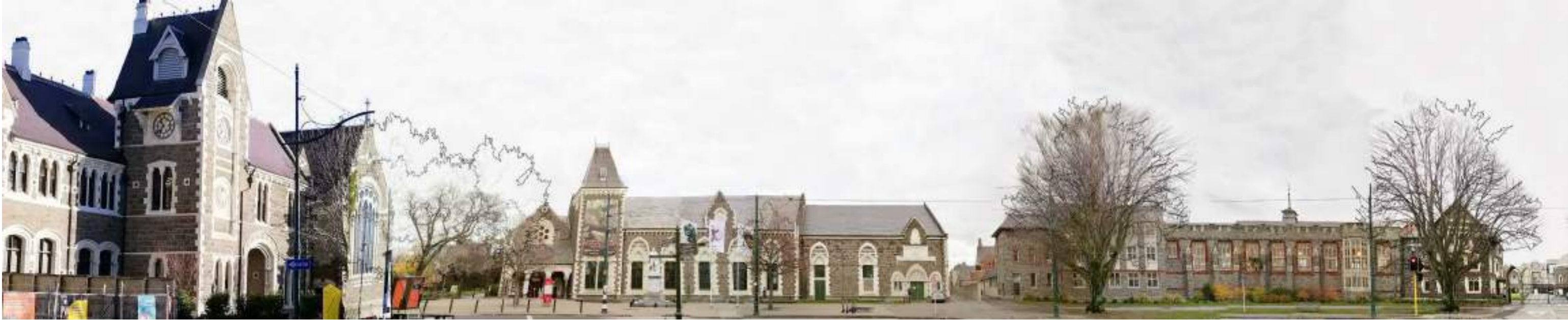
Existing conditions viewed from Rolleston Avenue
