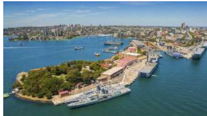
Ardex WPM 1500 and hydro stop were used in the Green Island Naval Base 1500mm below the Sydney Harbour waterline. (image: Ardex)
