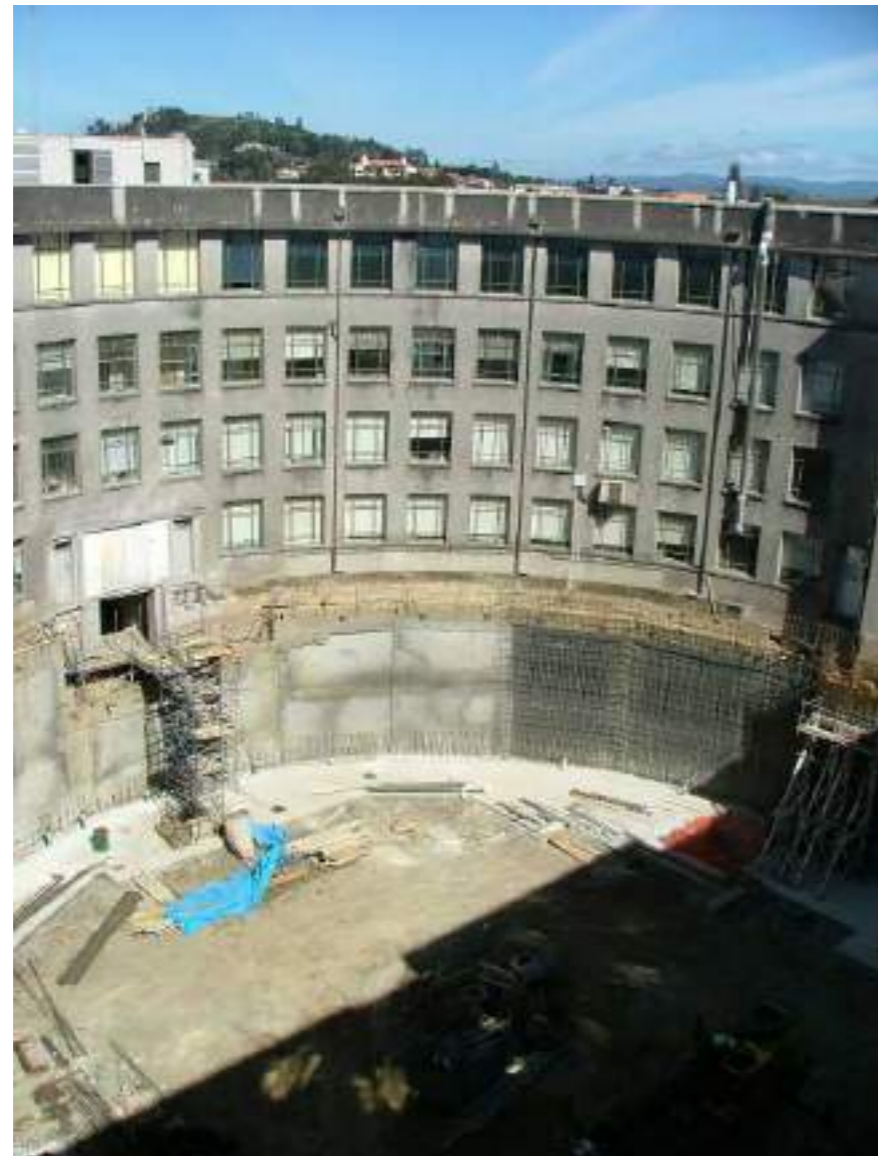
Auckland War Memorial Museum basement construction. (image: Allco)
