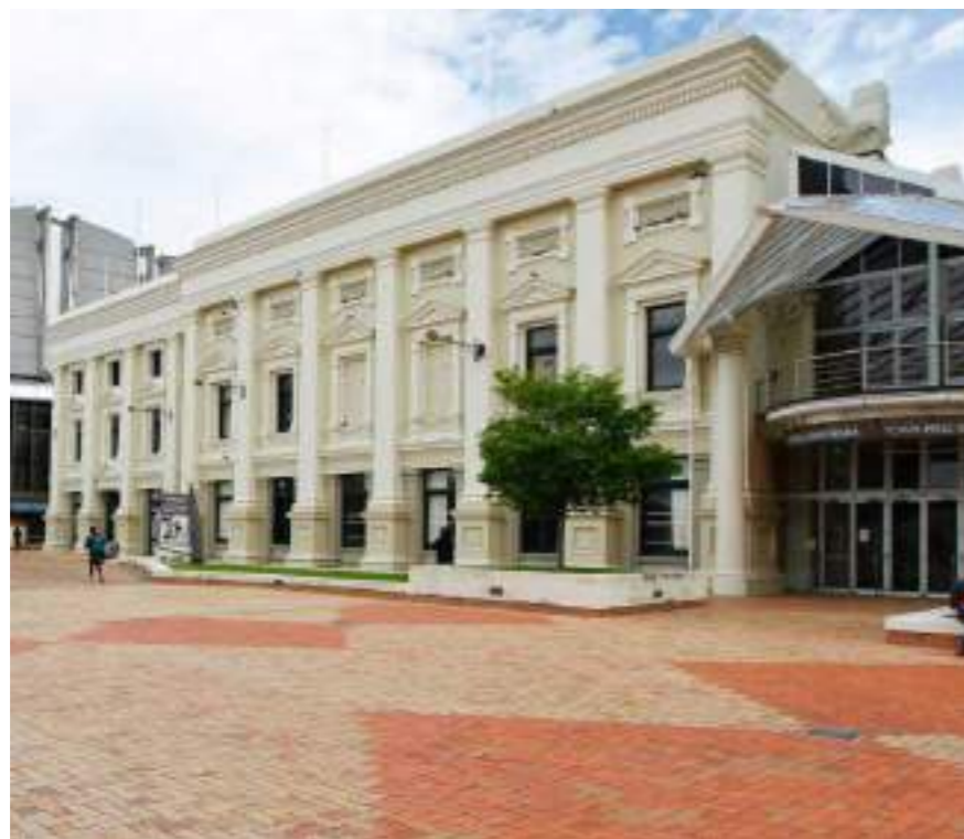
Wellington Town Hall is being strengthened and upgraded. View from Civic Square of Wellington Town Hall, as it looks in 2013.
