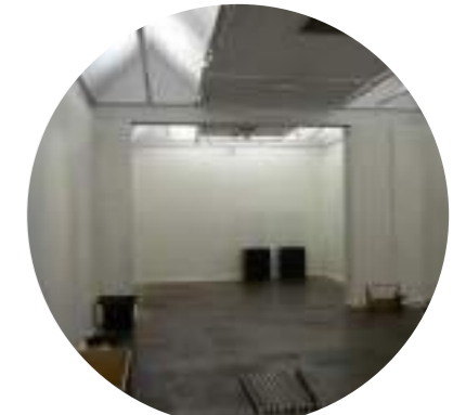
Gallery room current condition (image: DPAL, refer to RMG Conservation Plan for more information)
