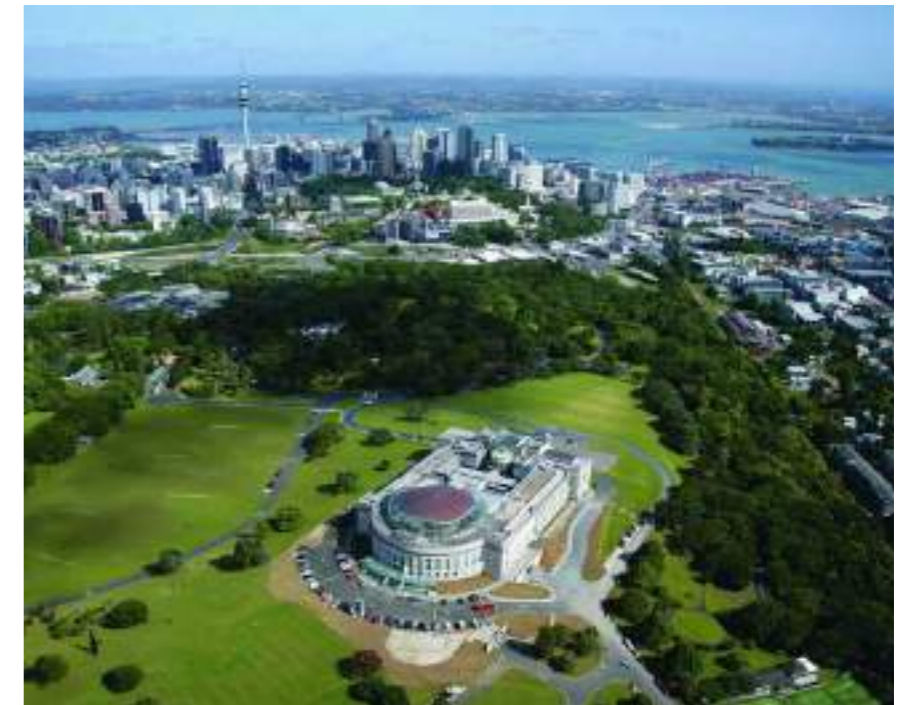
Auckland War Memorial Museum after renovation. (image: Holmes Consulting)
