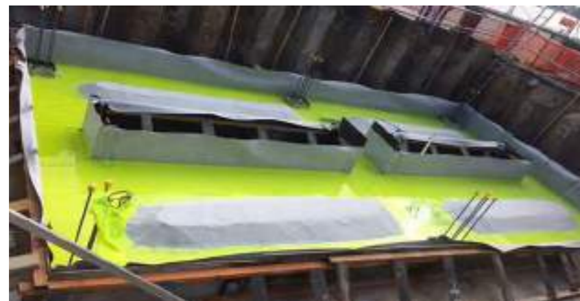
Green Island Naval Base Weldtec membrane application. (image: Ardex)
