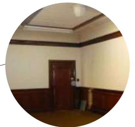
Restore Boardroom with Tasmanian Blackwood panelling and picture rail, architraves and door (image: DPAL, refer to RMG Conservation Plan for more information)
