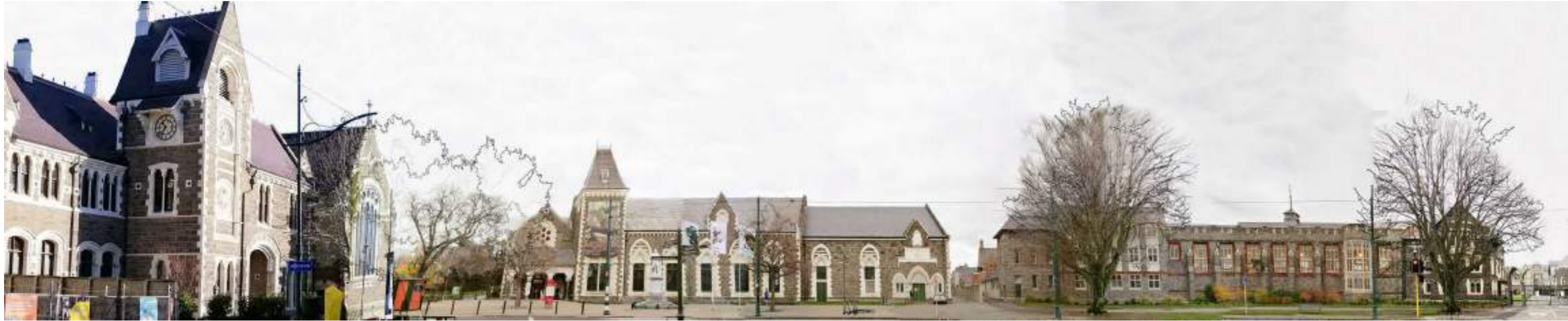
Existing conditions viewed from Rolleston Avenue
