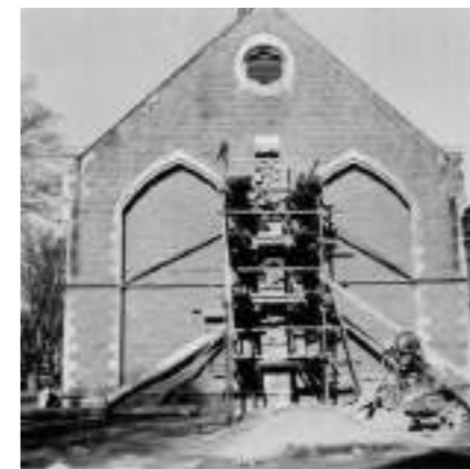
Removal of the 1872 buttress during Centennial Wing construction
