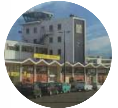
Folding roof (pictured: Christchurch Airport, now demolished, by Paul Pascoe 1960)
