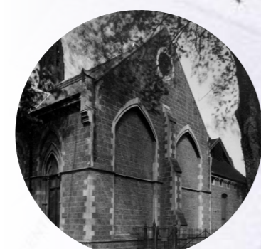
Expose hidden 1877 Mountfort building north facade
