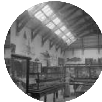
Restore Mountfort 1882 building to expose original roof truss
