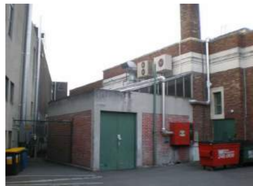
RMG workshop, entry from Museum service lane, RMG can be seen to the right
