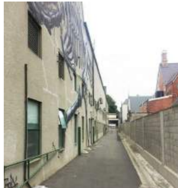
Service lane on the northern boundary, RMG night entry at the rear end
