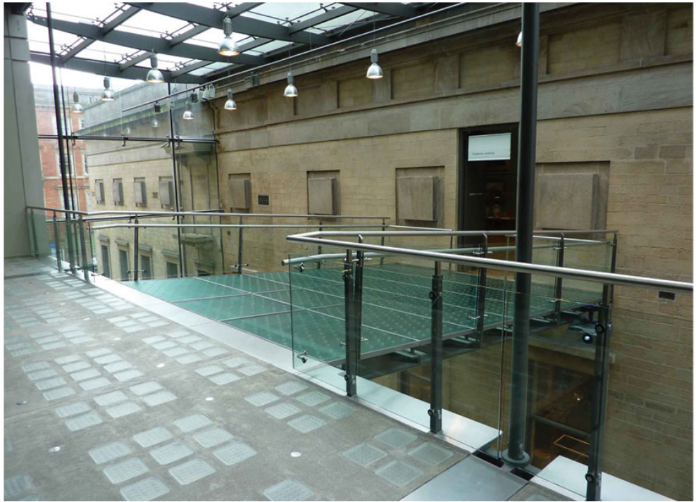
Image 18: Example of double height stone heritage wall being able to be legible from inside to outside. (note that in this case there is a glazed wall and roof connection). Manchester Art Gallery. Hopkins Architects (source: Anglezarke, 2009)
