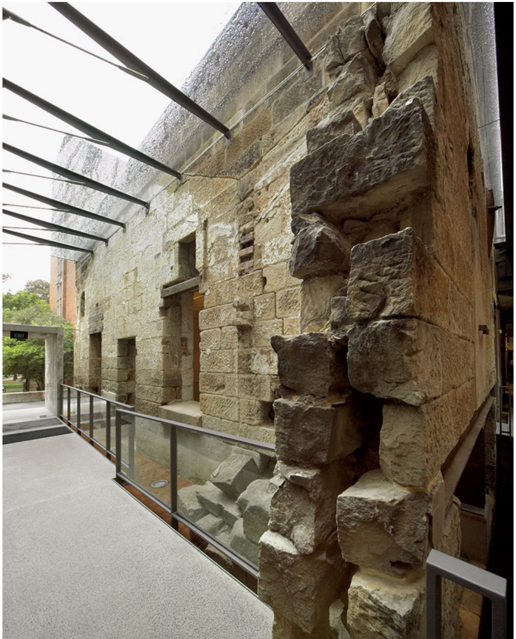
Image 20: Example of heritage stone wall with glazed separation to wall and roof allowing full appreciation of heritage wall inside and out. This image also highlights one benefit of the proposed open (non-glazed) separation in that even with glazing providing a high level of openness, you still get structure, reflections and rain which reduce visibility. The Mint, Sydney, FJMT Architects, 2002 (source: John Gollings)
