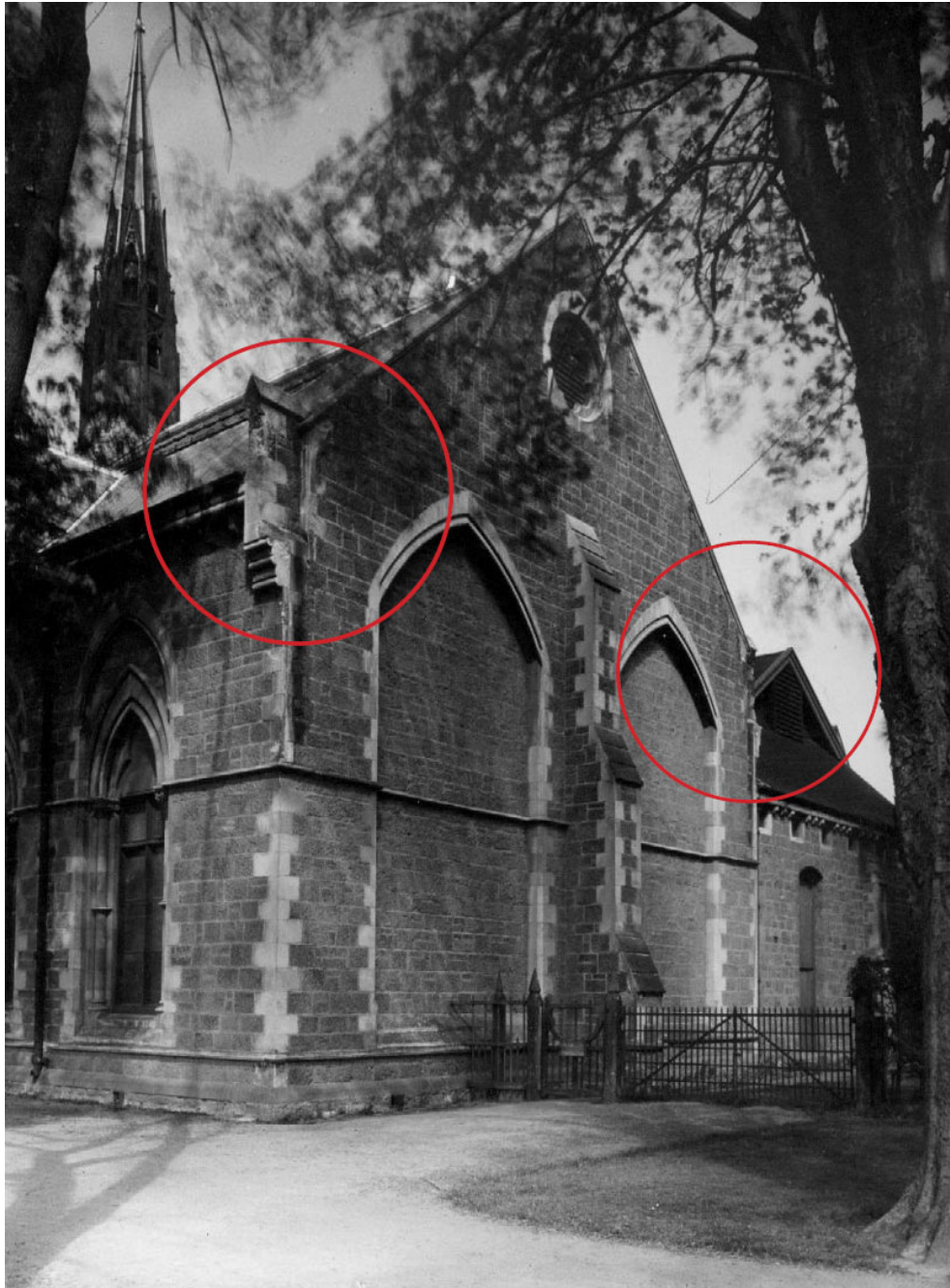
Image 24: 1877 Mountfort Building, north wall pre-1958. The central buttress has been demolished with the construction of the 1958 building, however all evidence suggests that all of the remainder of this façade will be able to be revealed to the public as part of the redevelopment, including the corbel detail (within right-hand circle) (original image source: Canterbury Museum archives)
