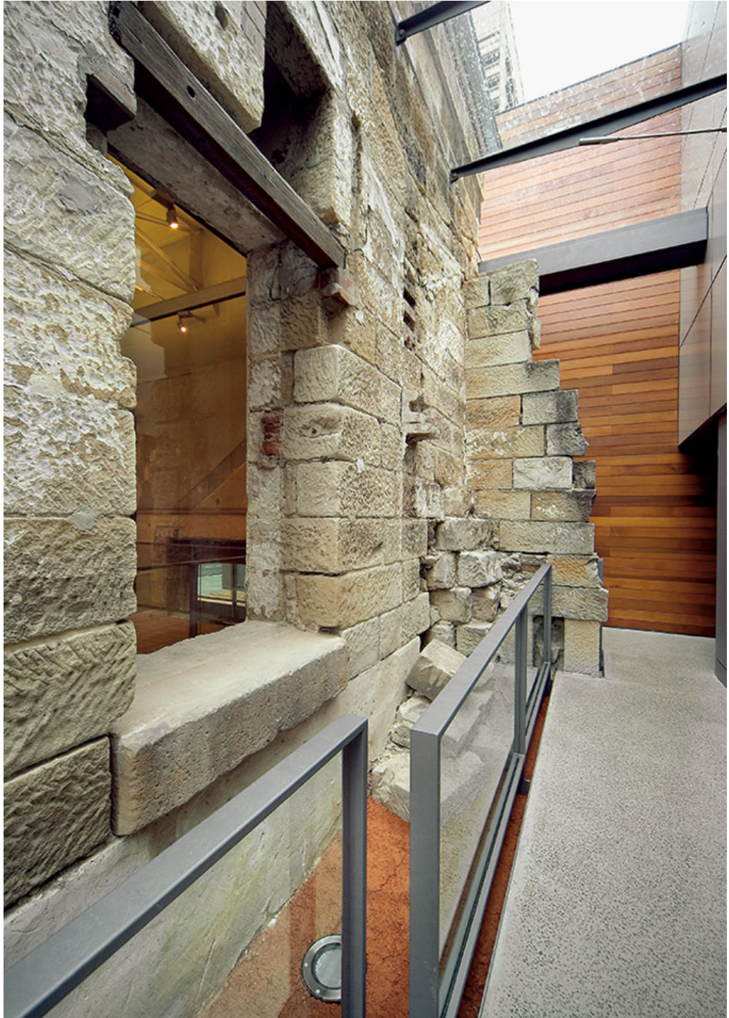
Image 21: Example of heritage stone wall with glazed separation to roof allowing greater appreciation of heritage wall inside and out. This image also highlights similar aspects to the separation between the 1877 & 1958 wings; the clear separation of new structure from primary significance even at floor level, the natural light grazing down the uneven stonework, the appreciation of the heritage wall even within a narrow space in this case a narrow corridor space) The Mint, Sydney, FJMT Architects, 2002 (source: John Gollings)
