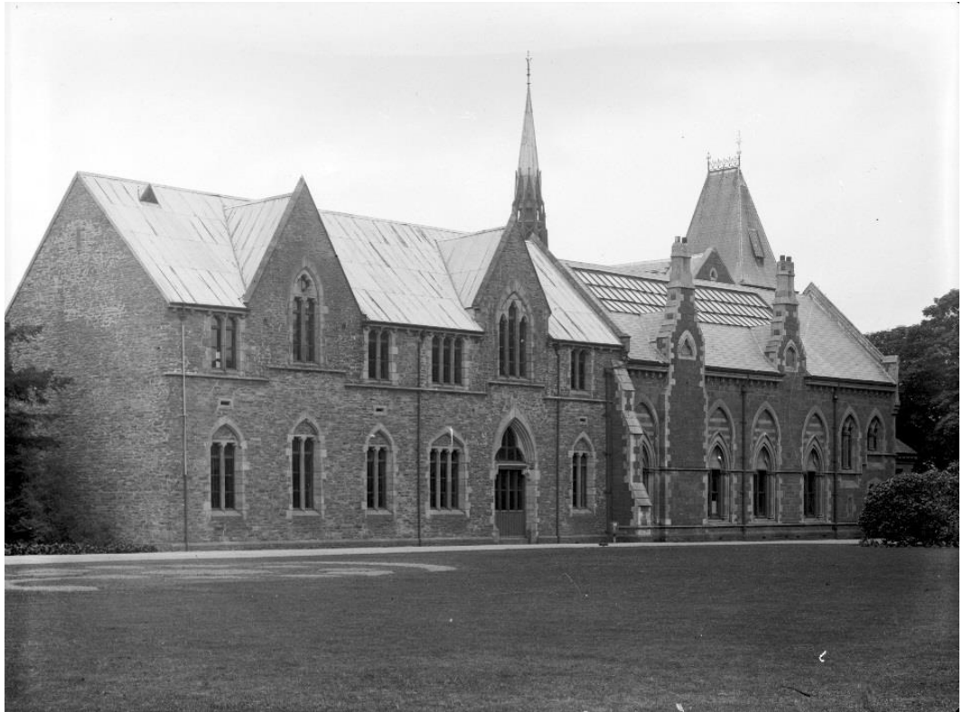
Image 31: View from Botanic Gardens showing 1872 & 1877 Wings. The benefit of the wider glazing proposed to the existing 1977 façade adjacent to the 1872 Mountfort building is that it will provide greater legibility of the Mountfort era and the gabled form of the west 1872 facade will be unveiled (albeit without the stone) (source WA Taylor photograph, Canterbury Museum archives)
