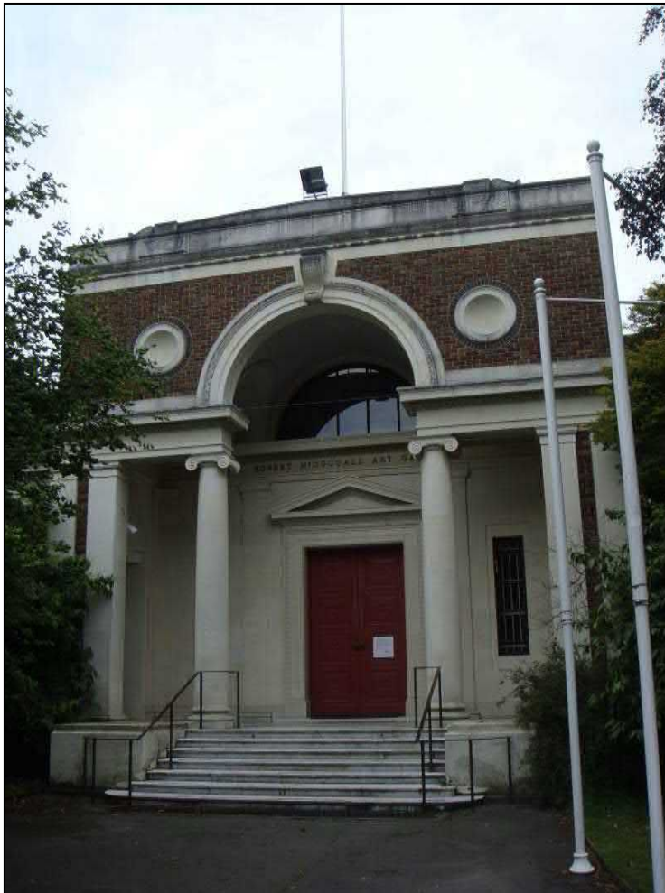
Central front entrance to Robert McDougall Gallery with floor above. (DPAL)
