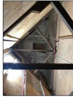
(3) Roof space showing trusses (OHF) and plywood bracing. (NHF)
