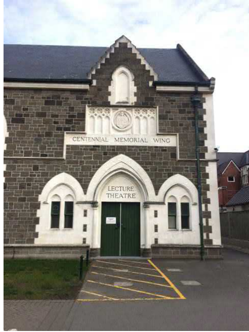
Figure 18. Original Rolleston Avenue entrance of the Centennial Wing (Source: Athfield Architects)
