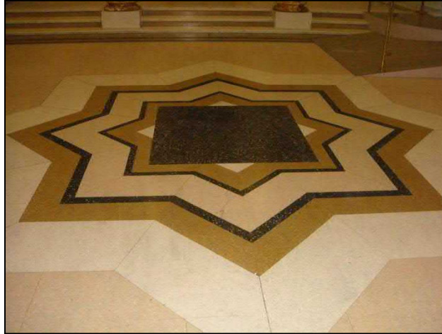
Terrazzo floor in sculpture court (DPAL).
