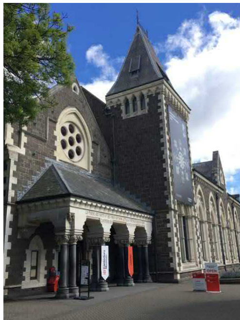
Figure 12. 1877 building and 1878 porch from Rolleston Avenue (Source: GJM Heritage)
