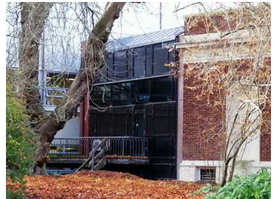
Figure 29. West elevation of the Canaday Wing (Source: Athfield Architects)
