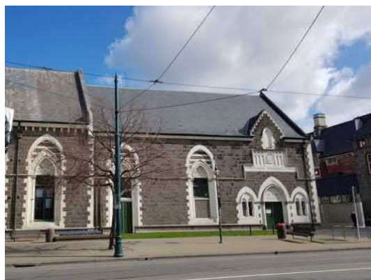
Figure 16. Rolleston Avenue (east) elevation of the Centennial Wing (Source: Athfield Architects)
