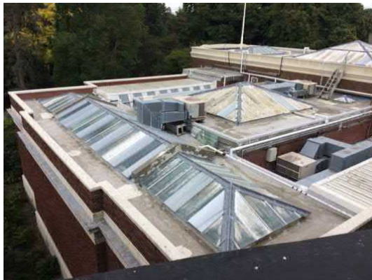
Figure 28. Robert McDougall Art Gallery roof (Source: Athfield Architects)
