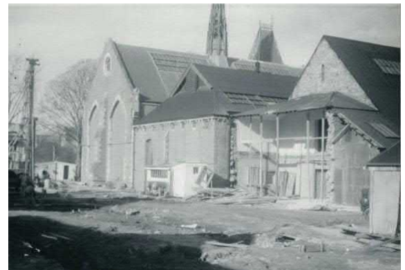
Figure 5. Construction of the Centennial Wing, 1955 (Source: Canterbury Museum)
