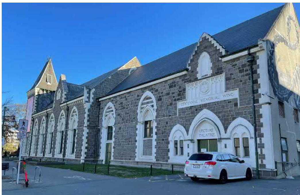
Photograph: Rolleston Avenue façade, juncture between 1877 and 1958 buildings, viewed from the North, A. Ohs 5 May 2021
