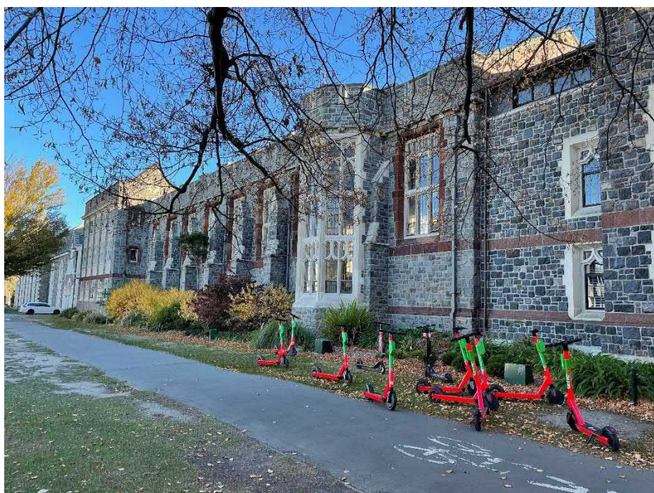
Photograph: Christ's College Rolleston Avenue façade. 1980s addition, far left. A. Ohs, 5 May 2021.
