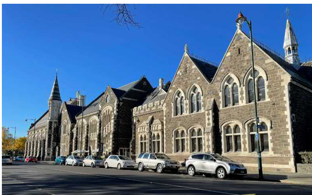
Photograph: Christchurch Arts Centre, Rolleston Avenue façade from South. A. Ohs 5 May 2021
