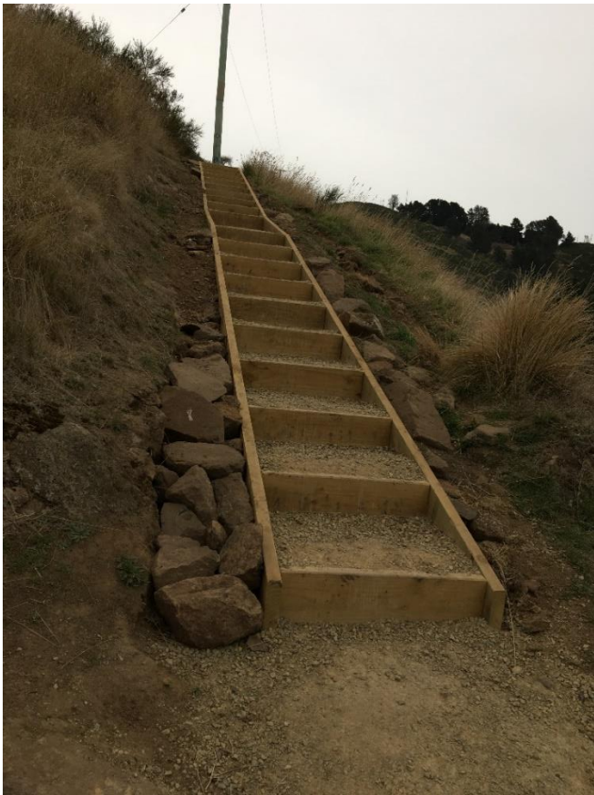
Longer flight of new wooden stairs built on Crater Rim Walkway May 2020. Rocks which previously were steps placed to sides
