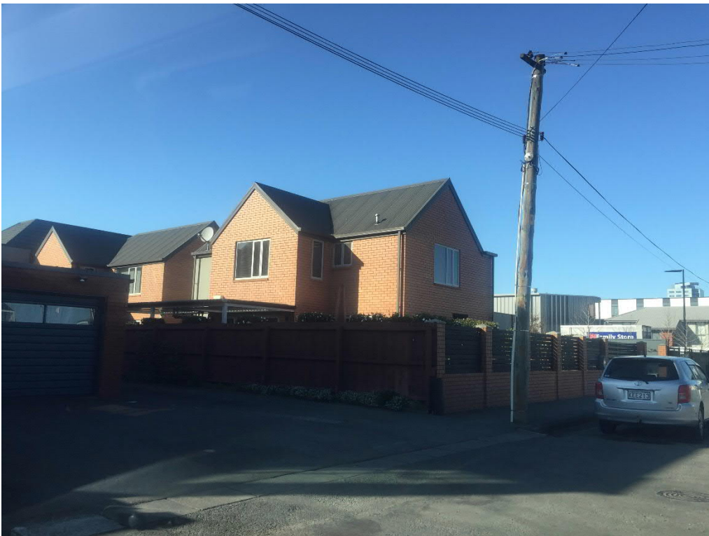
16 Gracefield Avenue on the eastern side opposite the proposed Manager's house.
