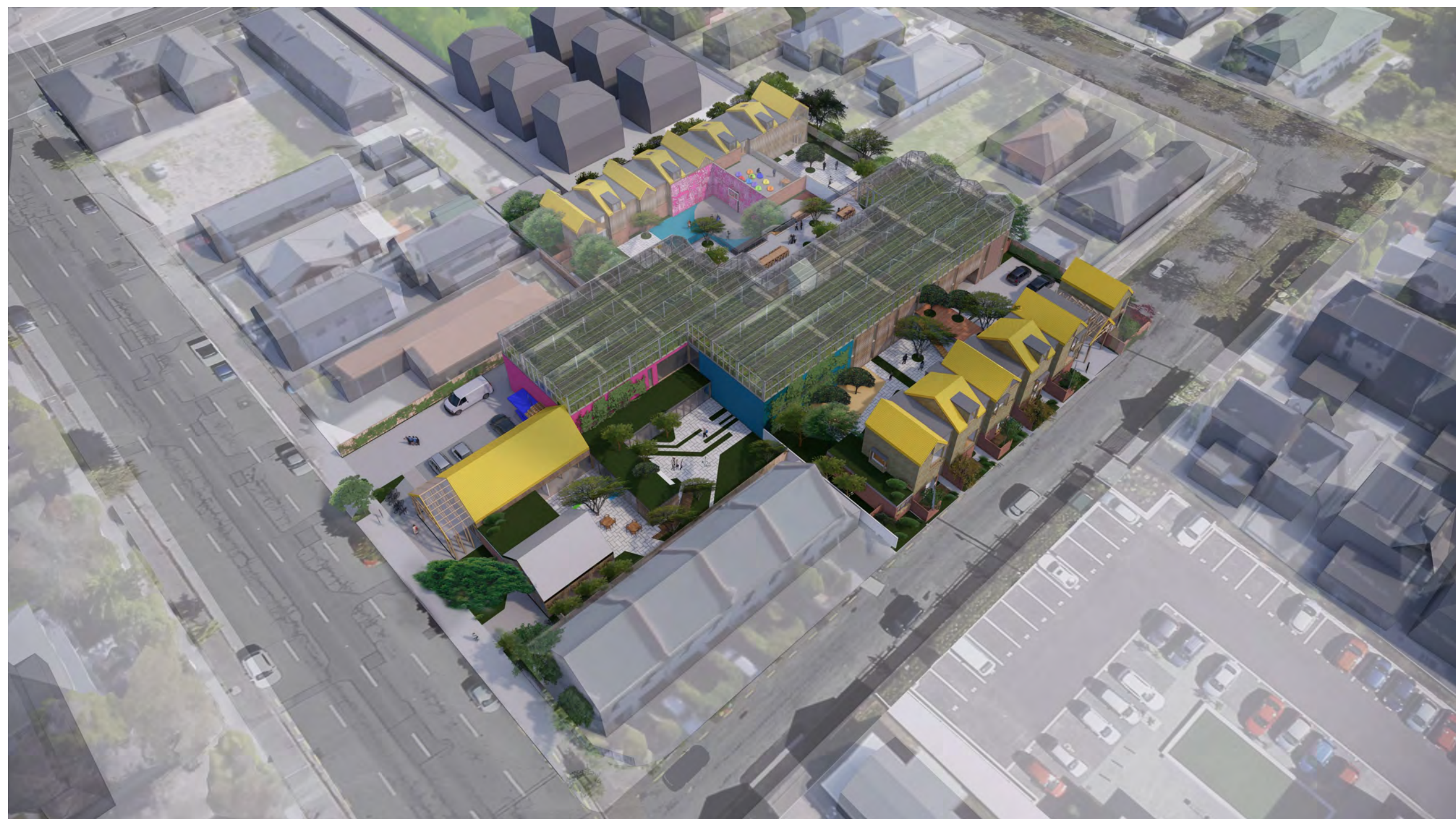
Over view of site from south east
