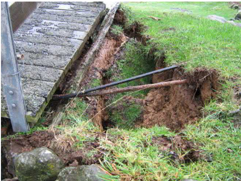
Damage to the above bridge caused by floodwaters undercutting the structure.
