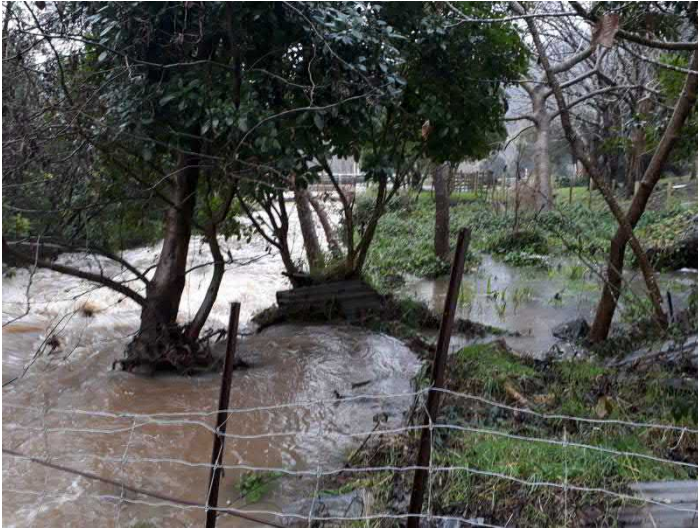
Water pooling next to the historic Pavitt Cottage during heavy rain.
