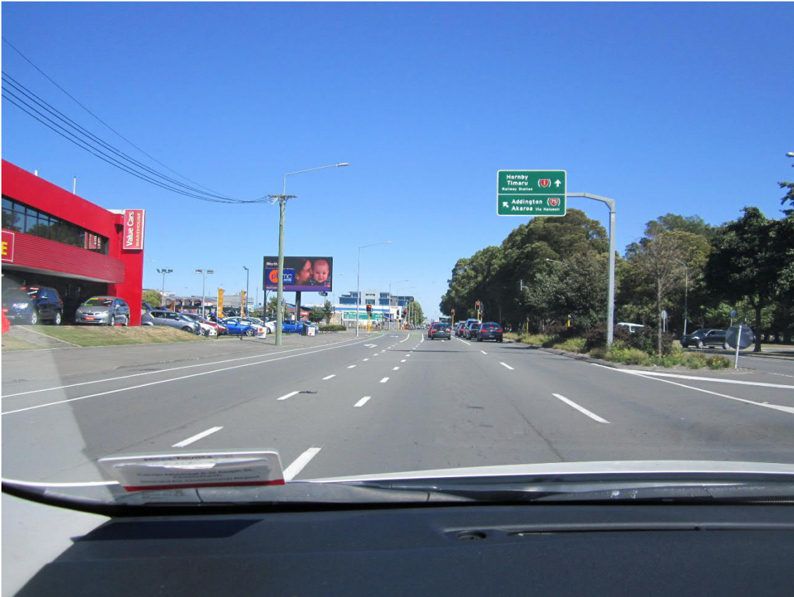
Photograph 10: Moorhouse Avenue – View West (approximately 80m from limit line)
