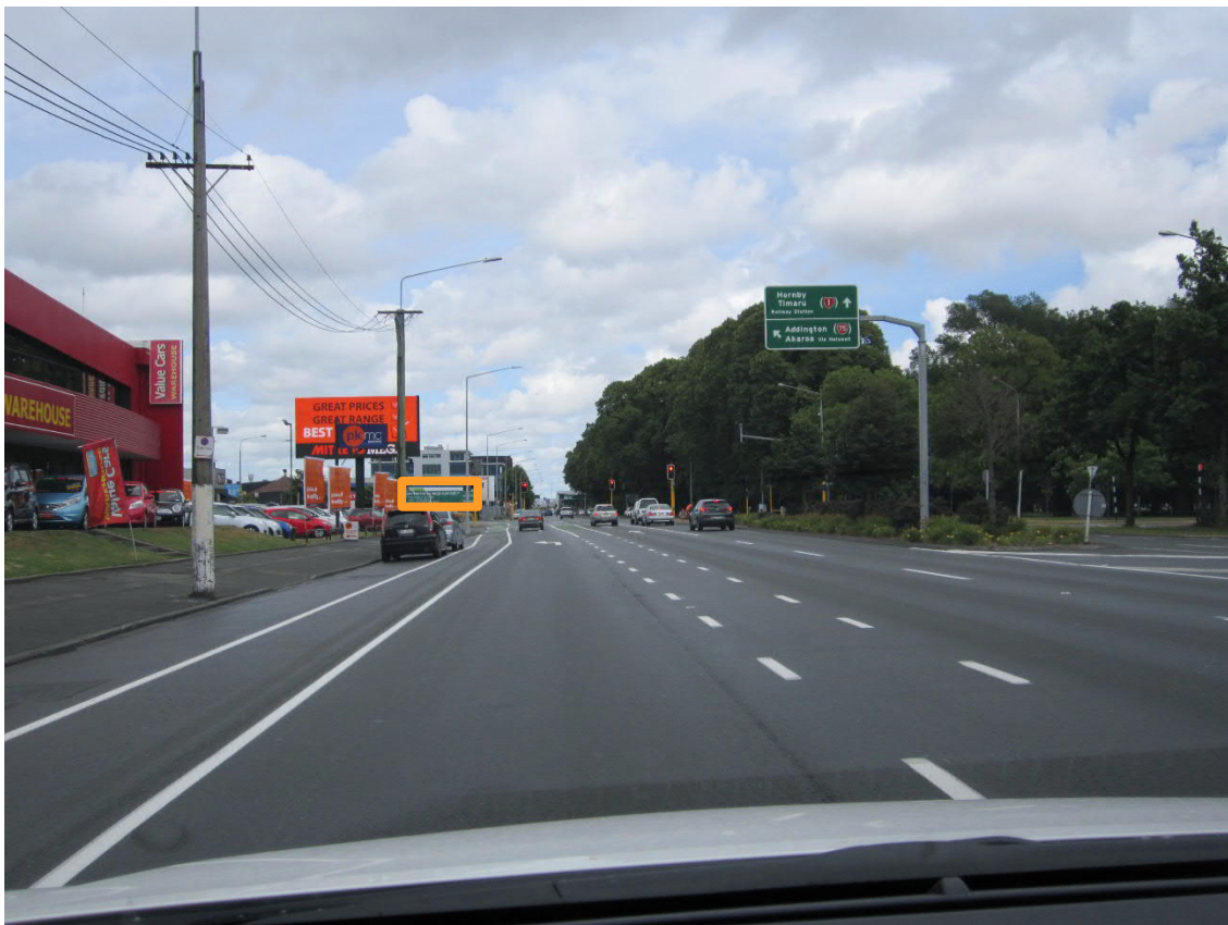
Photograph 3: Moorhouse Avenue View West – Approximately 90m from limit line
