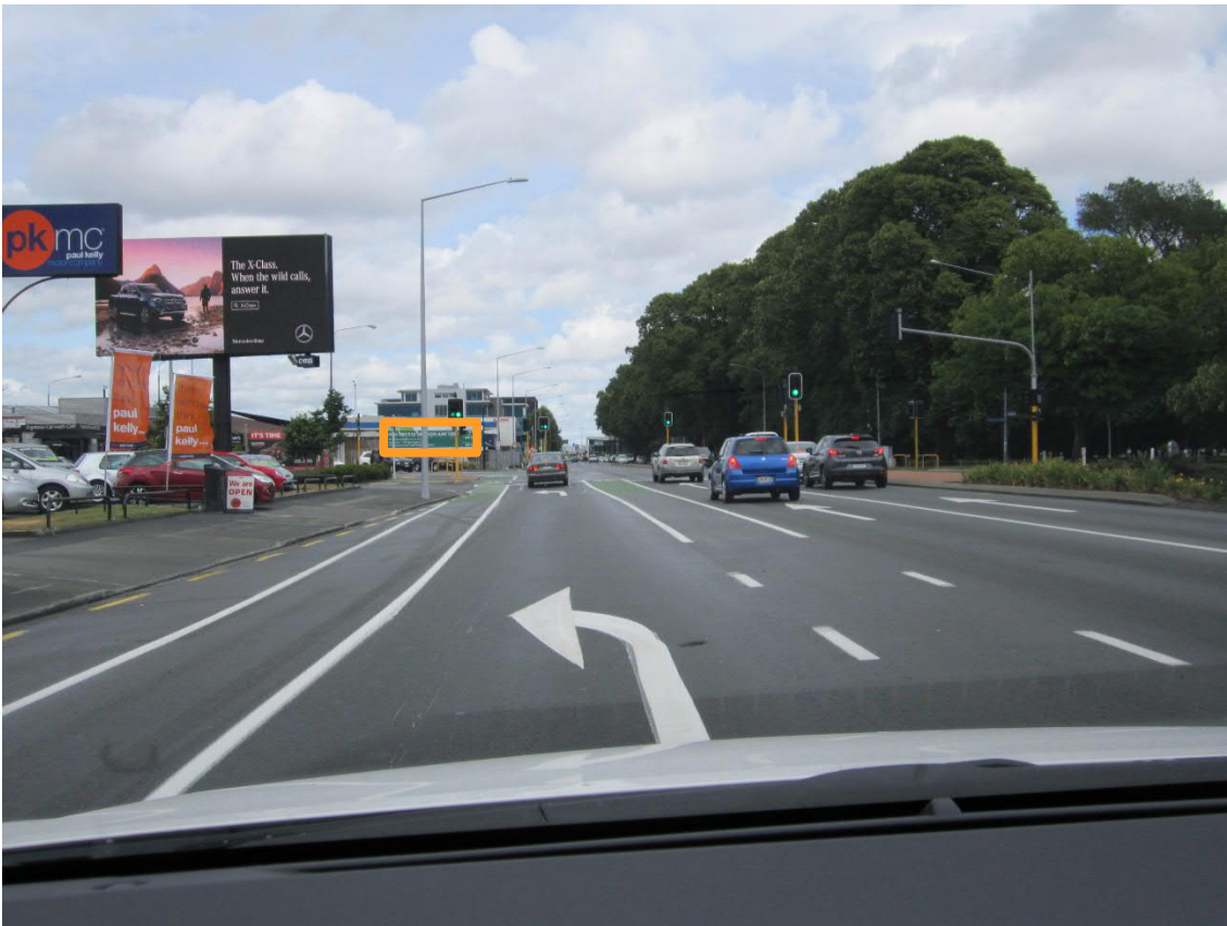
Photograph 5: Moorhouse Avenue View West – Approximately 50m from limit line
