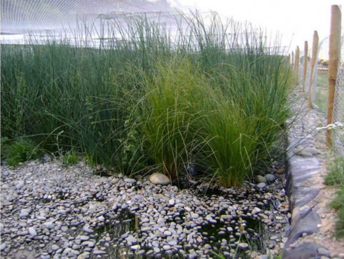
Figure 5-5 Planted Subsurface Flow Wetland at Abel Tasman (Cameron Gibson Wells Ltd)
