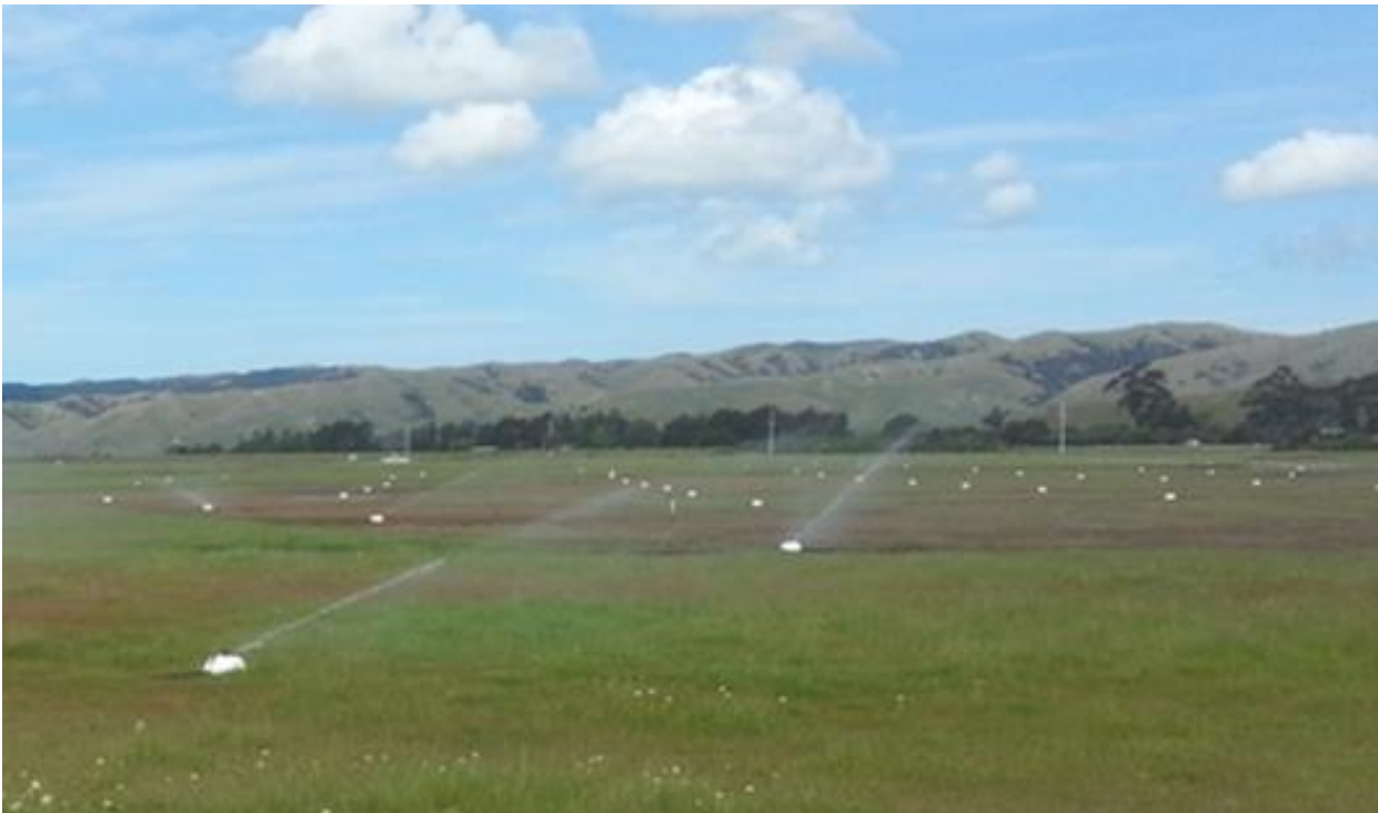
Figure 4-1 K-line spray irrigation of reclaimed water to pasture at Blenheim
