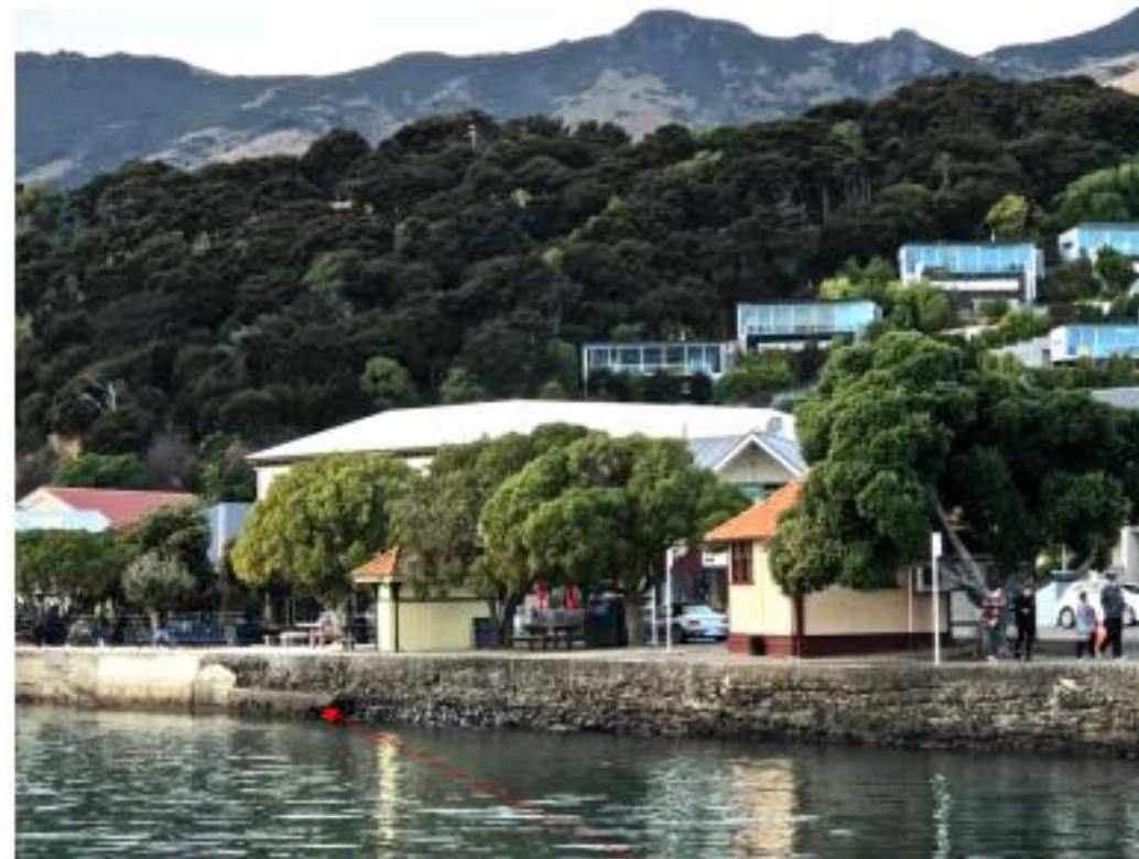
The photo above shows the area where Church Street ends. A possible location for the proposed new wharf, at the base of the 1850s jetty, is visible at the waterline. Fishermen's Rest is located on the left. The structure to the right is the Weighbridge building.
