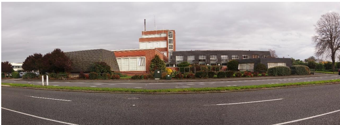
Figure 2: Existing site boundary treatment along Main North Road
