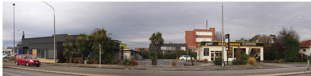
8 View of site from Northcote Road
