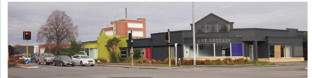
a Commercial Local frontage (site)
