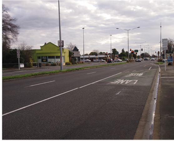
3 View north from eastern side of Main North Rd (opposite to site)
