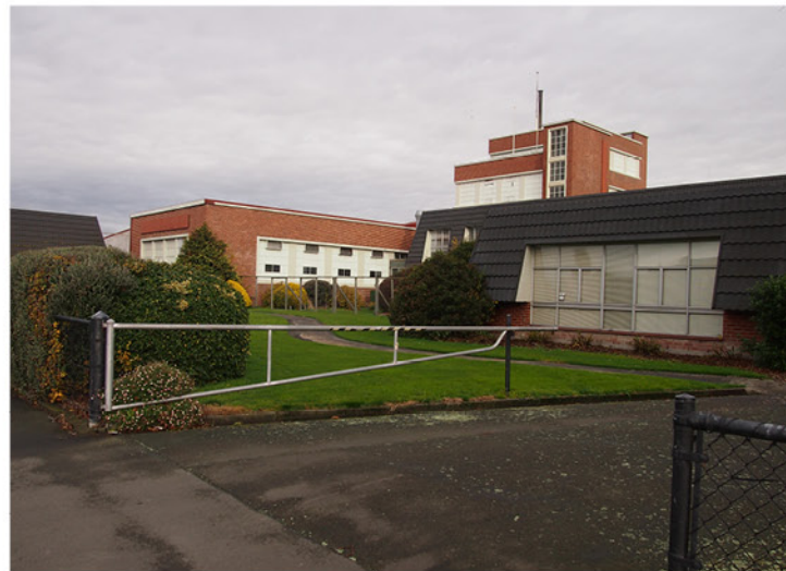
Multiple existing entry /exit points through the site, allowing easy access into the site
