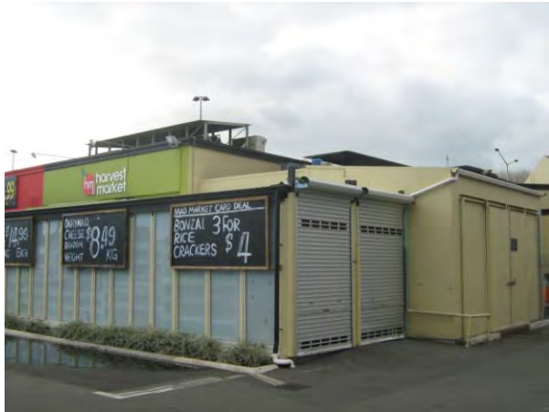
Photo 3: Roof mounted plant
