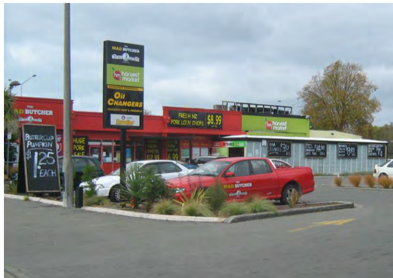
Photo 1 – Shop entrance (western façade)
