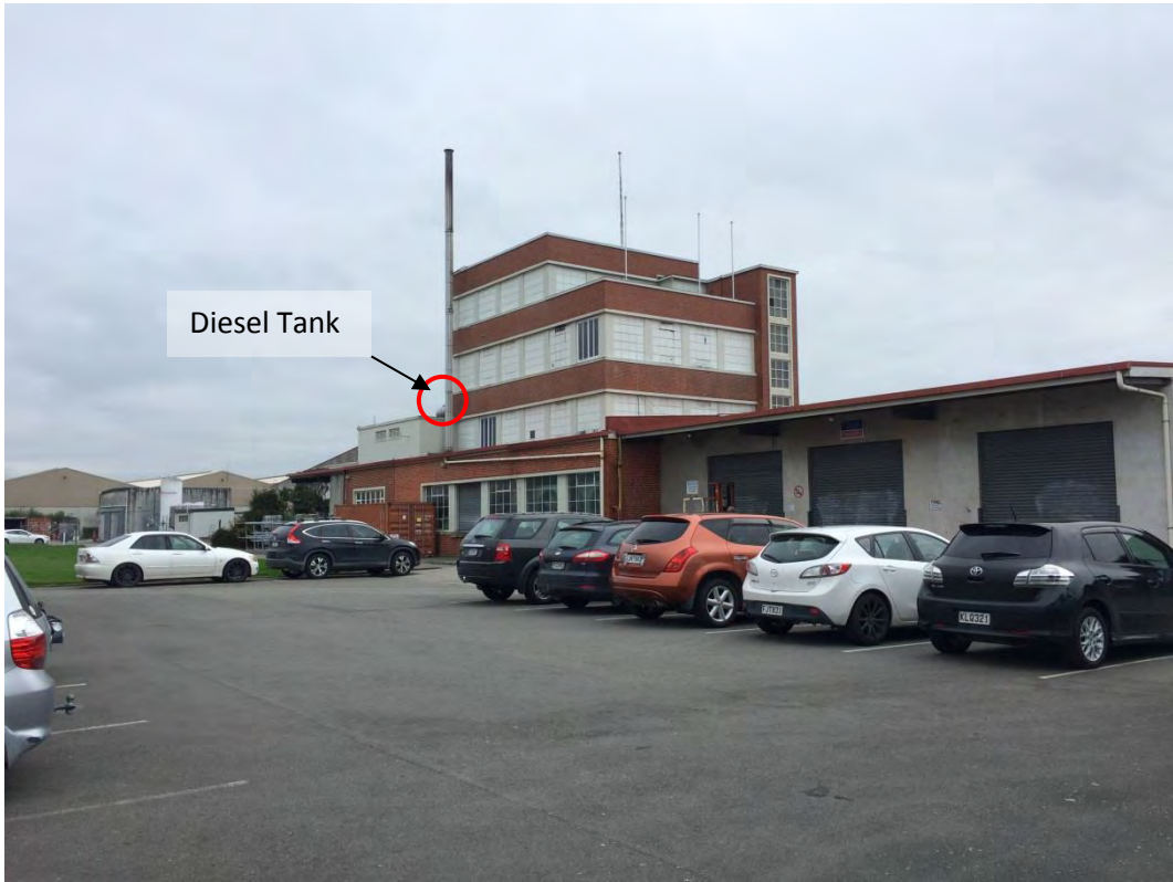
Photograph 15: View looking north-east towards the buildings at 171 Main North Road.
