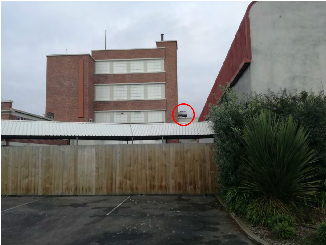
Photograph 6: View looking south over covered walkway towards diesel tank (171 Main North Road).
