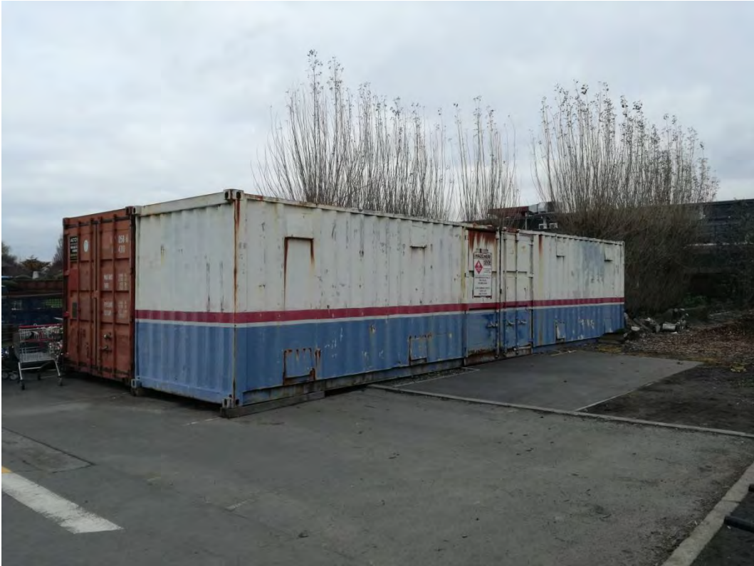
Photograph 11: Container storing flammable liquids in the south-west of the site (171 Main North Road).
