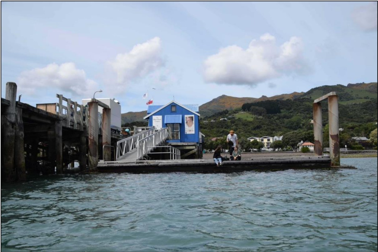
Photo 14 The floating pontoon on the south side of the wharf.
