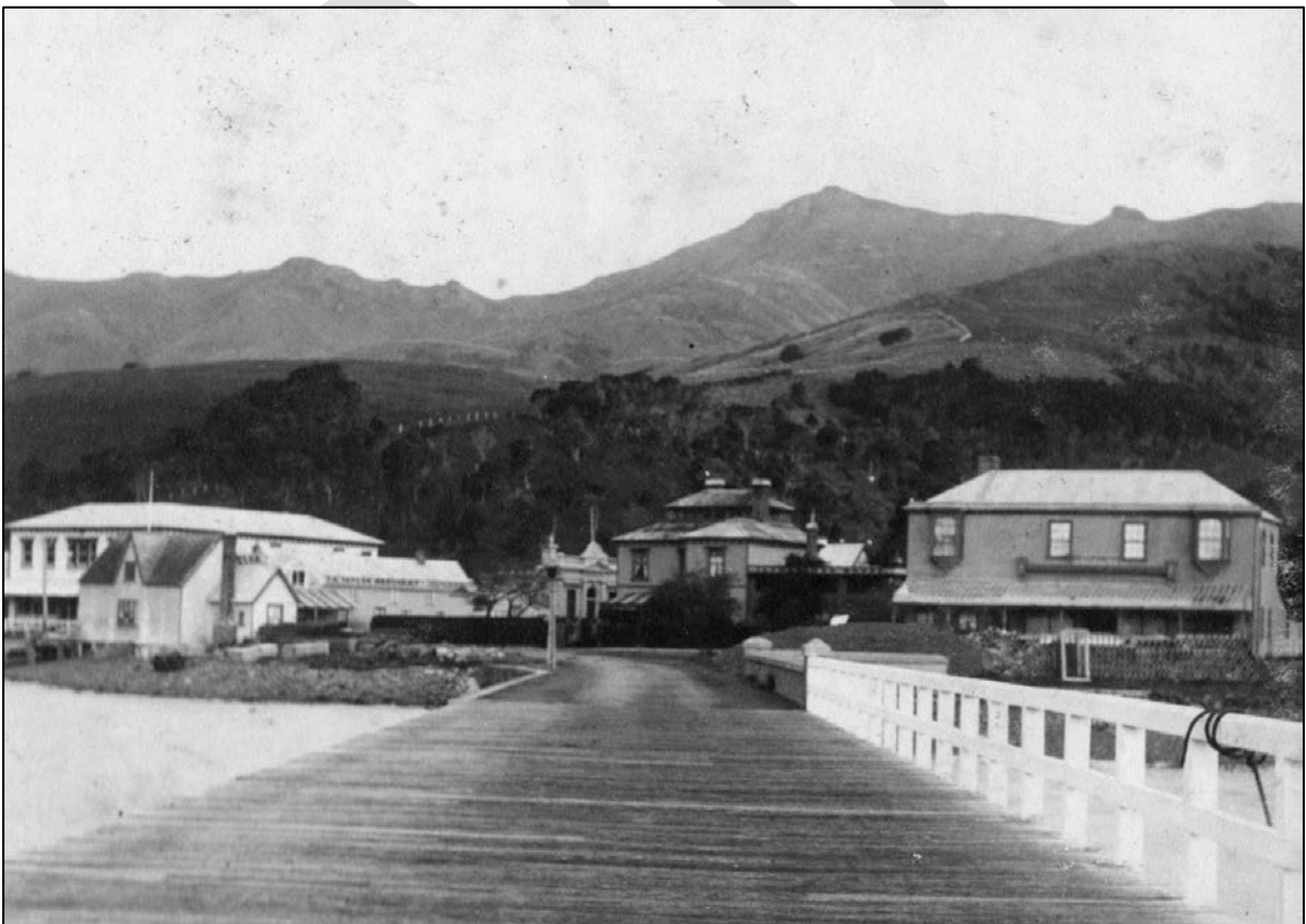
Figure 55. Looking east, 1904 (Kete Christchurch).
