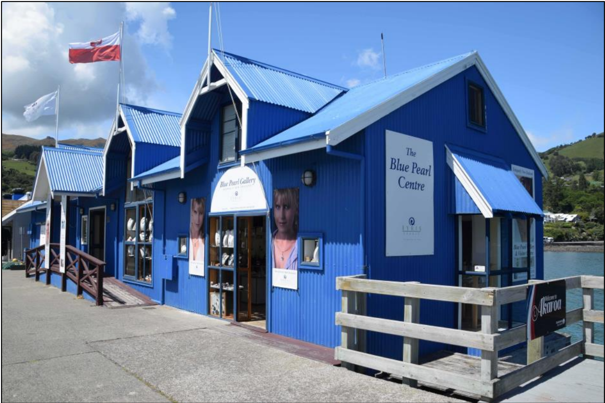
Photo 50 West end of modern sheds.
