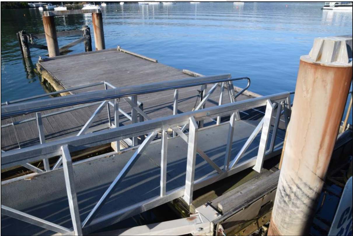
Photo 51 South floating pontoon.
