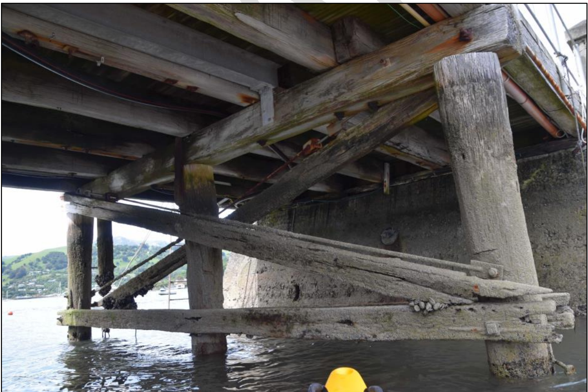
Photo 45 The first bent and the stringer/deck connection to the abutment. This part of the structure contains many original elements, including the pile cap, central pile with wrought iron strap connection to the cap, bracing timbers and horizontal wale between the piles, and timber stringers between the pile cap and modern decking boards.
