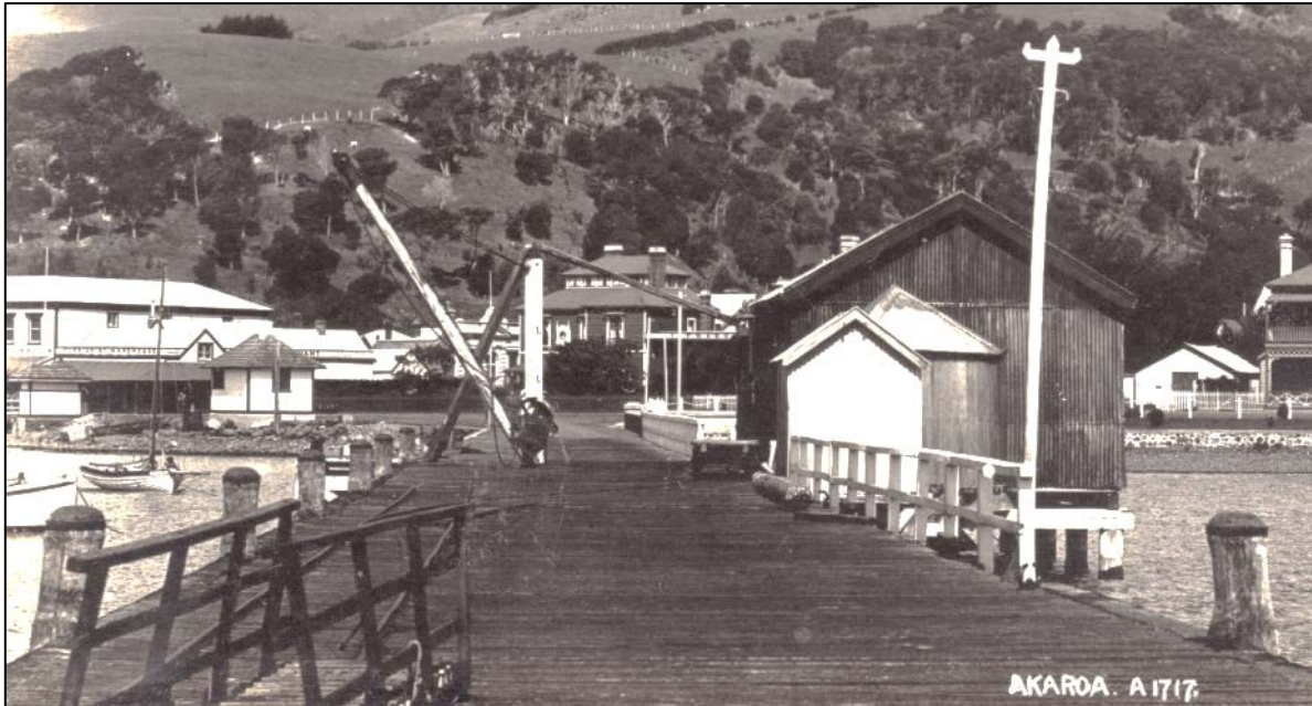
Figure 26. Brightened detail of a 1911 photograph showing the wharf decking (Kete Christchurch).
