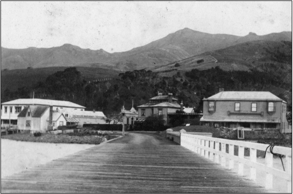
Figure 25. Detail of 1904 photograph showing the wharf decking (Kete Christchurch).
