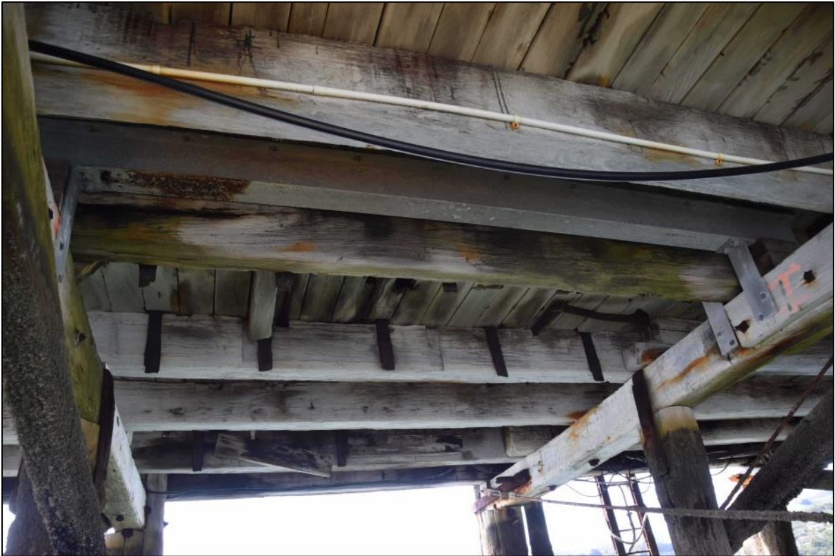
Photo 34 Steel stringer added.
