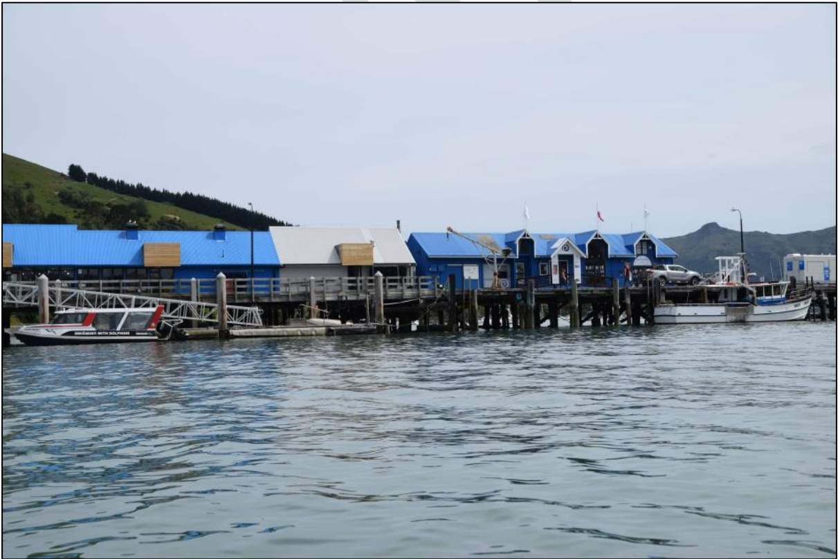
Photo 53 North floating pontoon.
