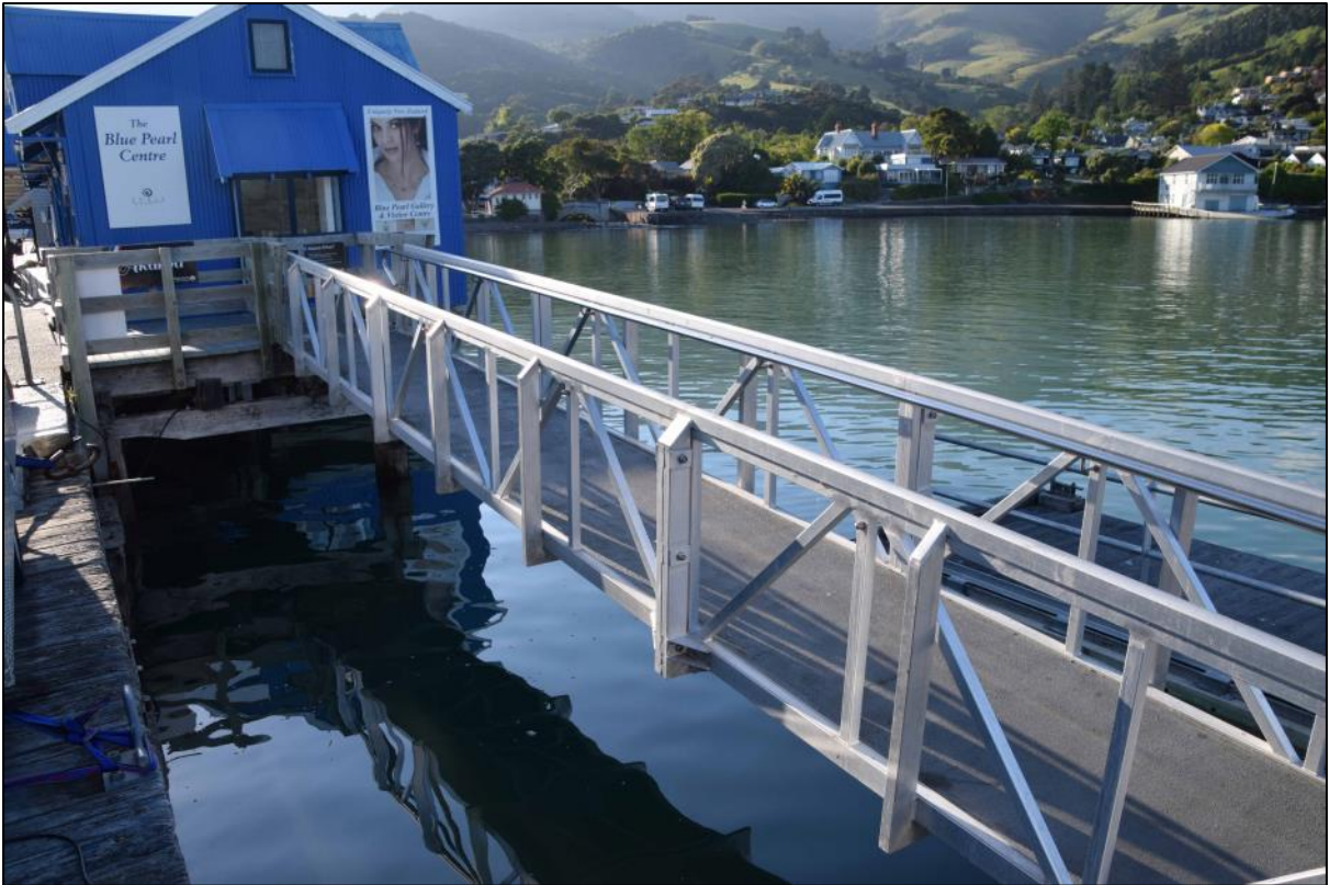
Photo 52 Access walkway to south floating pontoon.
