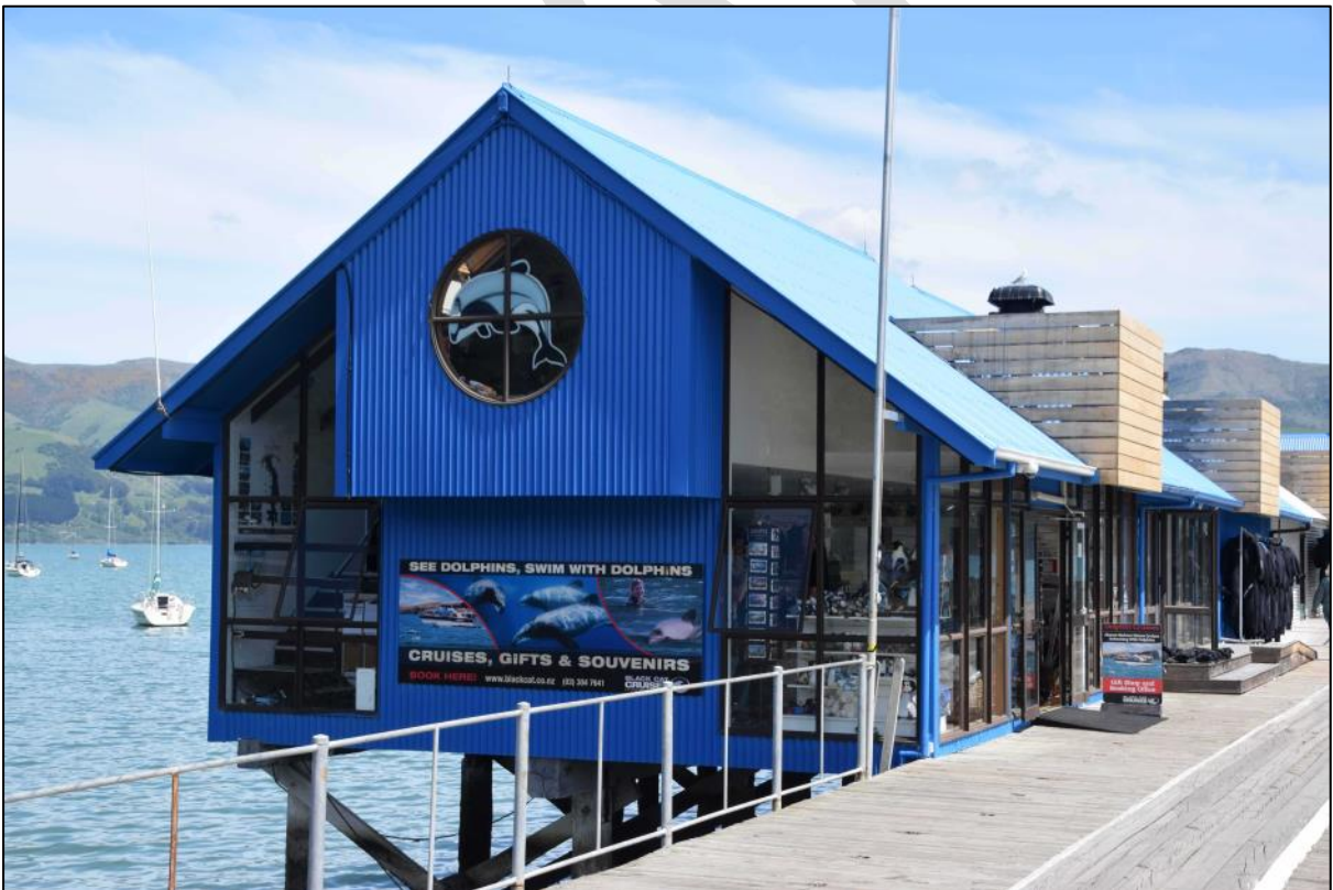
Photo 47 The recent eastern-most extension (extending towards the shore).
