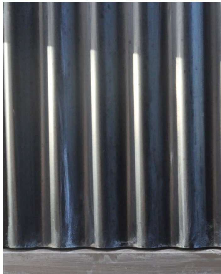
Existing corrugated iron facade along London St Reference profile's curve
