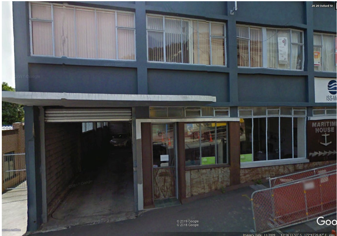
Figure 3: Former Vehicle Access and Roller Door to Car Park Court [Source: Google Earth]
