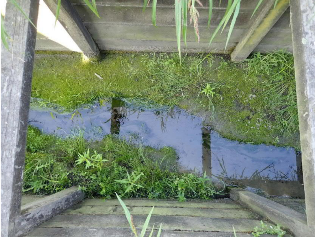
Figure 4: Timber-lined section of Days Drain, showing a sinuous low-flow channel created by sediment and macrophytes.
