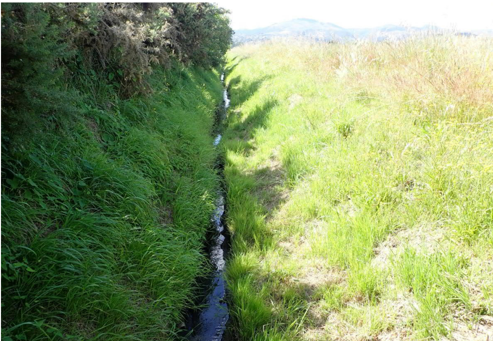
Figure 5: Unlined section of Days Drain, downstream of timber-lined section.
