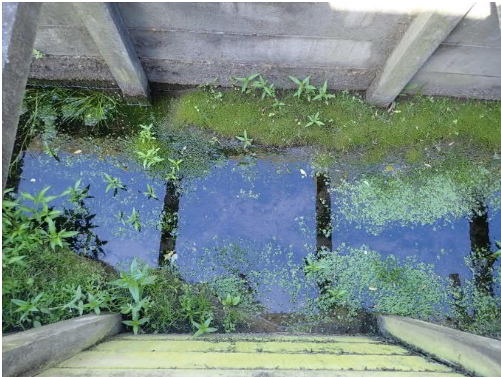
Figure 2: Timber-lined section of Days Drain showing macrophytes and substrate.
