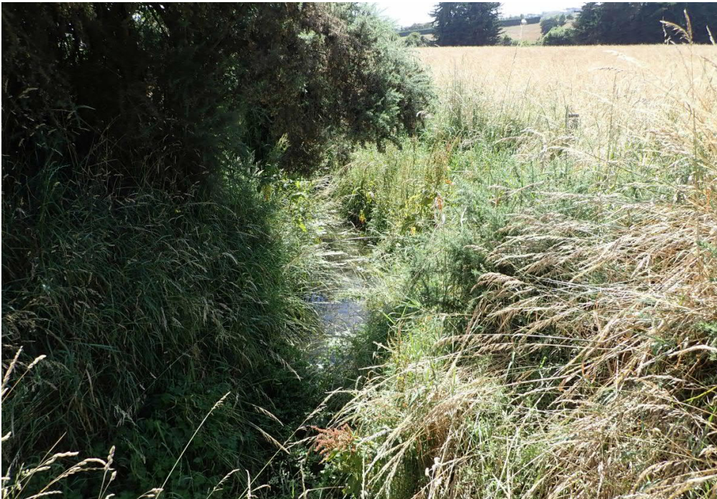
Figure 9: Quarry Road Drain, downstream of Sutherlands Road. This site is to be enhanced by Council in the near future.
