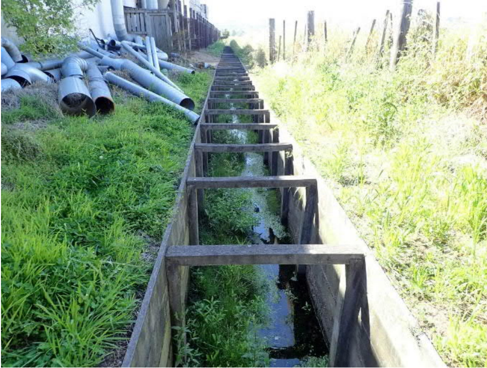
Figure 1: Timber-lined section of Days Drain, looking downstream from Halswell Road
