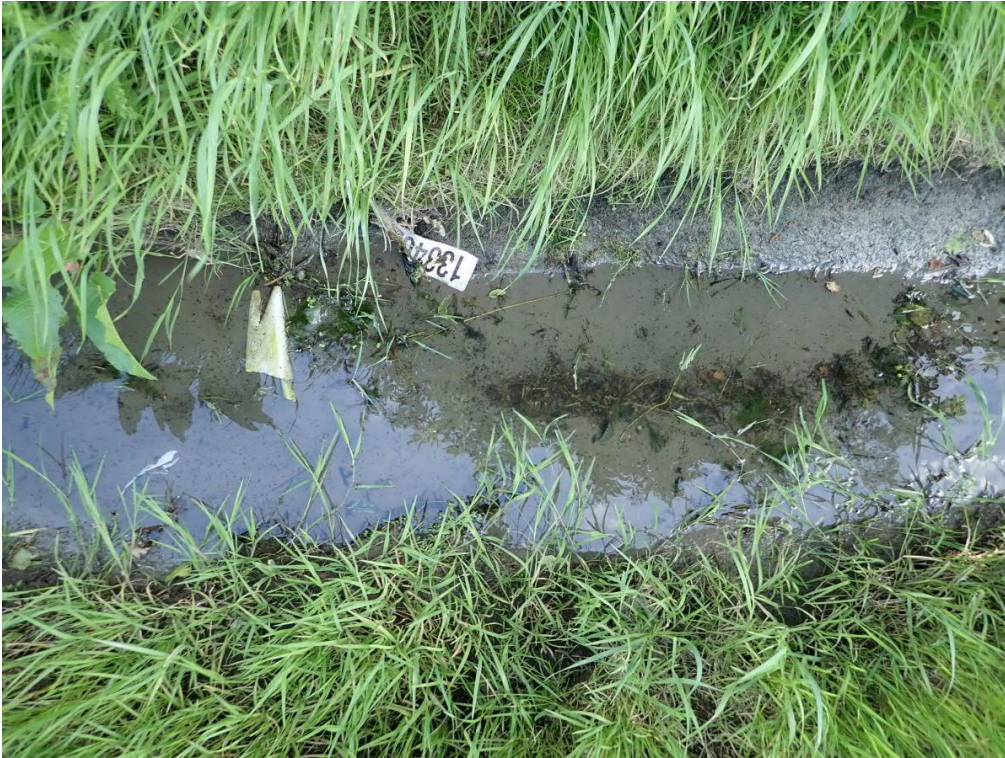
Figure 6: Unlined section of Days Drain showing fine substrate and litter from the timber yard.
