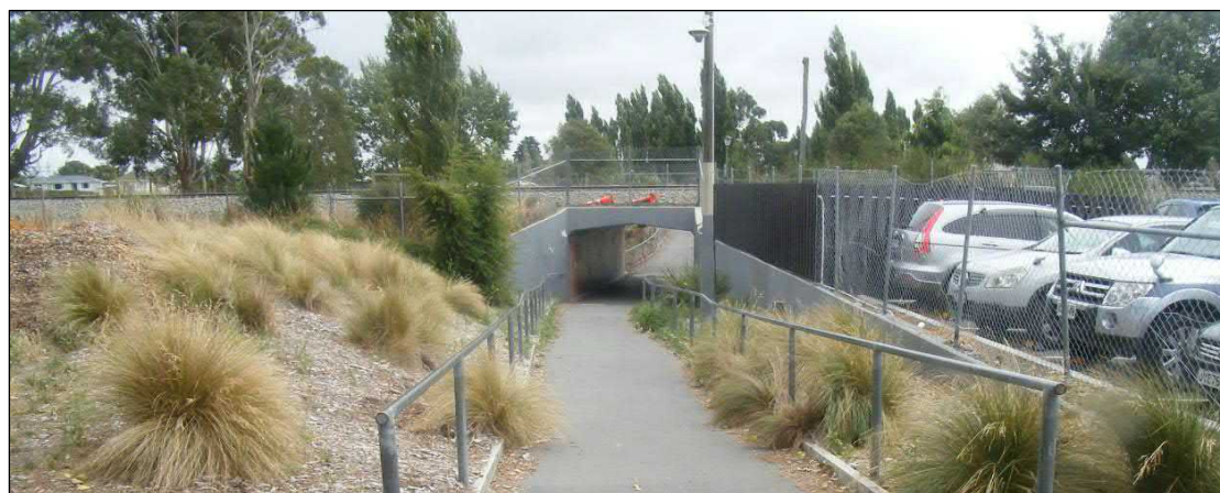
Railway underpass viewed from the southern approach.
