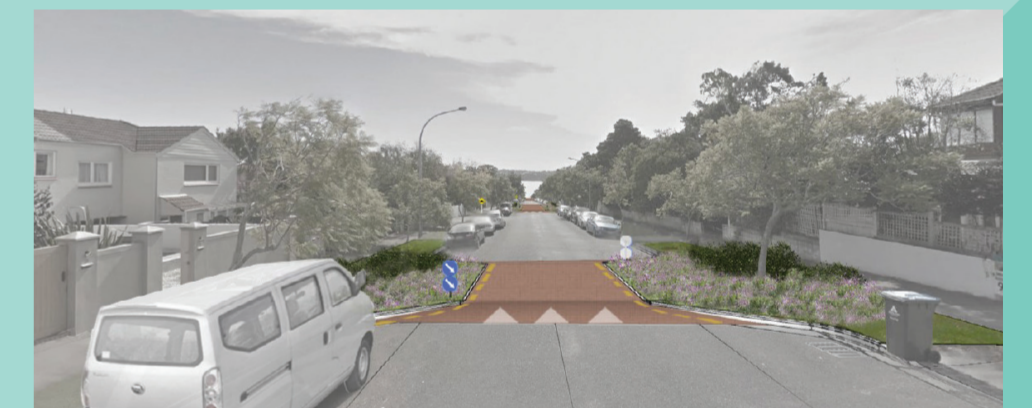
Mid block raised platform with road narrowing
