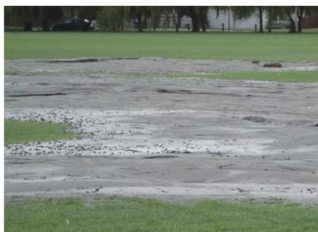
Liquefaction damage to QEII Park.
