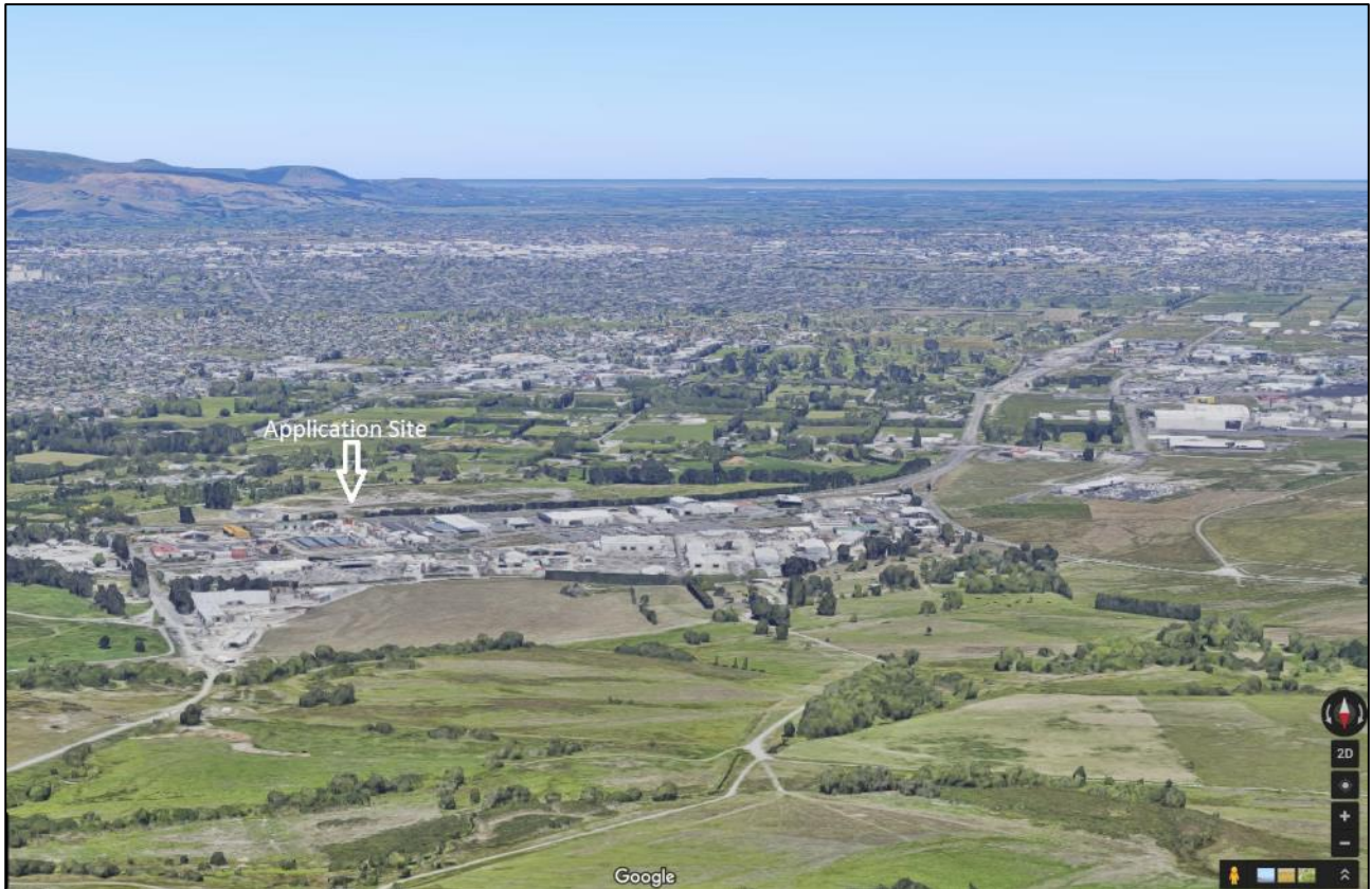
Figure 2-3 Oblique aerial [source: Google]
