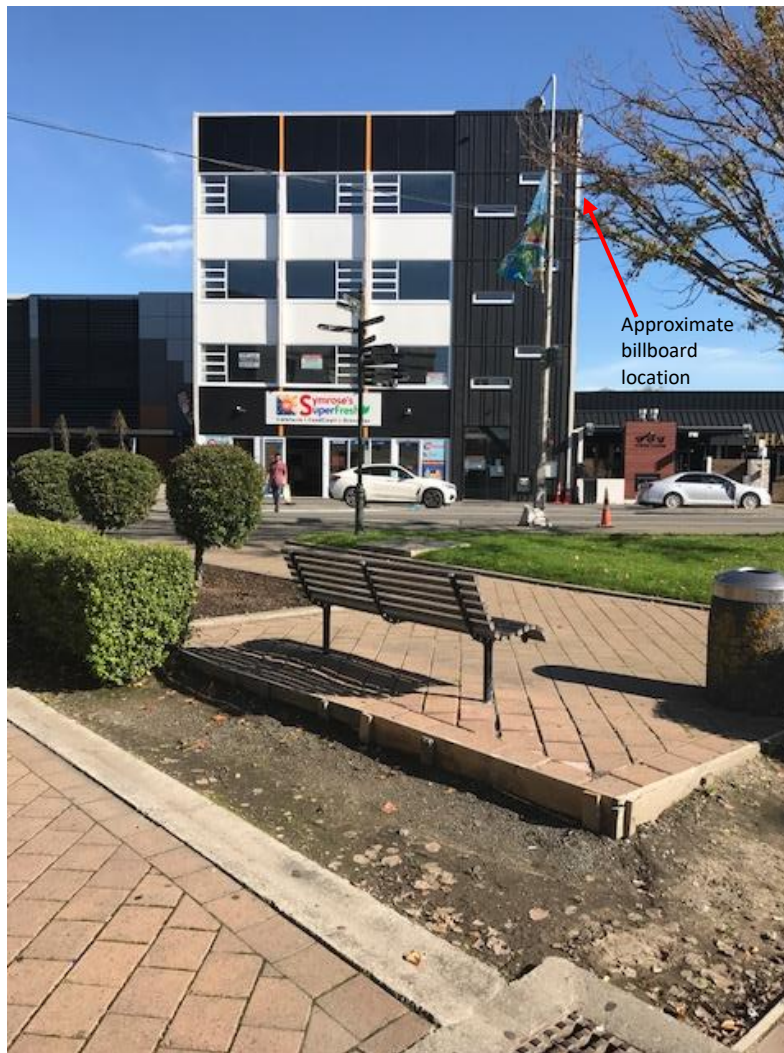
Image of the building frontage of 65-67 Victoria street facing south west as viewed from the Central City Community Park opposite the site.
