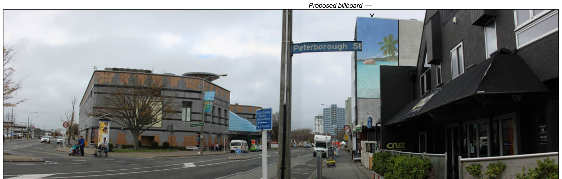
Photograph 4 View from west side Victoria Street at Peterborough Street intersection
