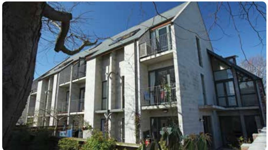
St Mary's Apartments, Christchurch
