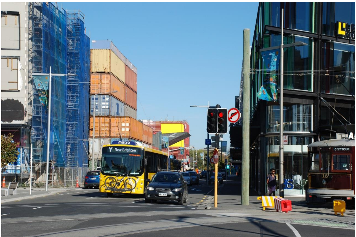
Location 4; Looking west from Lichfield Street roughly 265 meters away from the billboard. The billboard shows roughly the same size so messages can be just as easily read. The billboard is obscured by the roof of the bus interchange. This photo is taken exactly from the corner of the East frame as such a possible view for residential developments.
