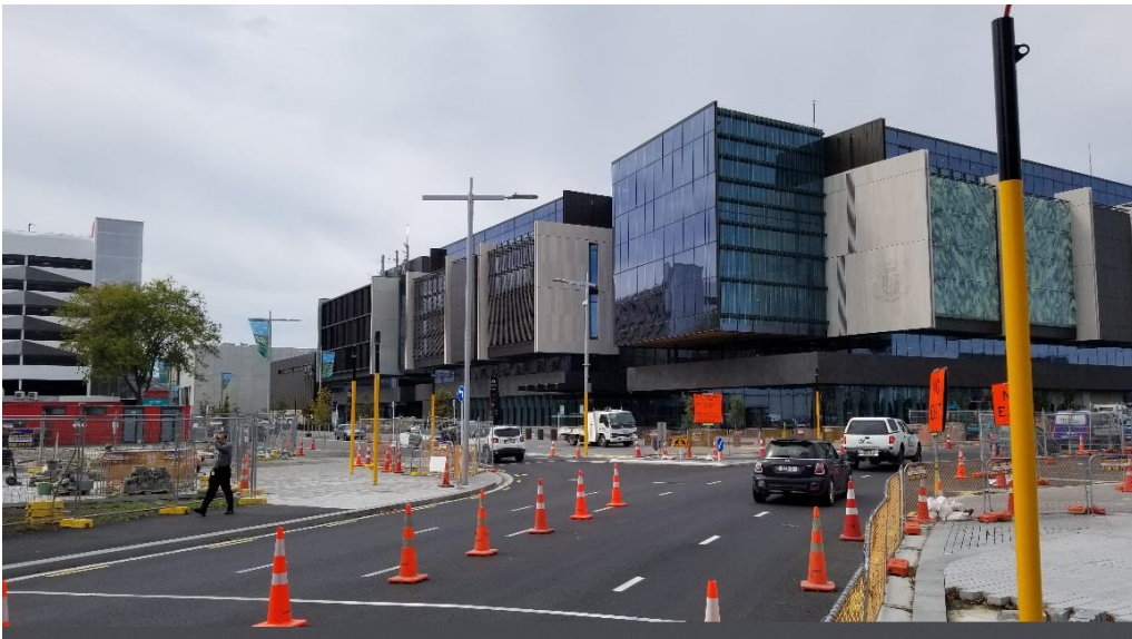
Justice and Emergency Services Precinct
