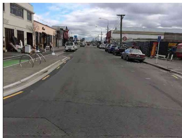
Photo 9: Same location as Photo 8, note no centreline or RRPMs for extended length west of Colombo Street
