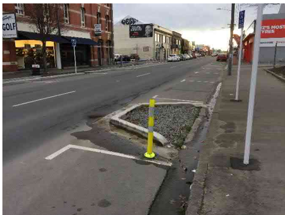
Photo 1: Example of new tree pit build-out and constrained road environment.
