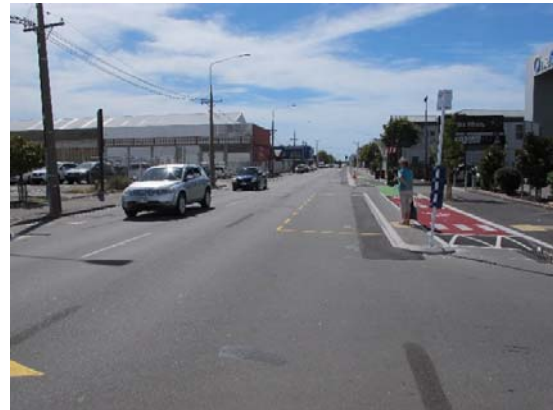
Photo 16: Example of conflicting markings (including ‘ghost’ markings from old road layout)
