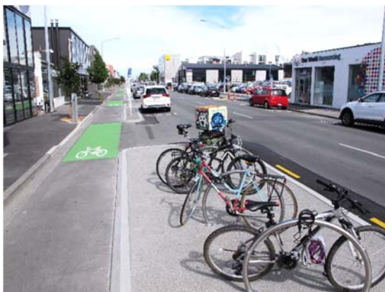
Photo 5: Example of left turn in protection offered by kerb build out. Note utilisation of this space for cycle parking and street art (installed by local business)
