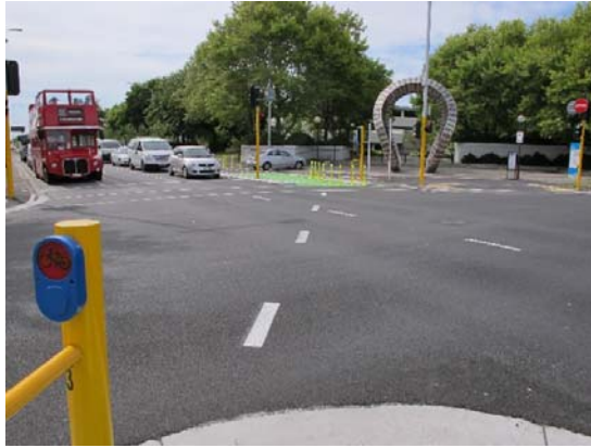
Photo 31: Miss-aligned pavement markings for cyclists. Note – this could be confused for conventional lane leader lines for drivers.
