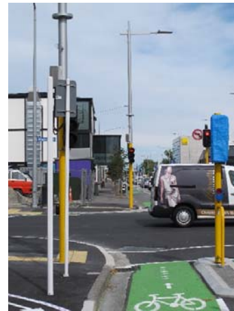
Photo 30: Sign masks primary traffic signal for cyclists.
