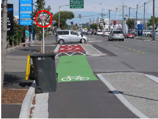
Photo 17: Cyclists view on approach to bus stop. Note Give Way sign (circled) is lost in street furniture, and rubbish bin placed in the cycle facility.
