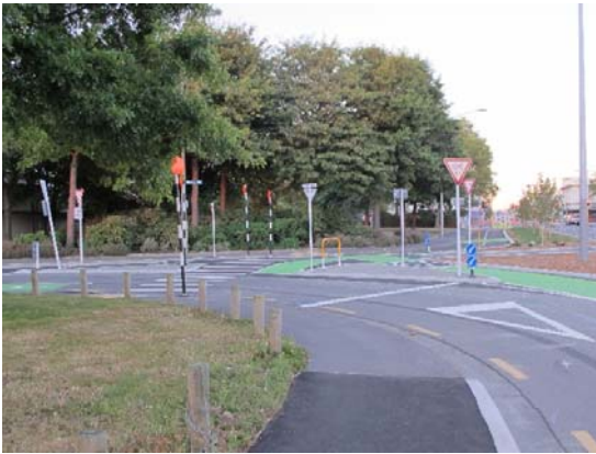
Photo 25: Confusing markings and signs – Ferry Road / St Asaph Street intersection
