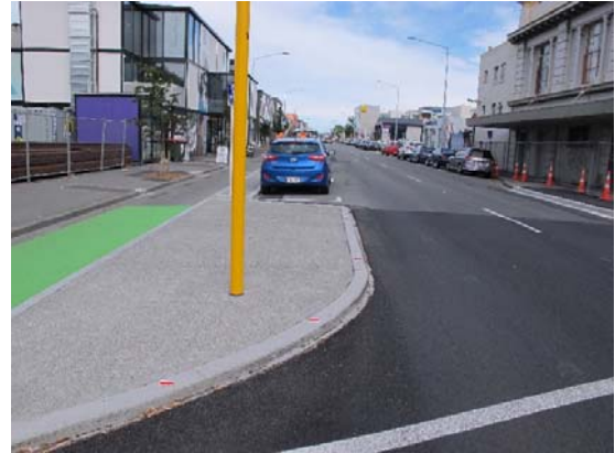
Photo 2: Example of kerb build outs to achieve protection for parked vehicles, and correct placement of traffic signals.
