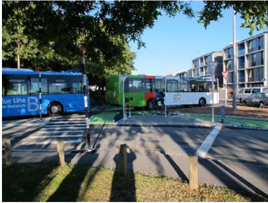
Photo 27: Current design requires an exiting bus to straddle the new facility. Cyclists cannot see merging cyclists on opposite side of the bus
