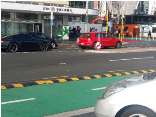
Photo 7: Example of low profile raised separator at access – Bi-directional facility, Quay Street, Auckland
