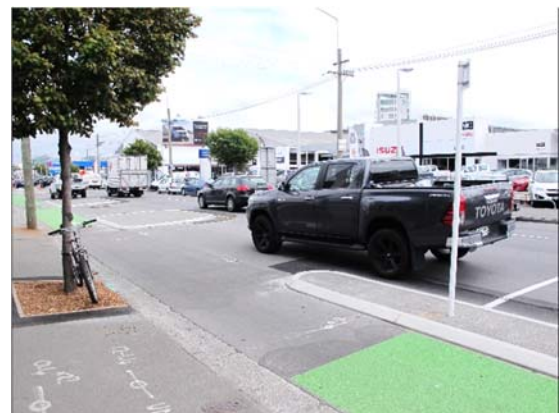
Photo 6: Example of unprotected left turn in. Driver is positioned such that they cannot see back down cycle facility.
