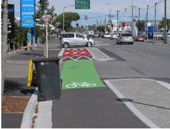
Photo 19: Example of rubbish bins placed in the cycle facility.
