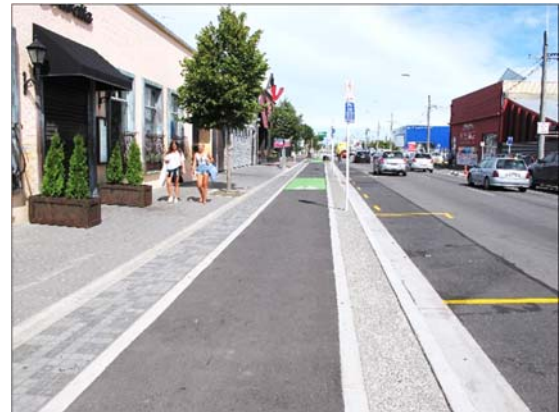
Photo 12: Example of cycle facility raised to footpath level, with concrete edge treatments to define path.
