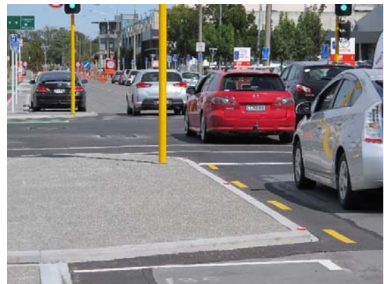
Photo 14: Example of Red RRPM installed on kerb top.
