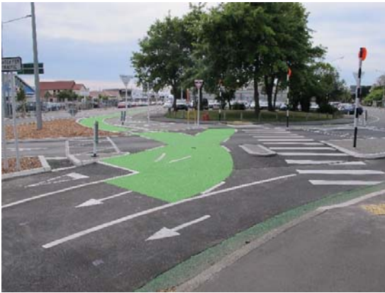
Photo 23: Confusing markings and signs – Ferry Road / St Asaph Street intersection
