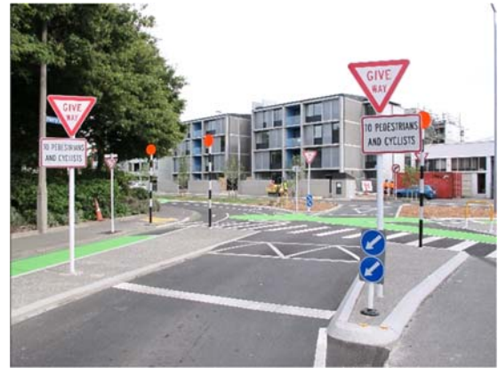
Photo 24: Confusing markings and signs – Ferry Road / St Asaph Street intersection
