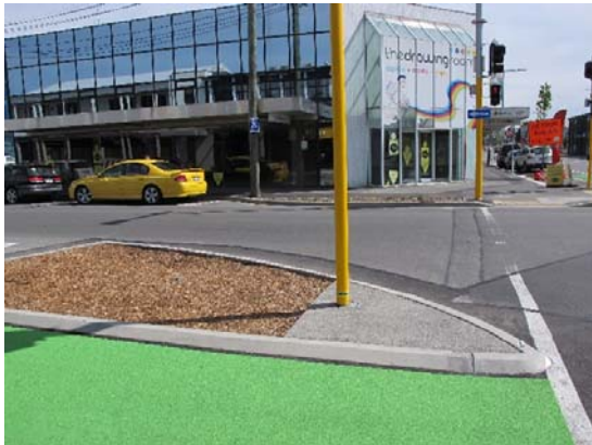
Photo 15: Example of old and ineffective pavement markings – Manchester St / St Asaph St.
