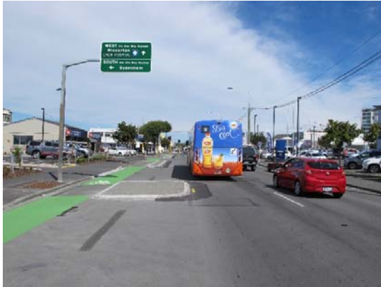
Photo 1: Example of new constrained road environment. Note low conspicuity of kerb.
