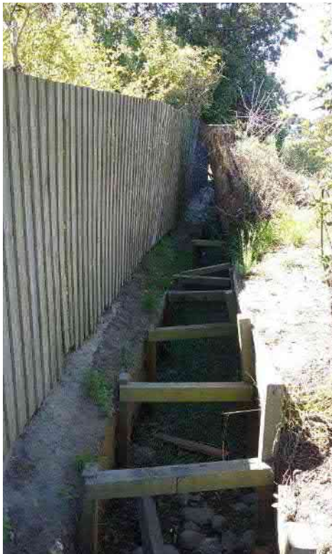
Image 7: Knights Drain (upstream timber-lined reach)
