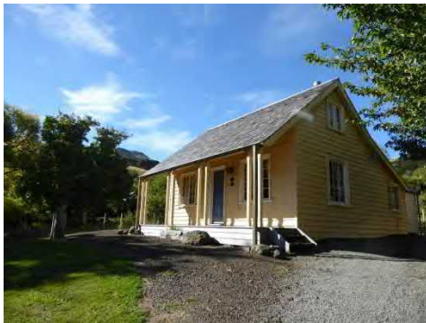
Figure 2 Flooding at Pavitt cottage April 2017
