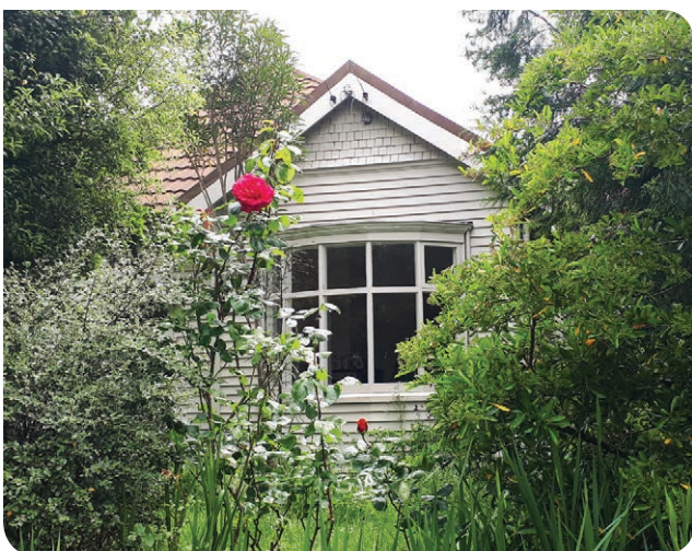
Detail of a gable end of an early 20th century villa
