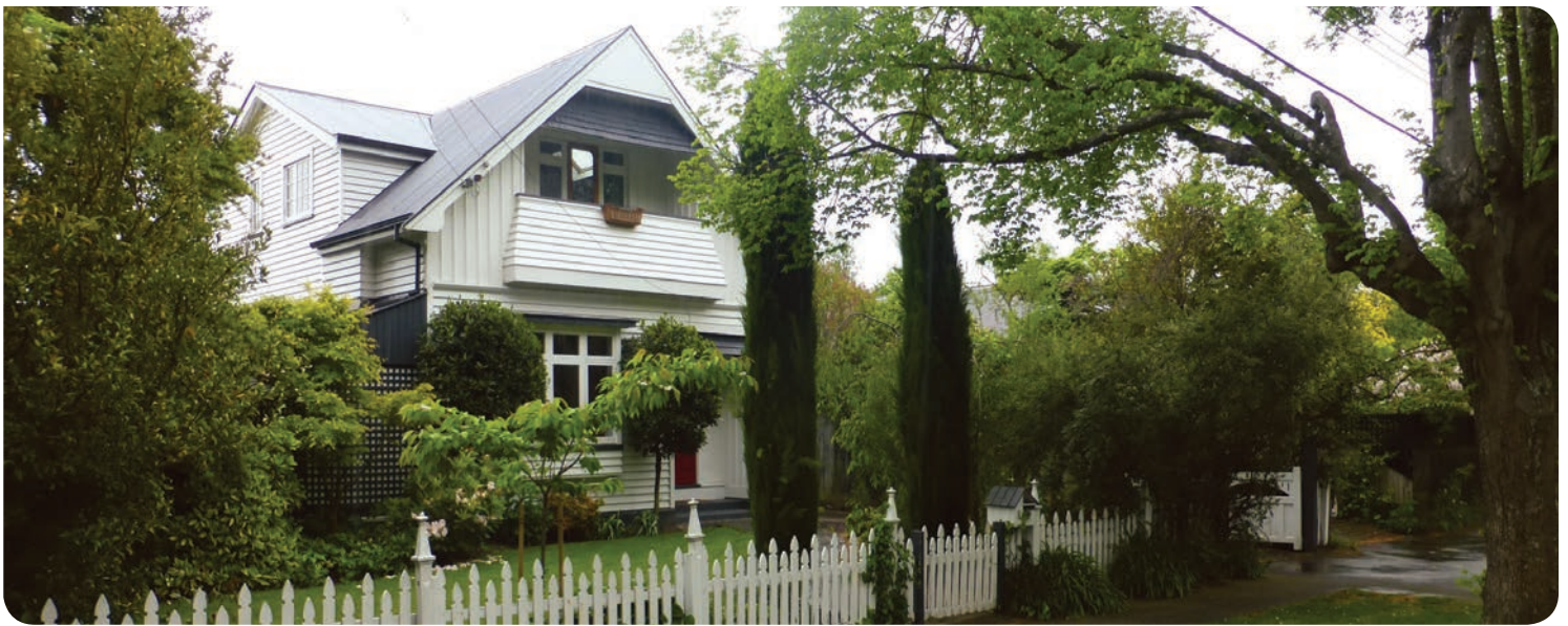
Example of a English Domestic Revival house in Tainui
